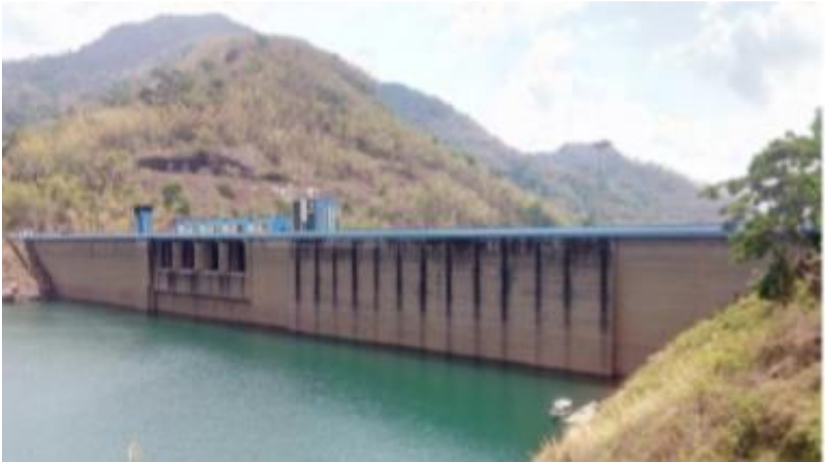
Figure 1.1: View of dam from upstream
