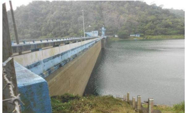
Upstream face of the Dam
