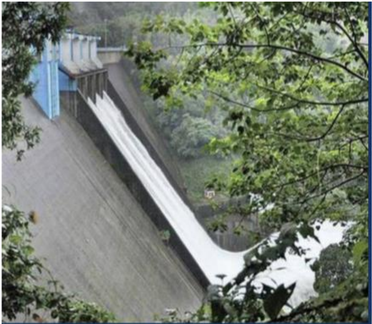
Figure 1.2: View of dam
