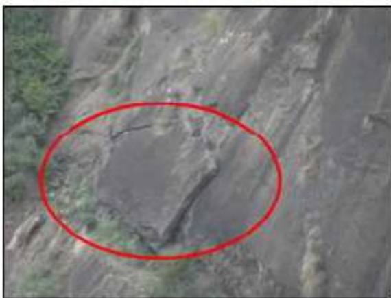
Rockfall from abutment rock of Idukki dam
