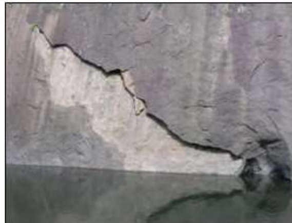
Rockfall from abutment rock of Idukki dam
