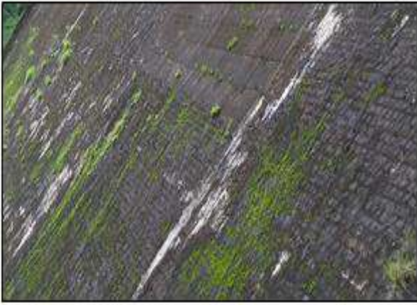
Leaching at Downstream face of Kulamavu Dam
