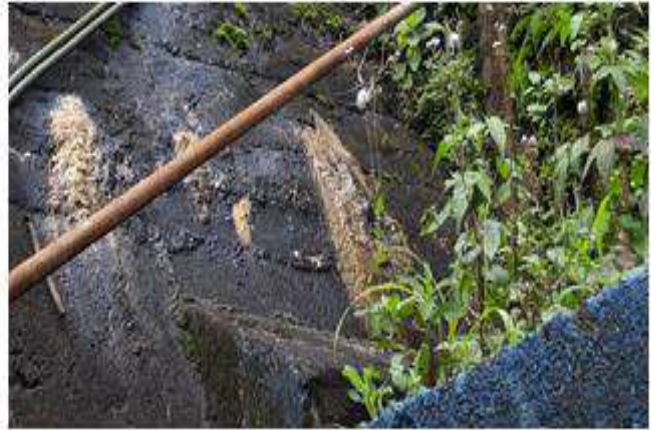
Leaching at Downstream face of Kulamavu Dam
