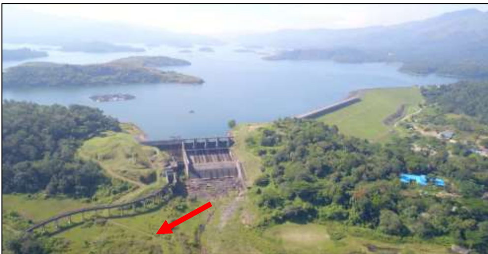
Proposed site for new access road to the right bank of spillway dam
