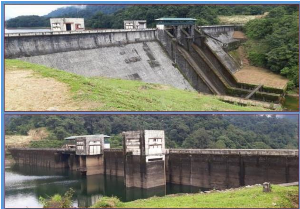
Figure 1.2: Downstream and upstream view of the dam
