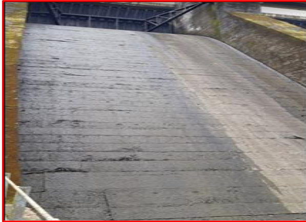
Rectification of pitting in spillway glacis
