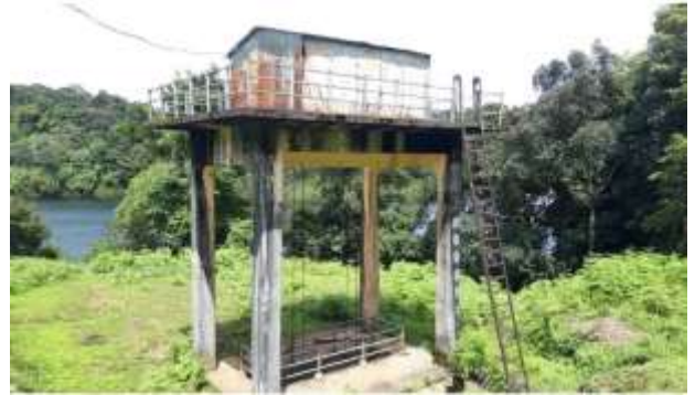
Control shaft of IC Tunnel
