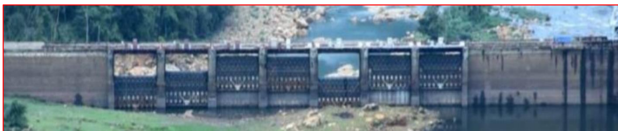
View of Dam from Upstream
