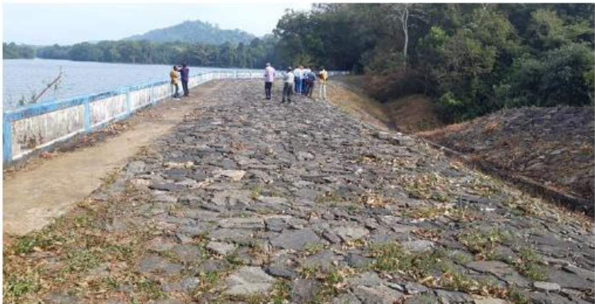
Figure 1.3: Selected Photographs of Improvement/Intervention area
