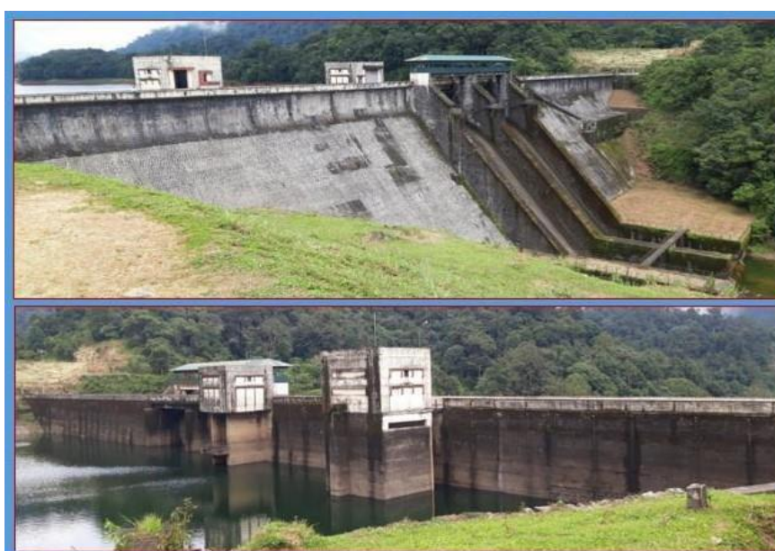
Figure 1.2: Downstream and upstream view of the dam
