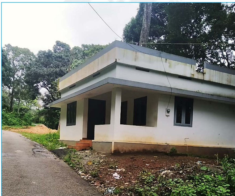
Security cabin at dam top
