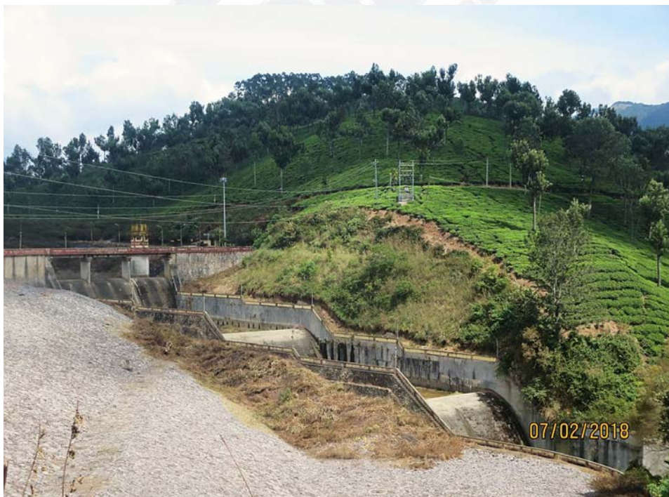
Fig 2.2b Spillway of Anayirankal dam
