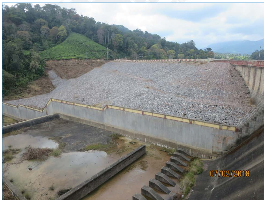
Fig 1.5b Downstream Elevation of Anayirankal Dam
