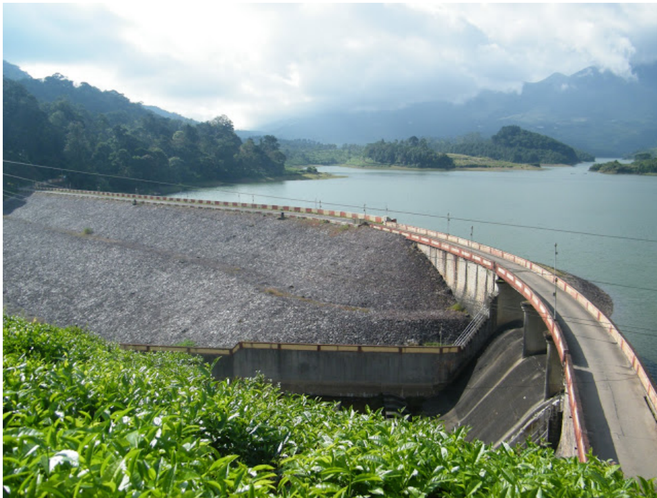
Fig 2.2a Spillway of Anayirankal dam
