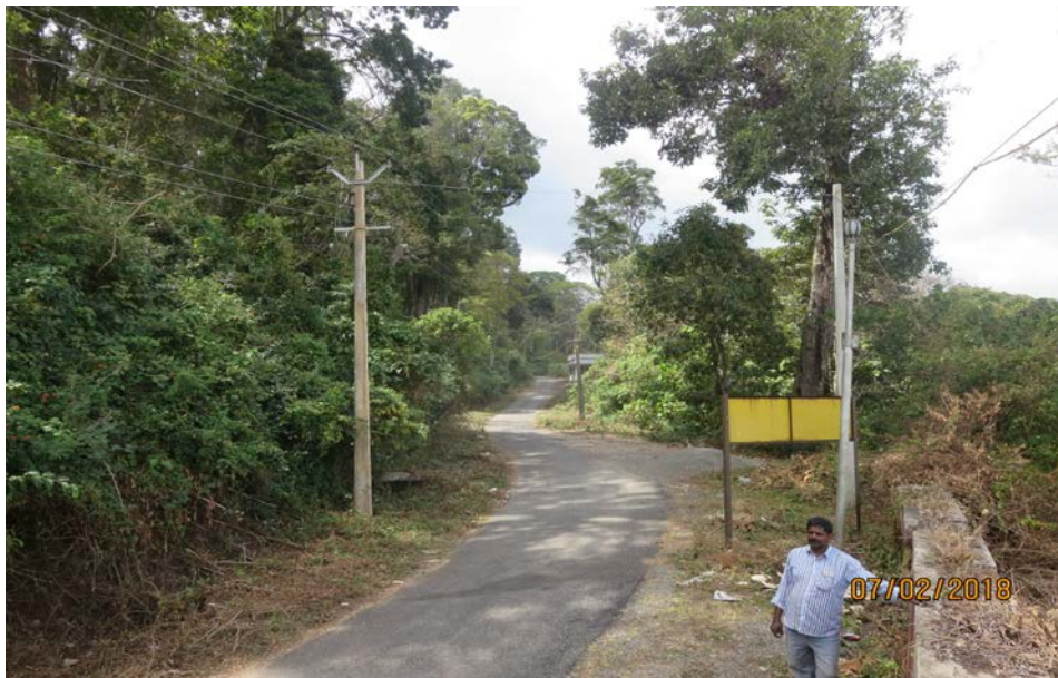
Approach road to dam top
