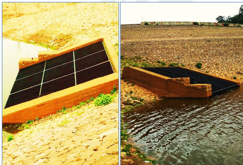
Fig 2.7 Anayirankal dam Sloping Trash rack
