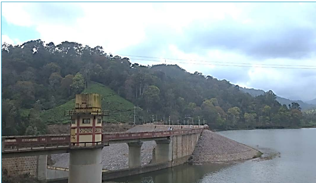
Upstream slope protection
