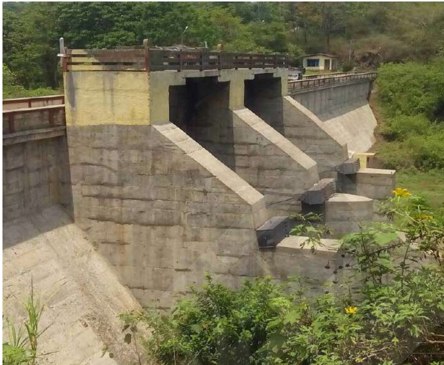
Fig 2.2a Downstream Elevation of Erattayar Dam
