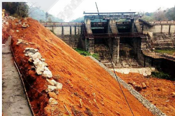
Protective wall at the right bank of d/s spillway
