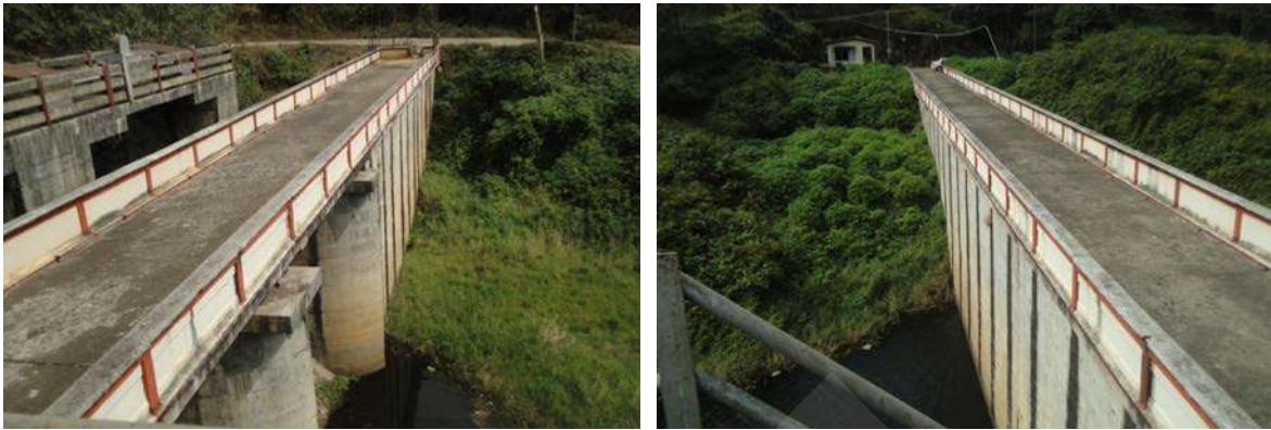
Fig 2.2c Upstream Right bank and Left bank
