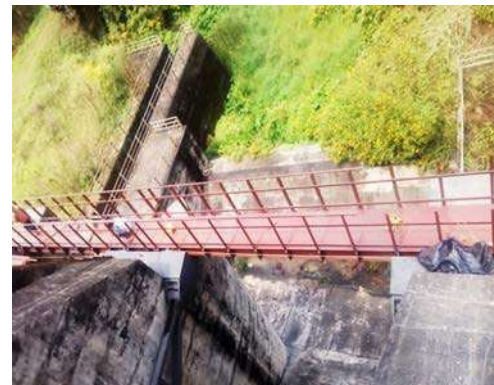
Fig 2.4b Downstream side river outlet
