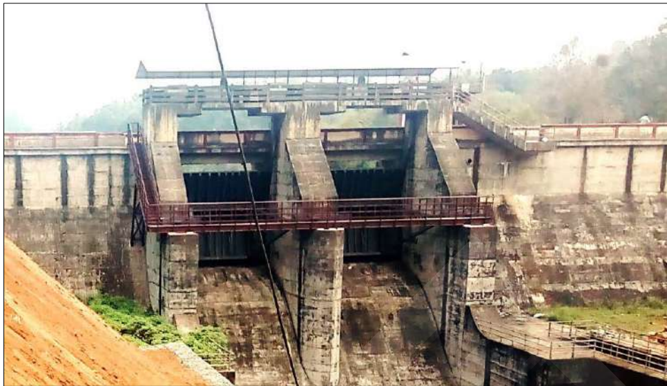
Fig 2.8b View of Spillway from downstream showing Spillway Gates
