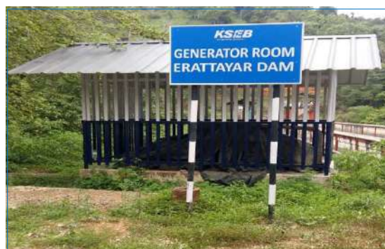
Erattayar Dam Generator room
