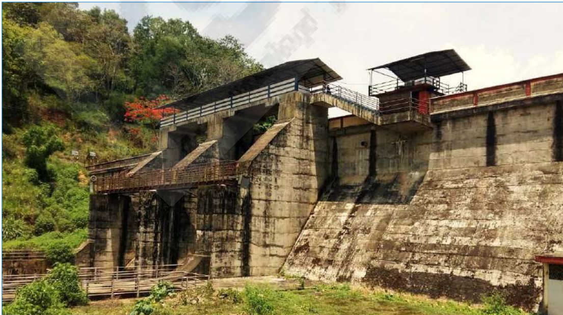
Fig 2.8a View of Spillway from downstream with Hoist Bridges
