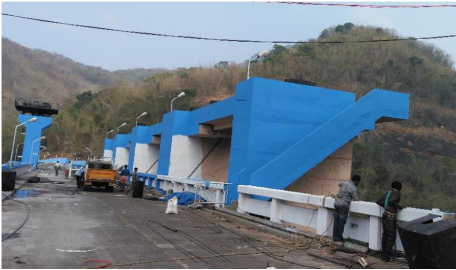
Fig 2.3 Radial Gates Hoist Bridge
