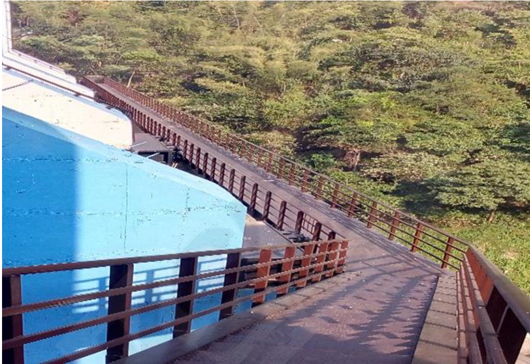
Fig 6.2 Catwalk connecting Radial gate trunnions
