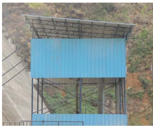
AFTER ROOFING WORK TO HOLLOW JET VALVE
