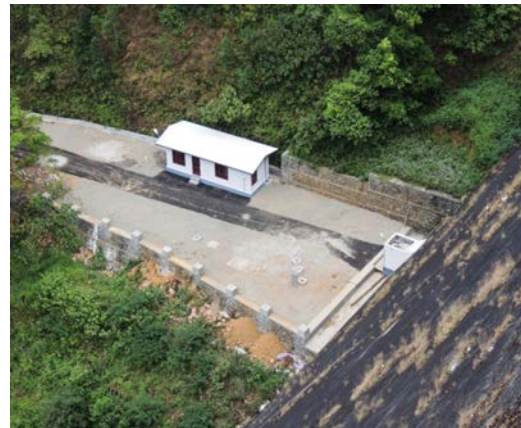
SECURITY GUARD ROOM D/S OF KAKKI DAM AFTER CONSTRUCTION
