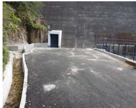
KAKKI DAM ADIT - II AFTER DRIP WORKS
