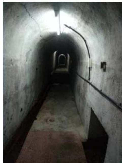
DRIP – Reaming of drain holes
