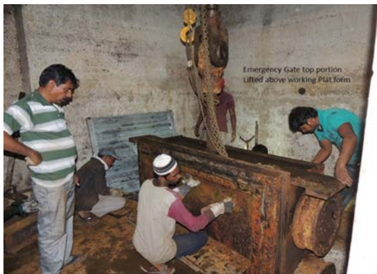
EMERGENCY GATE LIFTED FOR REPAIR WORK
