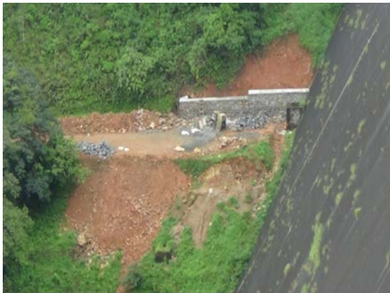
SECURITY GUARD ROOM D/S OF KAKKI DAM BEFORE CONSTRUCTION
