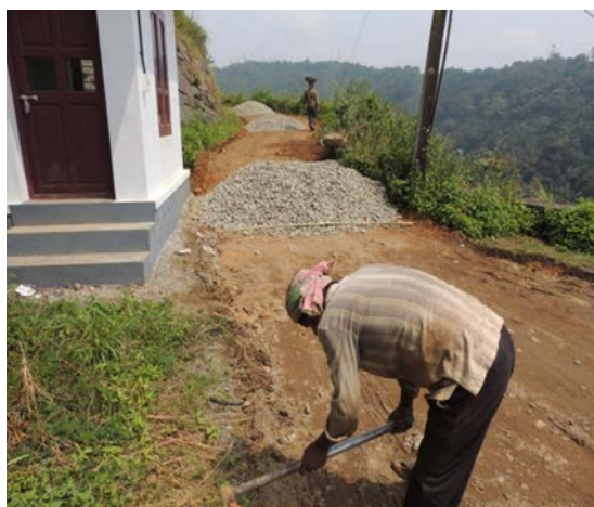
KAKKI DAM L/B ADIT-1 ROAD ENTRANCE BEFORE DRIP WORK
