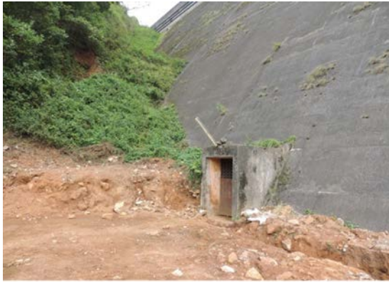
KAKKI DAM - D/S RETAINING WALL BEFORE CONSTRUCTION
