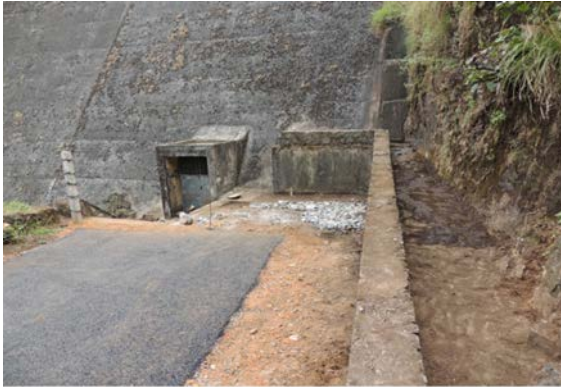
KAKKI DAM ADIT-I, BEFORE DRIP WORK
