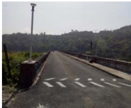
After - Dam Top Wearing coat
