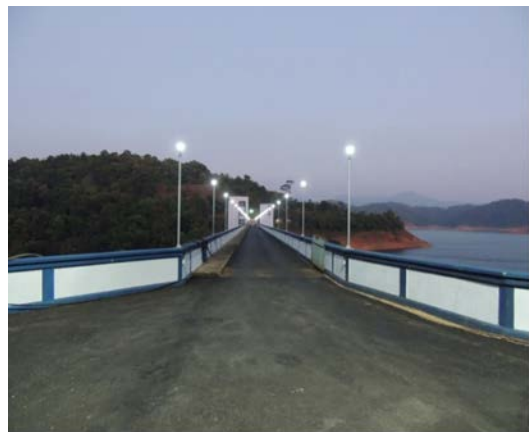
KAKKI DAM - POST TOP LANTERN - AFTER DRIP WORKS
