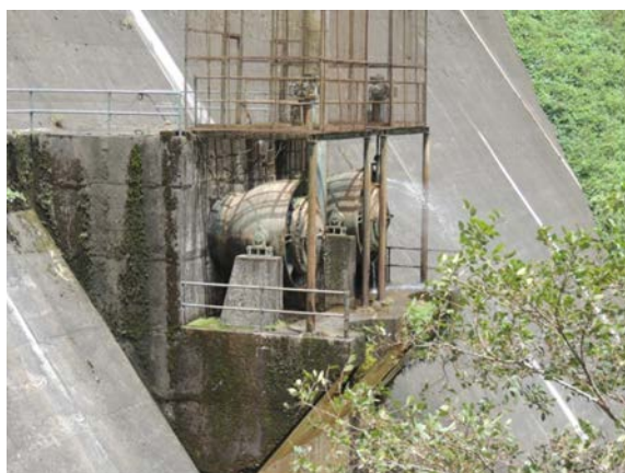
HOLLOW JET VALVE BEFORE REPAIRING
