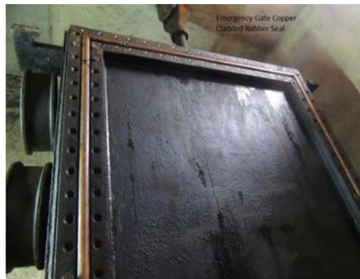
EMERGENCY GATE - AFTER REPAIR WORK
