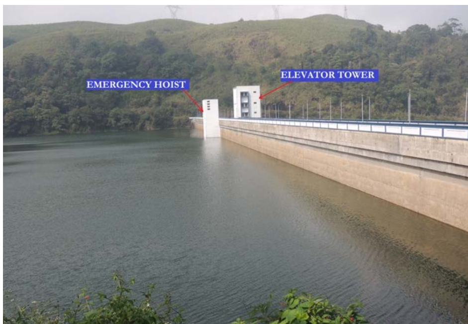
Fig 1.8b Dam Top and Upstream Elevation of Kakki dam
