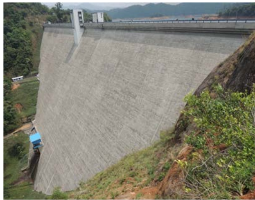
KAKKI DAM DS FACE AFTER PRESSURE WASHING
