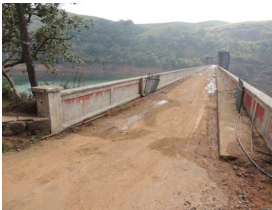
KAKKI DAM - POST TOP LANTERN - BEFORE DRIP WORKS
