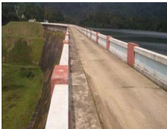
Before - Installation of top lantern
