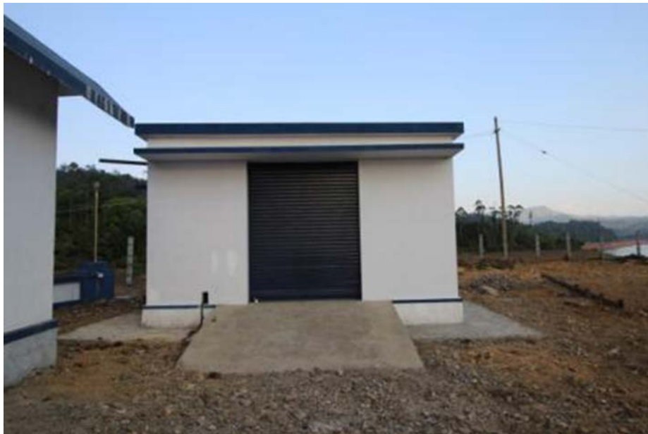
Construction of Generator room
