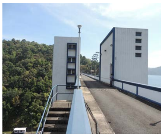
KAKKI DAM - AFTER PAINTING
