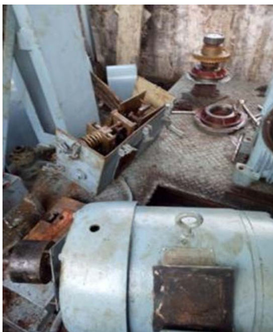
Before - Special repair to Hoist mechanism
