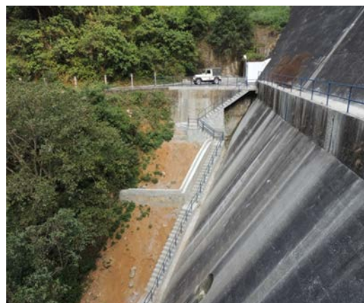
(AFTER) CONSTRUCTION OF STEPS TO V-NOTCH
