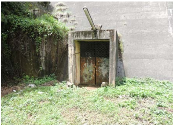
KAKKI DAM ADIT-II BEFORE DRIP WORKS
