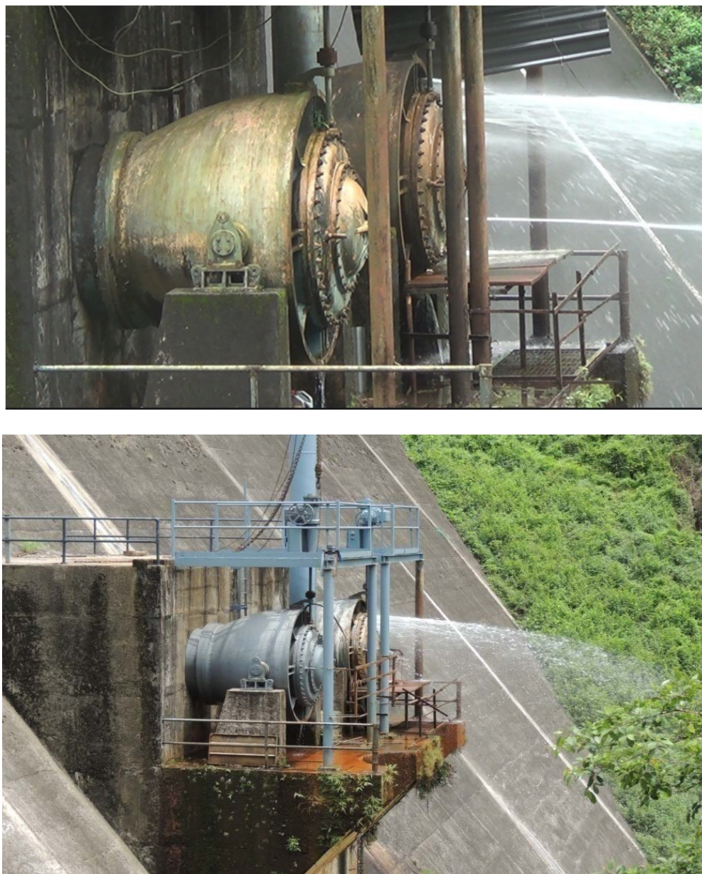
Fig 2.6 Hollow Jet Valves of Kakki Dam
