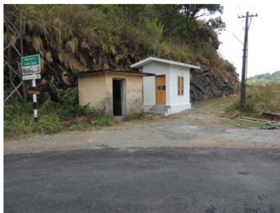
GUARD ROOM – LEFT BANK
