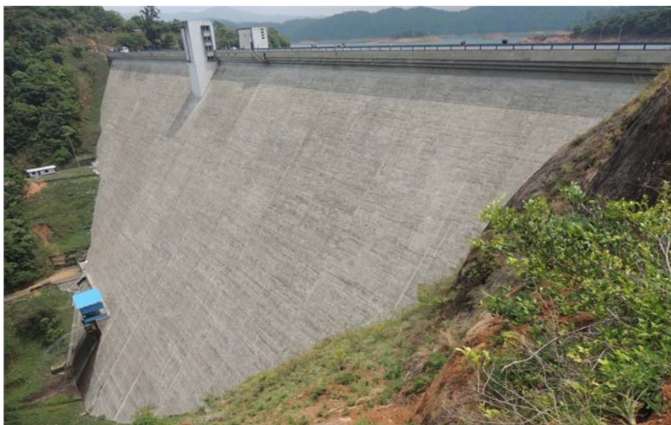
Fig 1.8a Downstream Elevation of Kakki dam
