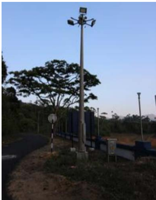
DRIP work - High mast light
