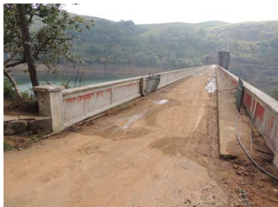
KAKKI DAM TOP ROAD - BEFORE DRIP WORKS
