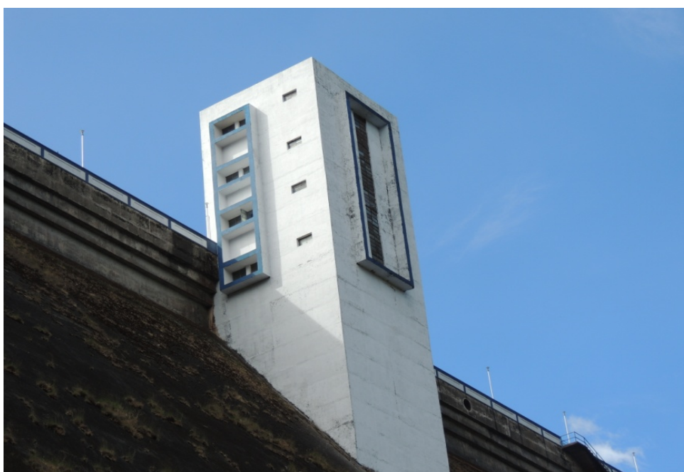
Fig 1.10 Elevator Tower at Kakki Dam
