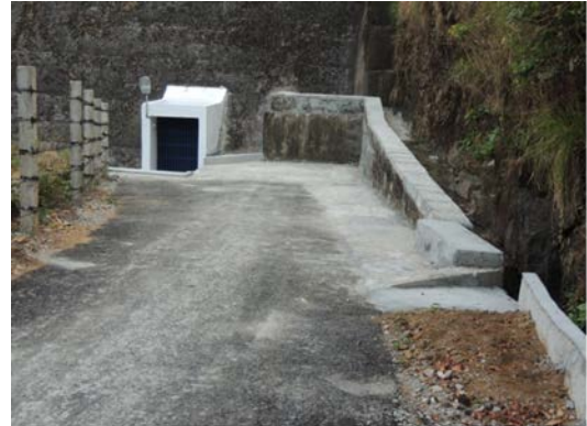
KAKKI DAM ADIT - I, AFTER DRIP WORKS
