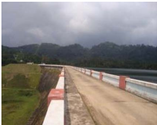
Before - Dam Top Wearing coat
