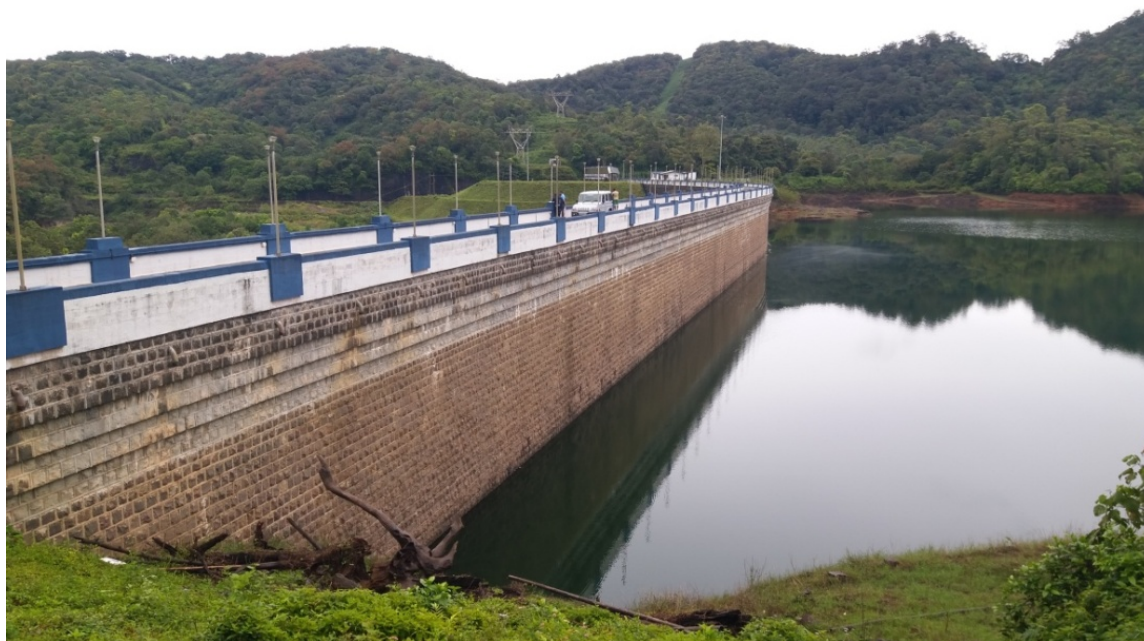
Fig 1.11a Upstream Elevation of Anathodu Dam
