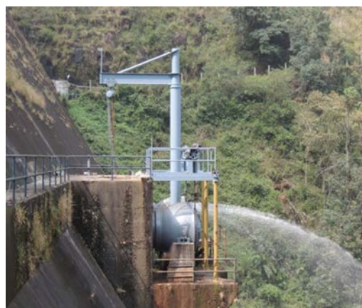
HOLLOW JET VALVE AFTER REPAIR WORK (RIGHT SIDE ONE)
