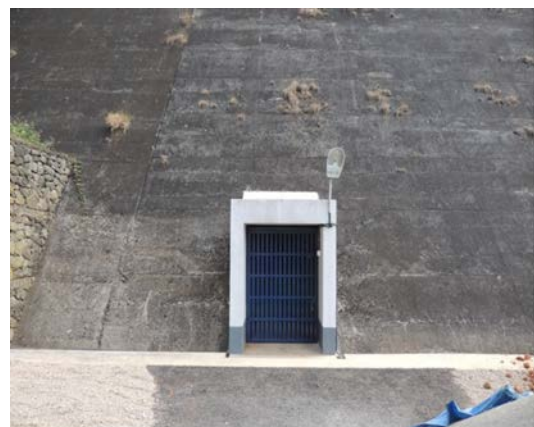
KAKKI DAM ADIT-III, AFTER DRIP WORKS
