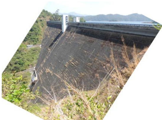
KAKKI DAM DS FACE PRESSURE WASHING (BEFORE WASHING)
