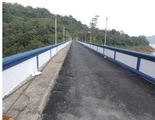
KAKKI DAM TOP ROAD - AFTER DRIP WORKS
