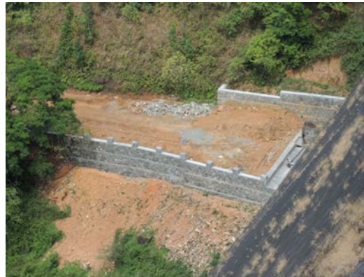
KAKKI DAM - D/S SIDE RETAINING WALL AFTER CONSTRUCTION
