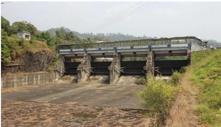
Fig 2.3a Downstream Elevation of Spillway - Anathodu Dam
