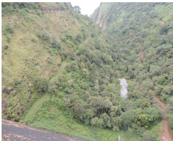
KAKKI DAM L/B & R/B ADIT ROADS BEFORE DRIP WORKS
