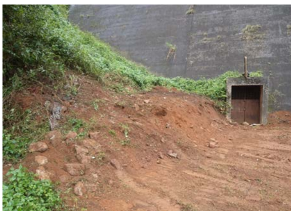
KAKKI DAM ADIT-III BEFORE DRIP WORKS
