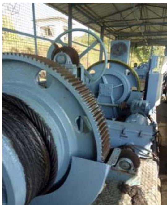
After - Special repair to Hoist mechanism
