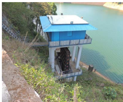
PROTECTIVE ROOFING TO INTAKE BUILDING - AFTER WORK
