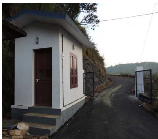
KAKKI DAM L/B ADIT-1 ROAD ENTRANCE AFTER DRIP WORKS
