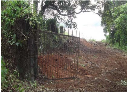
LOCATION OF GUARD ROOM NEAR INTAKE BEFORE CONSTRUCTION
