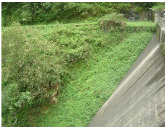
(BEFORE) CONSTRUCTION OF STEP TO V-NOTCH
