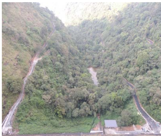
KAKKI DAM L/B & R/B ADIT ROADS AFTER DRIP WORKS
