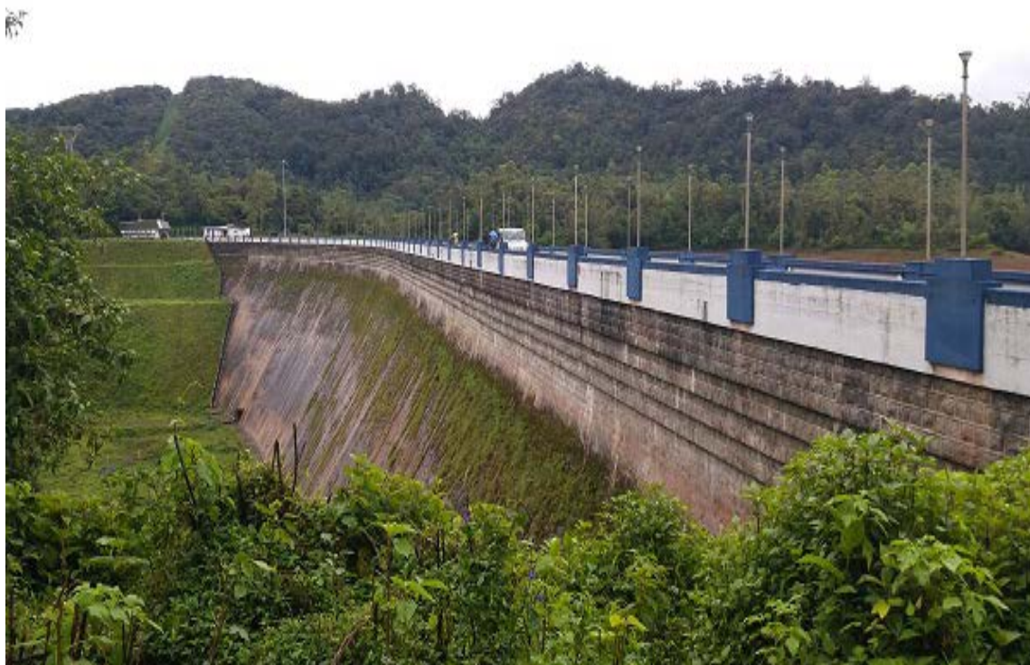
Fig 1.11b Downstream Elevation of Anathodu Dam
