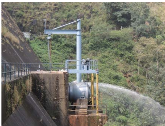
HOLLOW JET VALVE BEFORE ROOFING WORK
