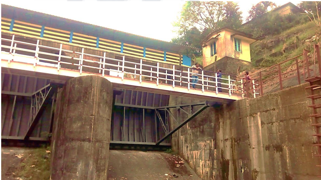
Fig 2.7 View of Spillway Gate Operation Bridge from downstream
