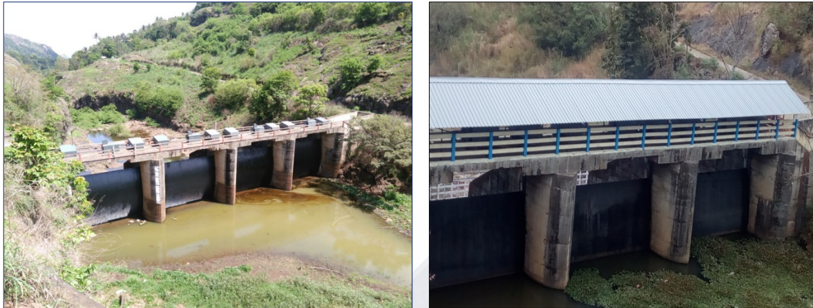
Kallar dam hoist bridge before and after roofing
