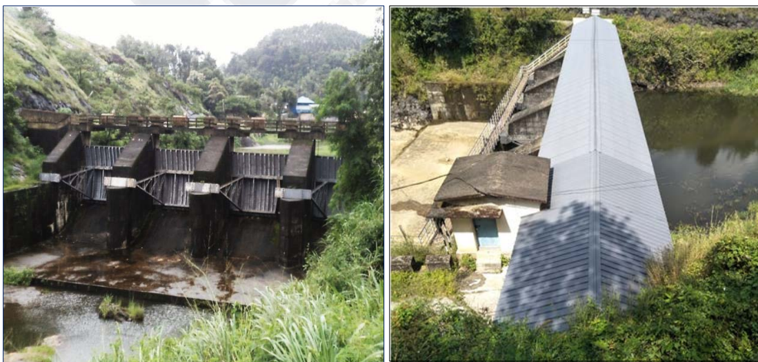
Kallar dam before & after DRIP 1
