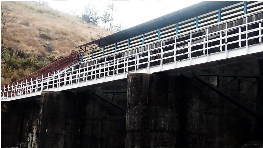
Kallar dam catwalk and access to downstream
