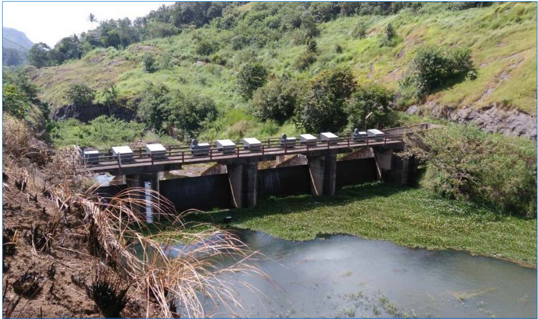
Fig 2.2b Upstream Elevation of Kallar Dam
