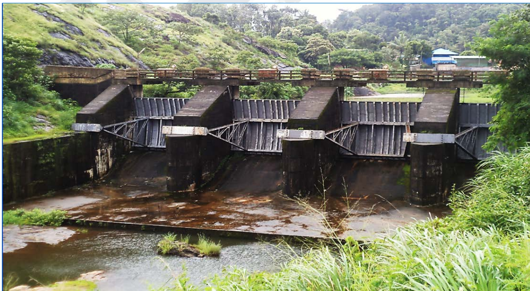
Fig 2.2a Downstream Elevation of Kallar Dam
