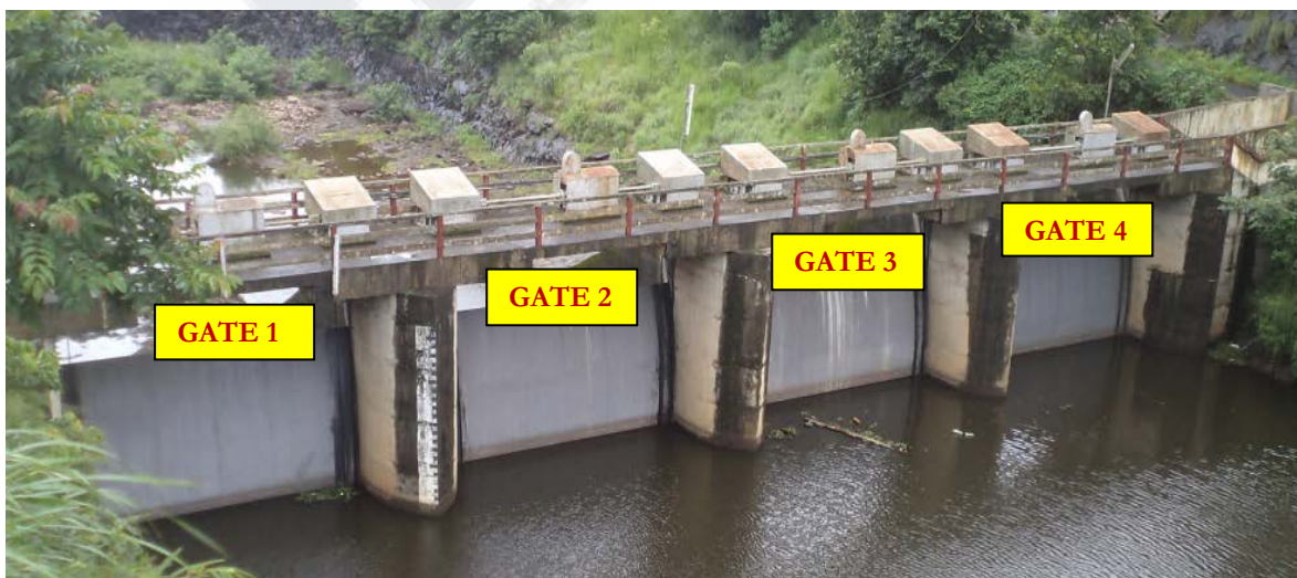
Fig 2.5 Kallar dam hoist platform
