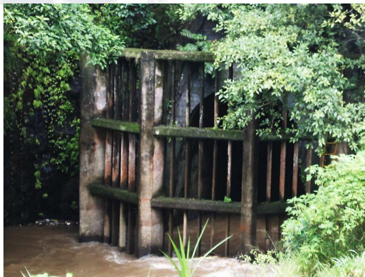
Fig 2.12 Entrance of Diversion Tunnel
