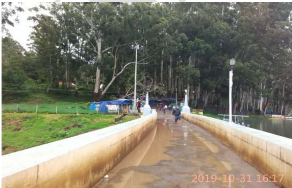
Fig 6.5 High mast light and parapet painting
