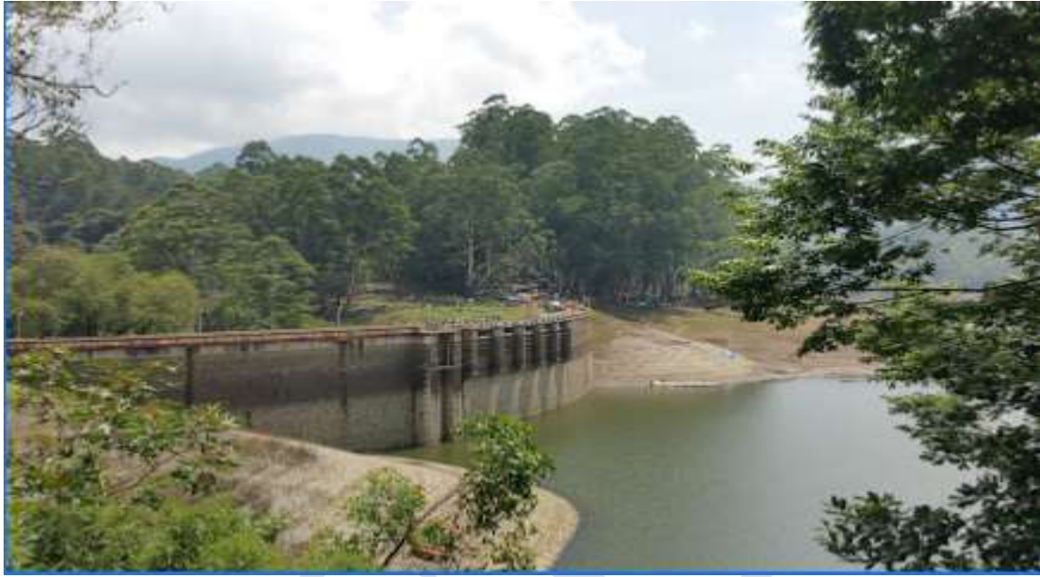
Fig 1.1 Kundala Dam – Upstream view
