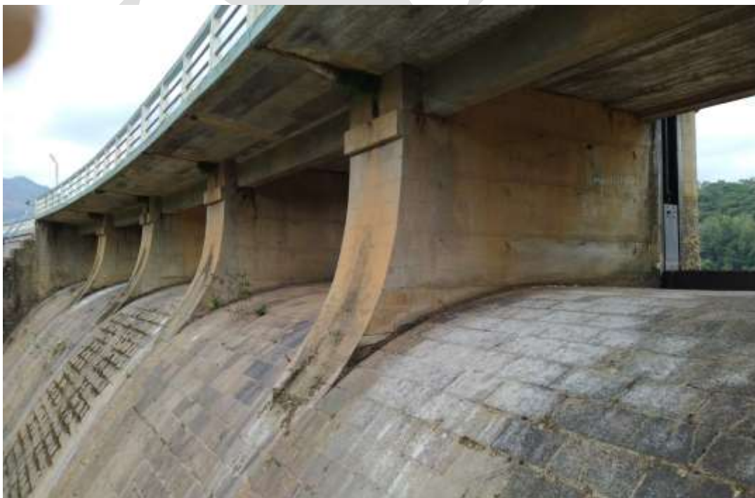
Fig 2.5 Spillway of Kundala dam
