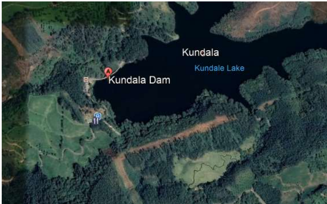
Fig 1.5 Kundala dam – View from Google Earth
