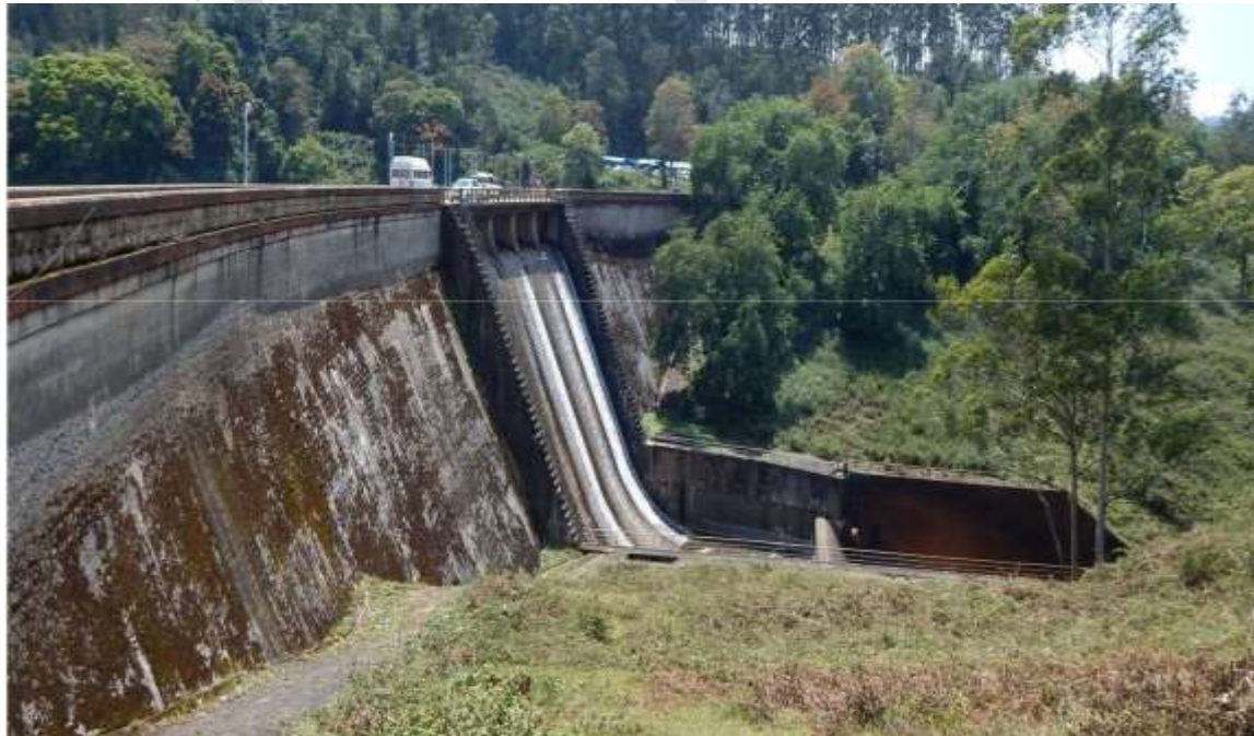
Fig 1.2 Kundala Dam – Downstream view
