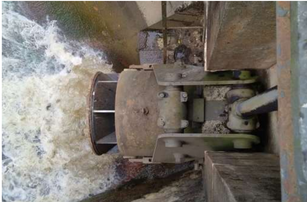
Fig 2.12 Disperser valve
