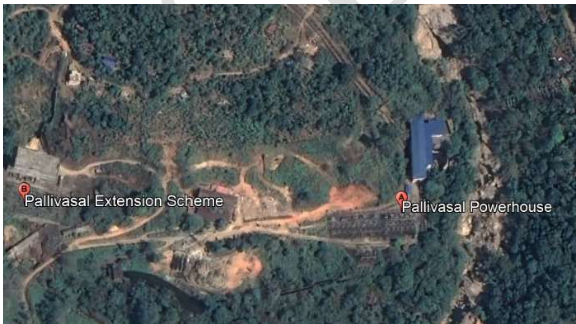
Fig 1.6 Pallivasal Power House – View from Google Earth
