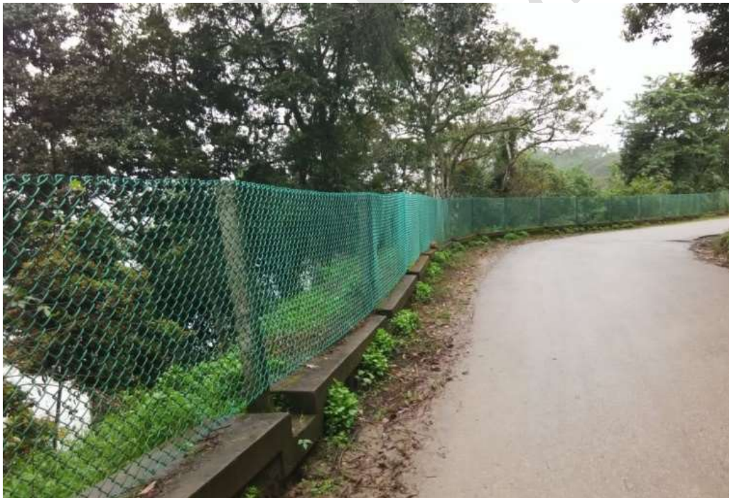
Fig 6.1 Fencing and road work
