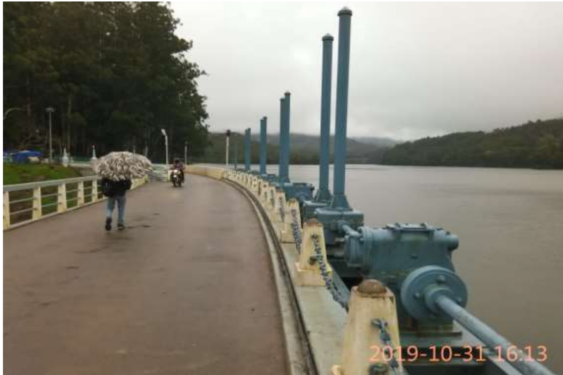
Fig 6.4 Hoisting mechanism after painting
