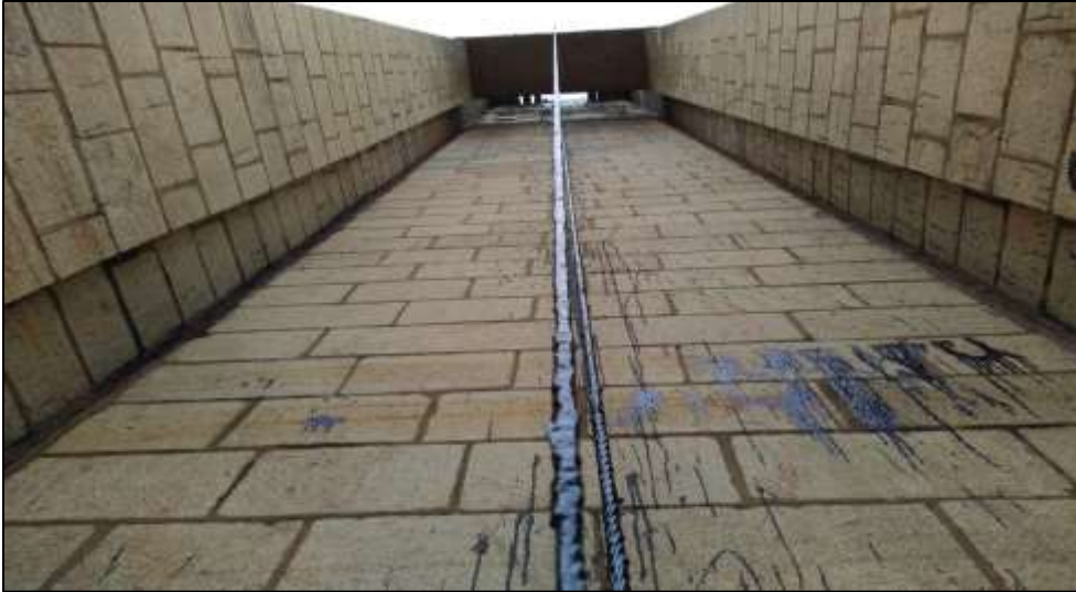
Fig 2.10 Emergency gate guiding column
