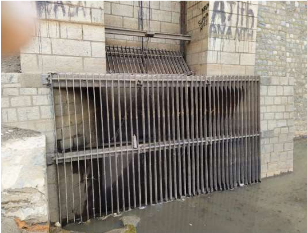
Fig 2.9 Trash rack
