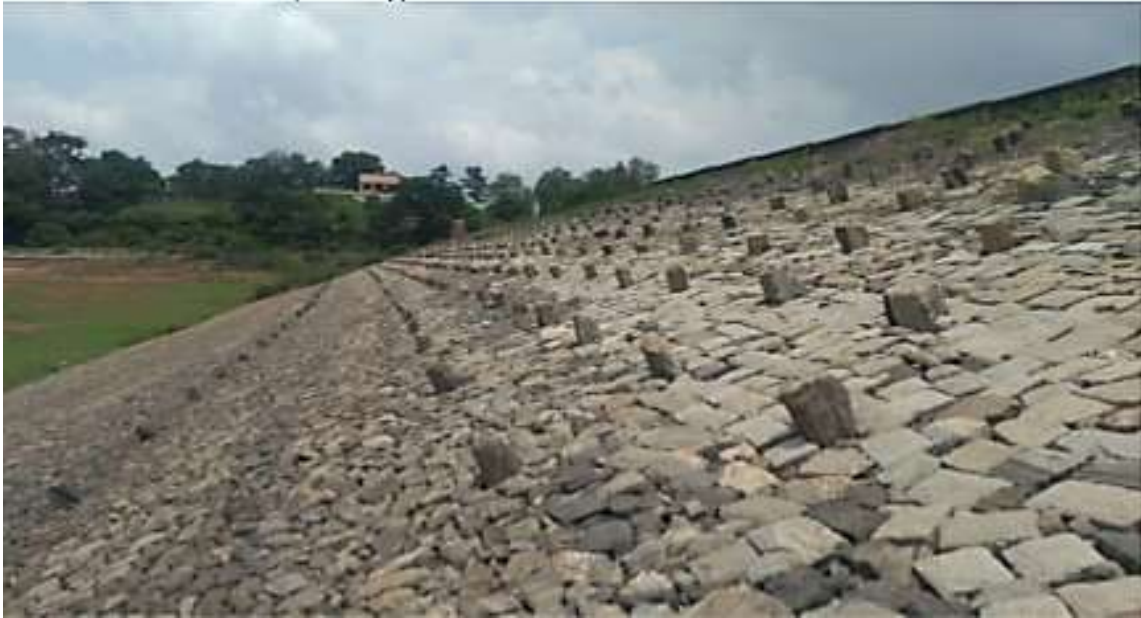
Fig 4.1 Upstream rip rap
