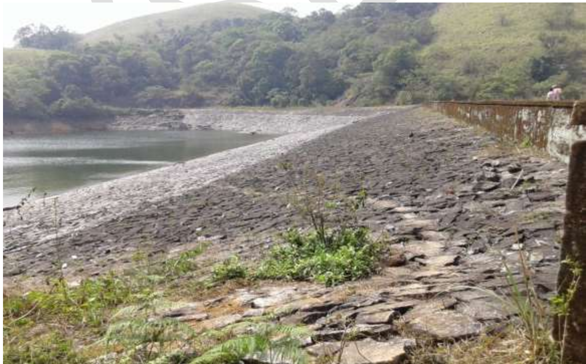
Fig 2.20 Rubble packing – upstream side of Kosani Saddle Dam
