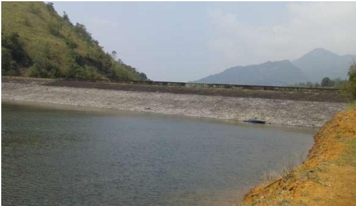
Fig 2.19 Upstream view of Kosani Saddle Dam
