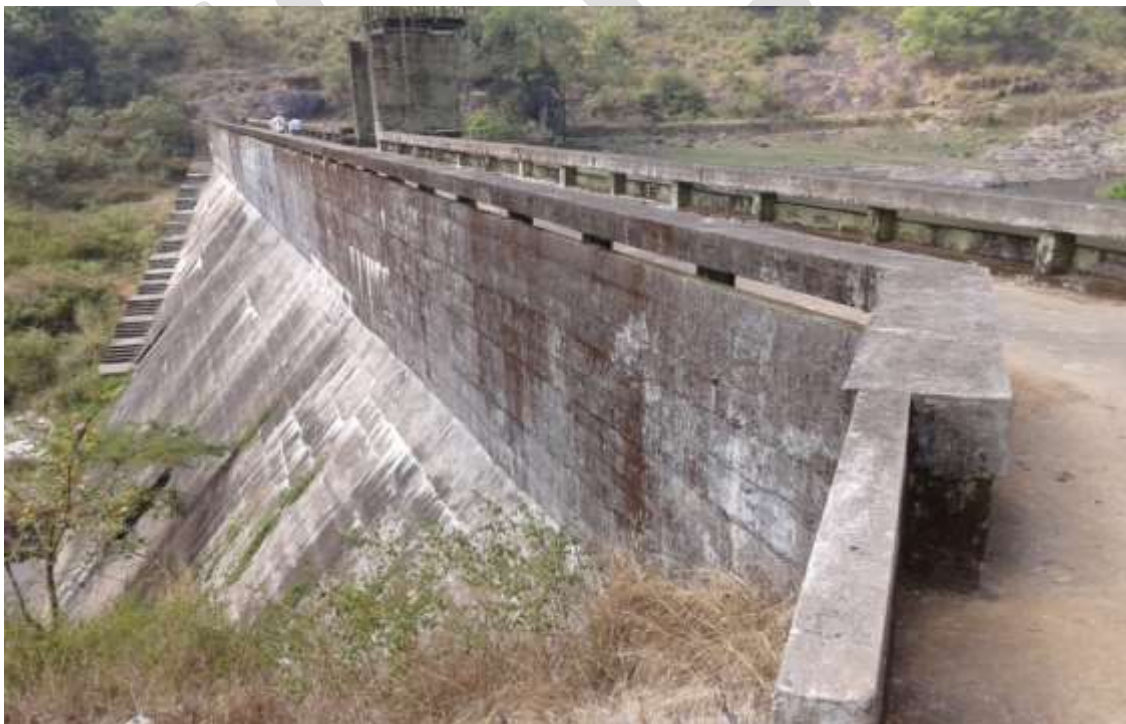
Fig 2.14 Downstream view of Kuttiyadi Saddle Dam
