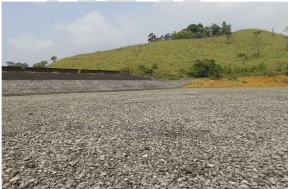
Fig 2.16 Rubble packing – upstream side of Kottagiri saddle dam
