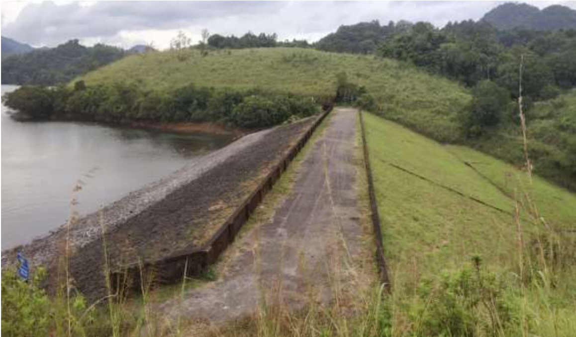
Fig 1.8 Saddle dam near Kottagiri
