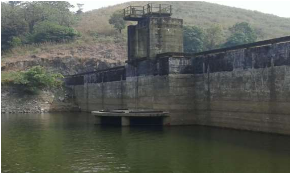
Fig 2.13 Upstream view of Kuttiyadi Saddle Dam
