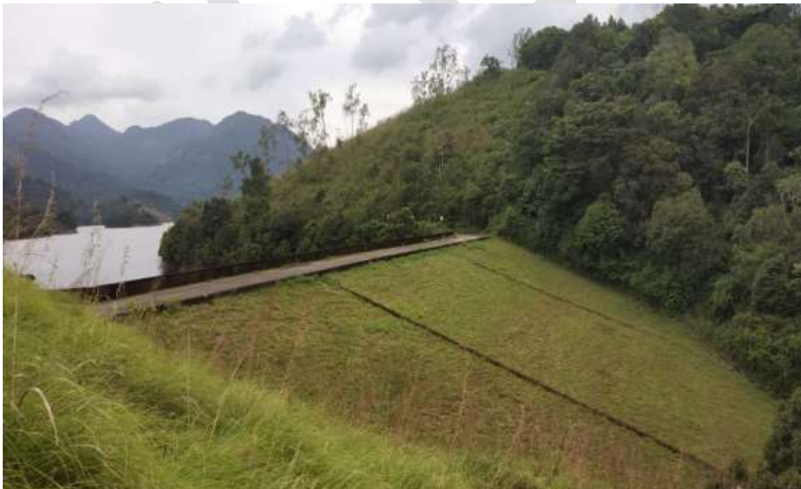
Fig 1.7 Kottagiri saddle dam
