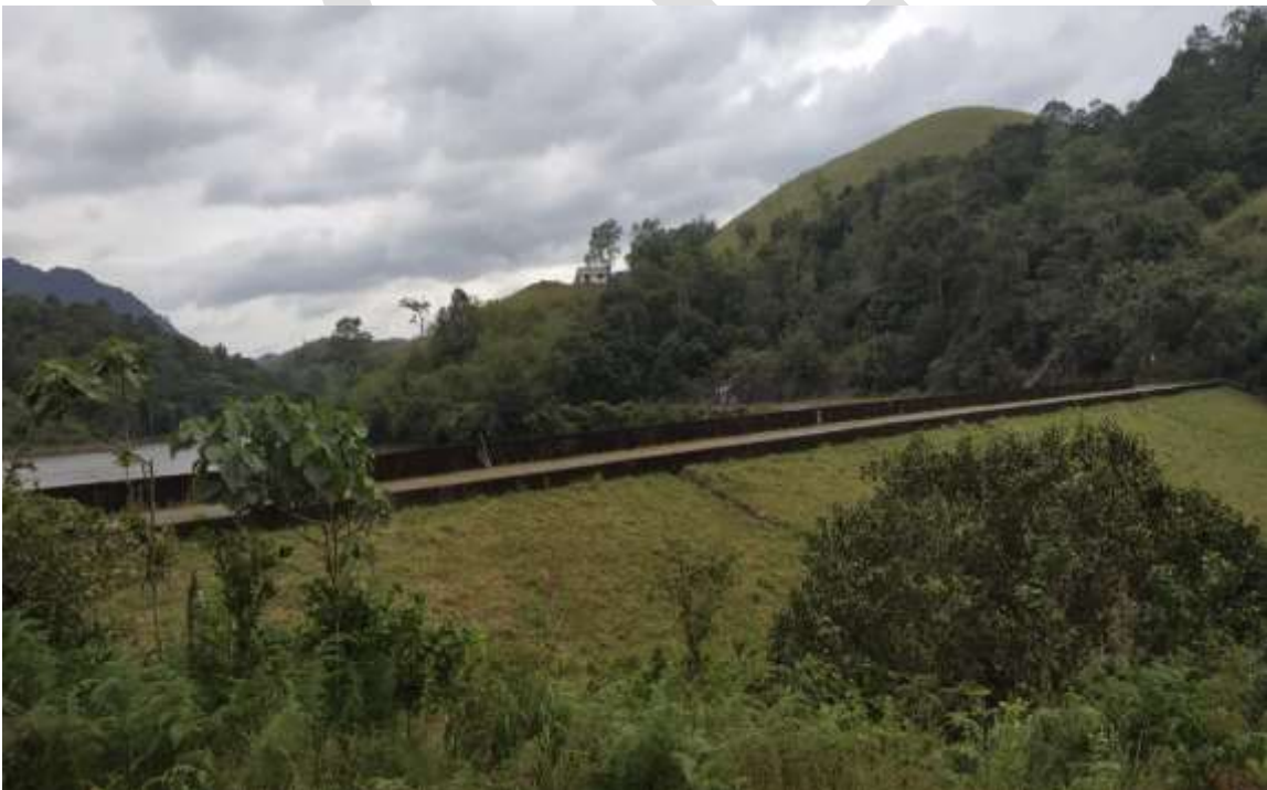
Fig 1.9 Kosani saddle dam
