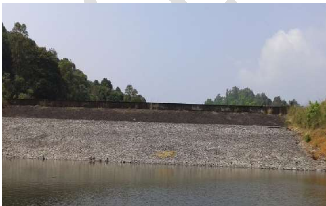
Fig 2.17 Upstream view of saddle dam near Kottagiri
