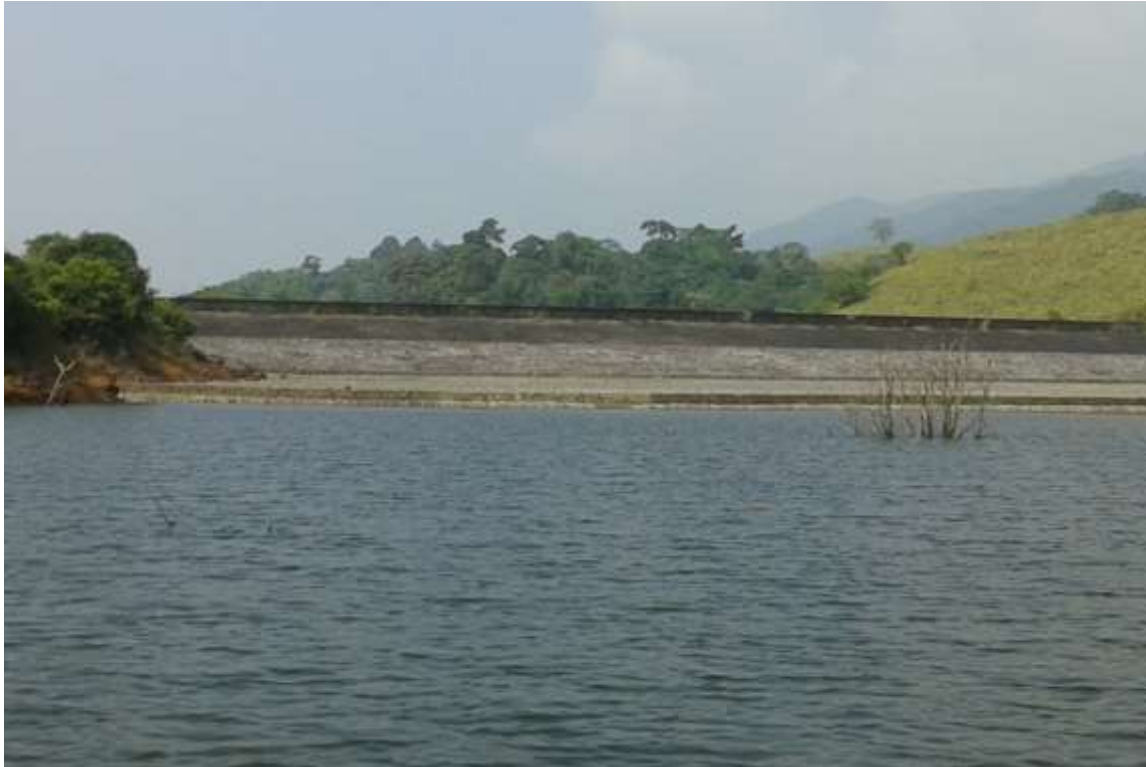
Fig 2.15 Upstream view of Kottagiri Saddle Dam
