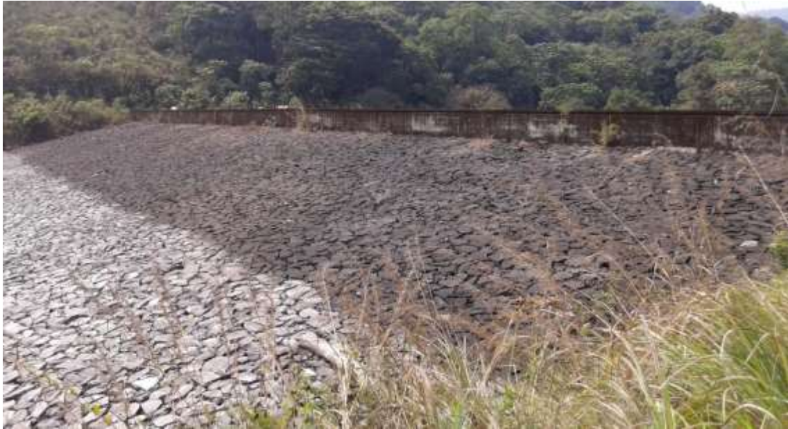
Fig 2.18 Rubble packing – upstream side of saddle dam near Kottagiri
