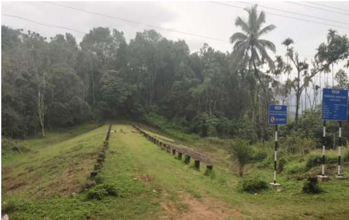
Fig 1.10 Manjoora saddle dam
