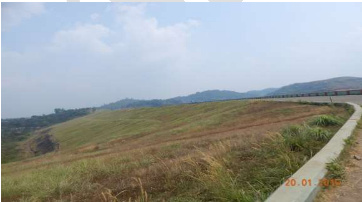
Fig 2.11 Down Stream View of Main Dam
