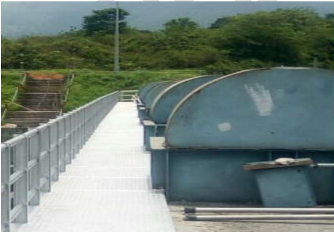
Fig 6.3 Steel walkway at spillway
