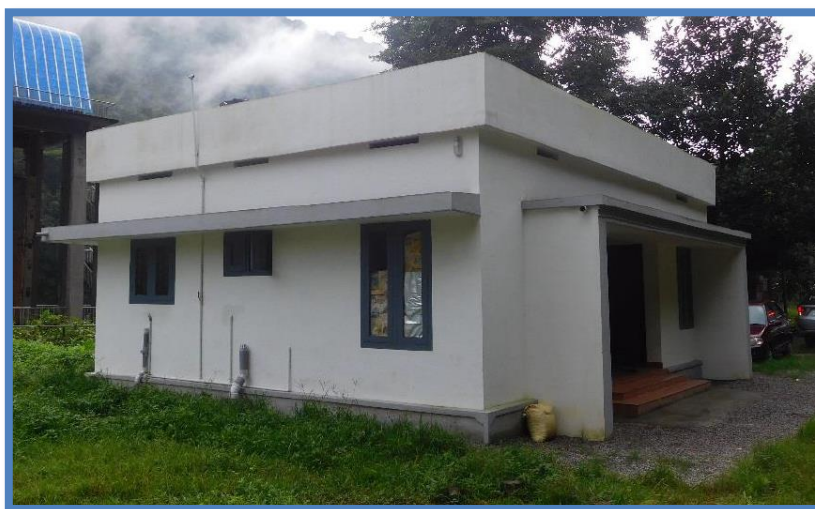
Fig 6.8 Photograph showing Security cabin cum Control Room
