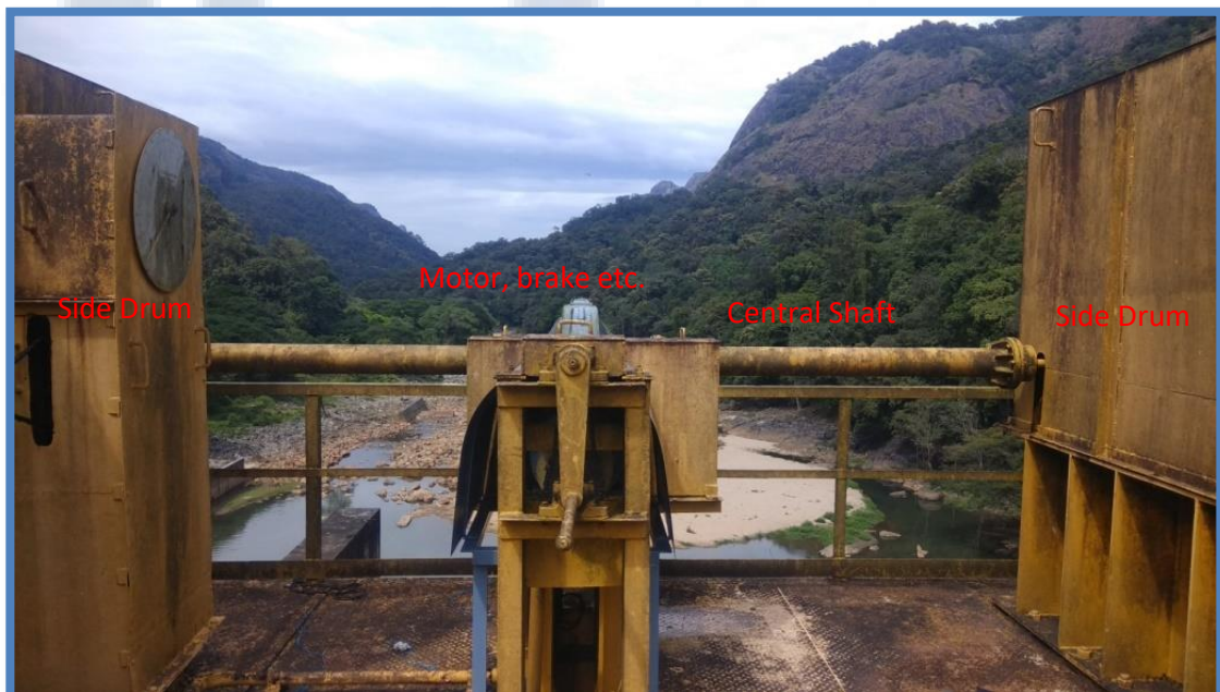
Fig 2.7 Photograph Showing Hoisting arrangements of Radial gate for Upper vent
