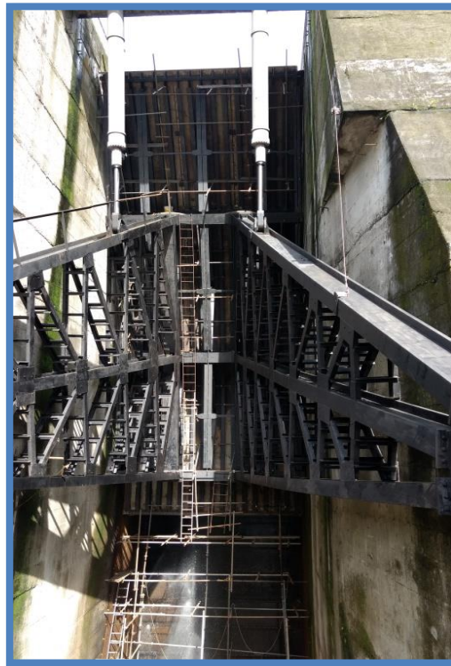
Fig 6.6 View of Repairs to low vents gates
