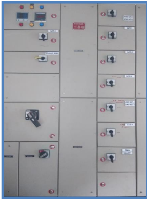
Fig 2.11 Photograph of Main DB- LP Dam
