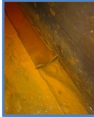
Fig 5.3 V notch in gallery of Lower Periyar dam
