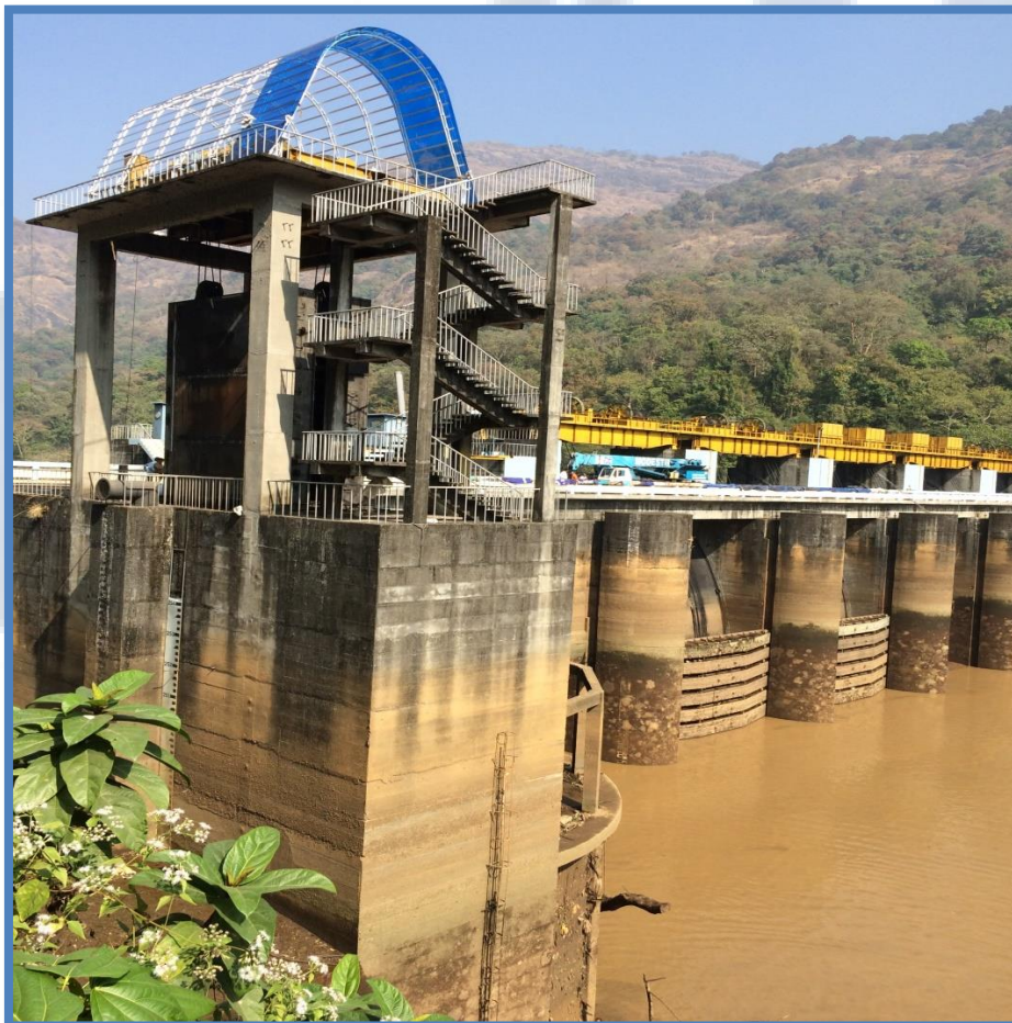
Fig 1.11 View of upstream
