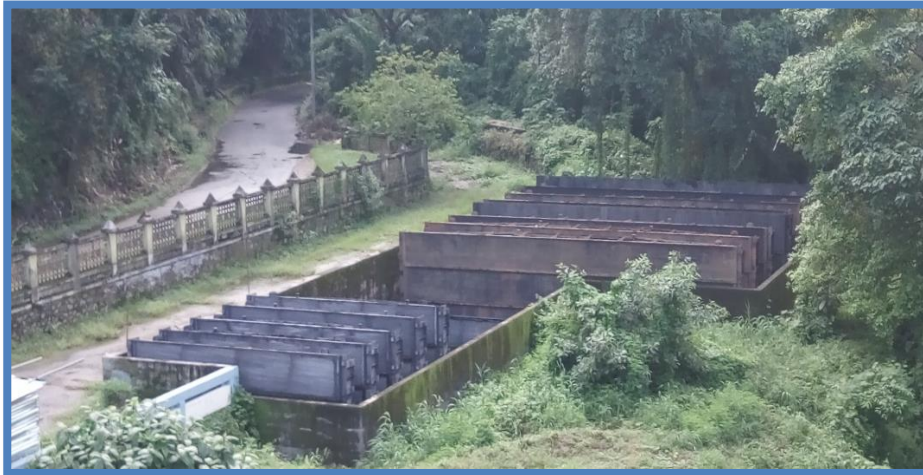
Fig 2.14 Stop log gates
