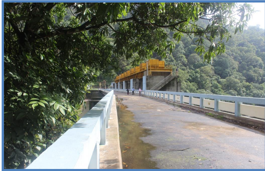
Fig 1.10 View from right abutment
