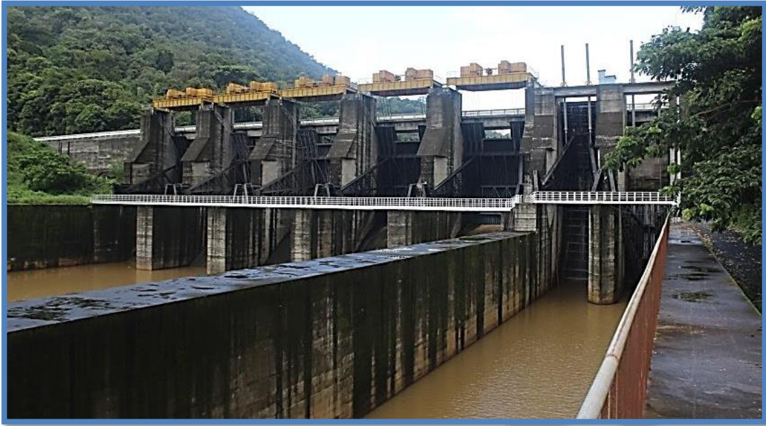
Fig 1. 8 View of Lower Periyar Dam gates
