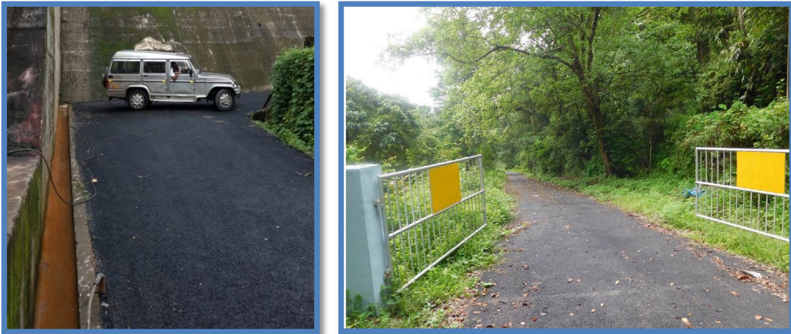
Fig 6.2 Photograph showing Road to Foundation Gallery
