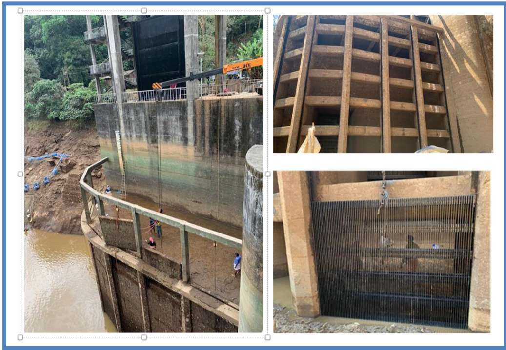
Fig 6.10 Photographs of Trash rack replacement Work
