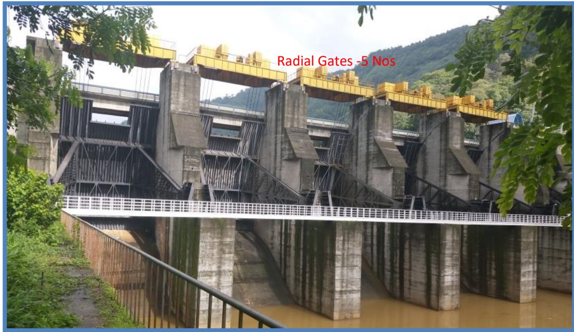
Fig 2.6 Photograph Showing Upper vent (Radial Gate) of Lower Periyar Dam
