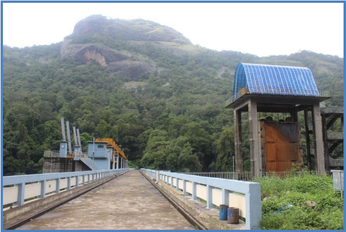
Fig 2.1 Photograph showing an overall view of Lower Periyar Dam
