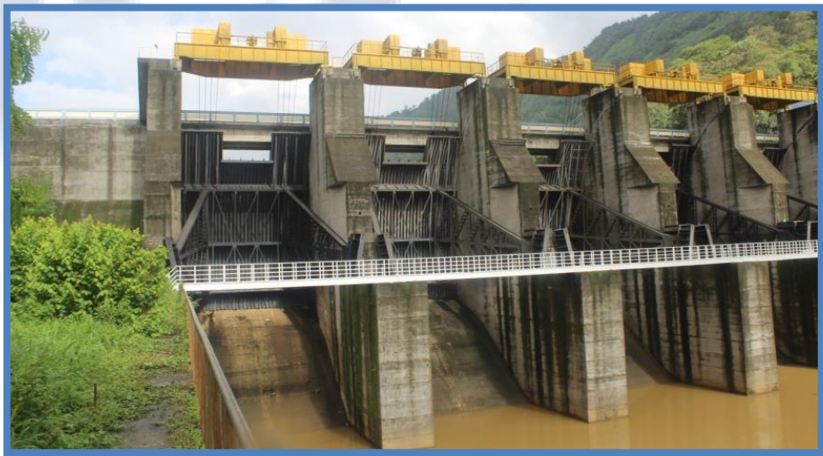
Fig 6.5 Photograph showing Catwalk
