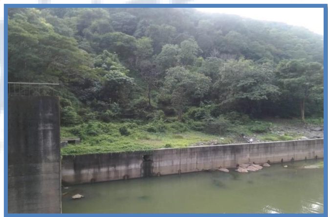
Fig 6.7 Photograph showing River training works
