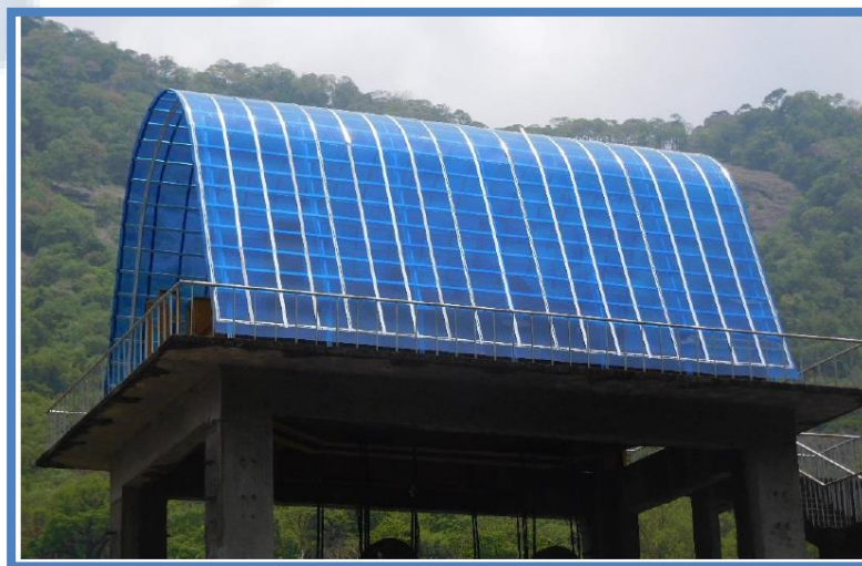
Fig 6.1 Photograph showing Intake Gate Roof
