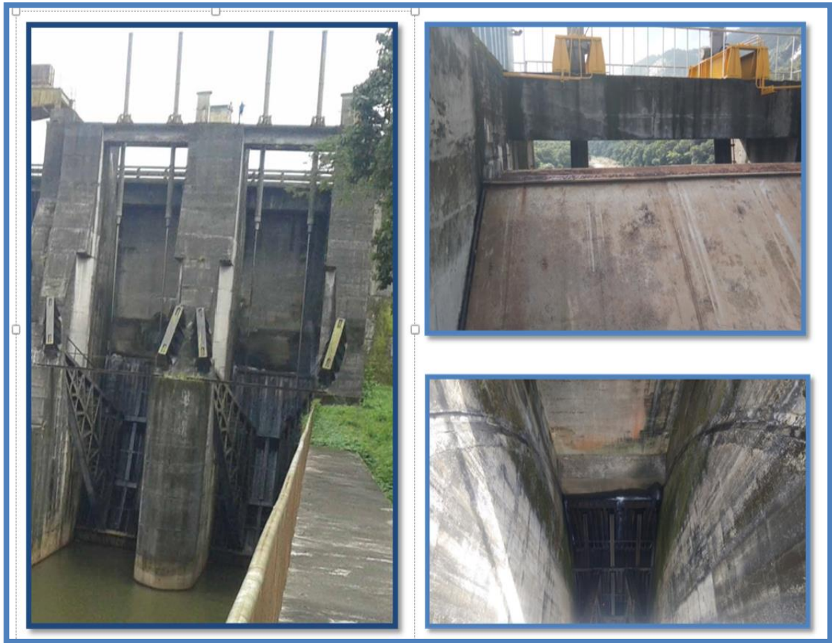
Fig 2.9 Photograph of Lower vent gate showing top and upstream view
