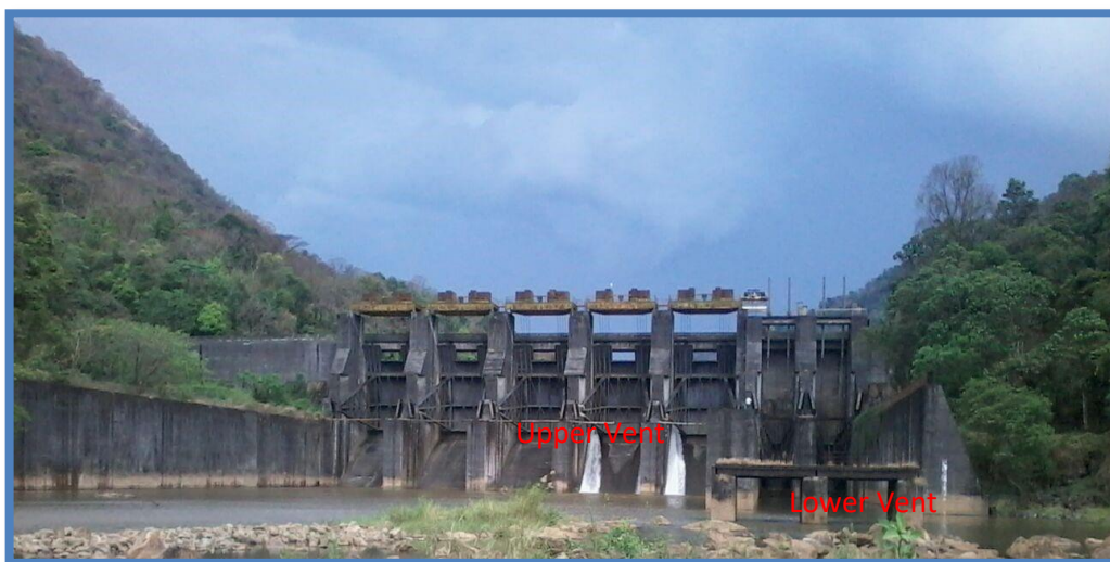
Fig 2.2 Photograph Showing Spillway and River outlet of dam
