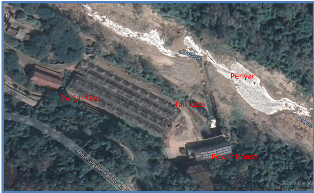
Fig 1.12 Google View of LPHEP Power House
