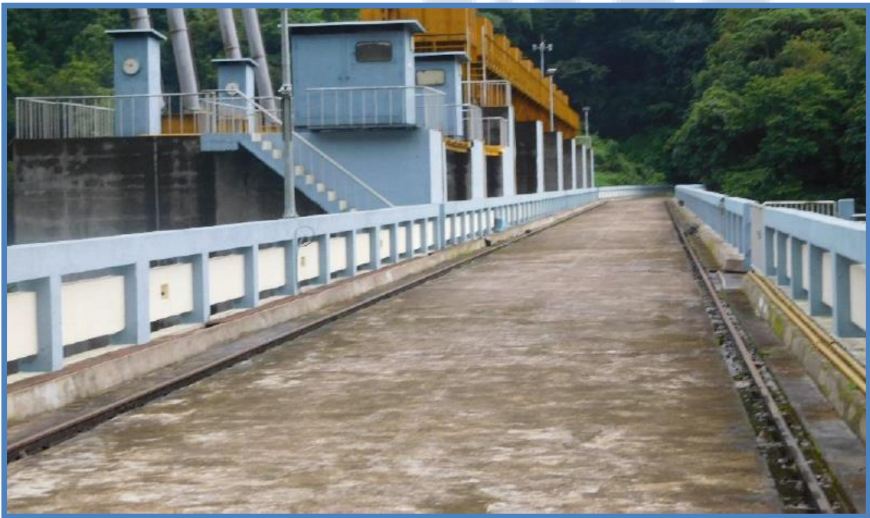
Fig 6.3 Pressure washing and Painting of parapet
