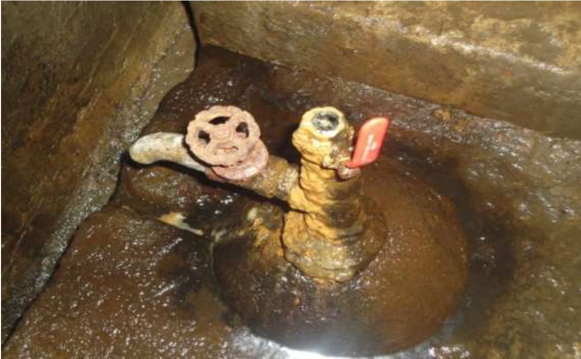
Fig 5.1 Drain hole FDH No.7
