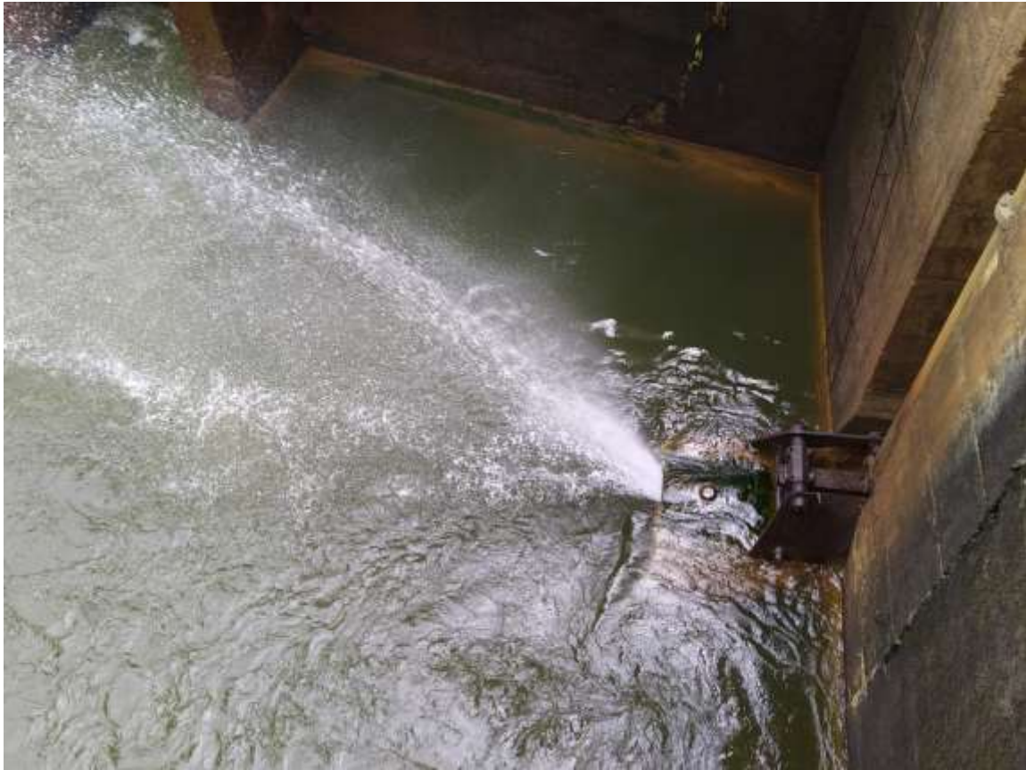
Fig 2.7 Disperser valve
