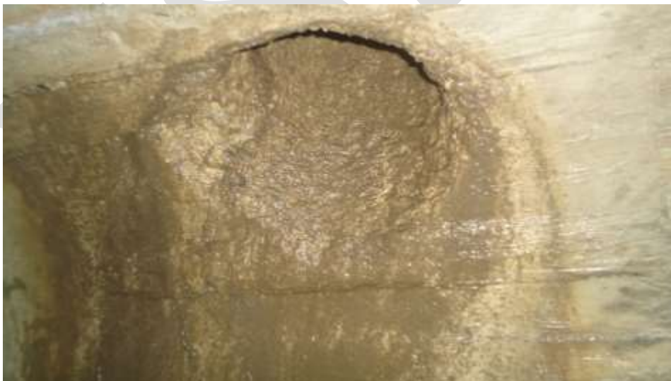
Fig 5.2 Drain hole BDH No.7
