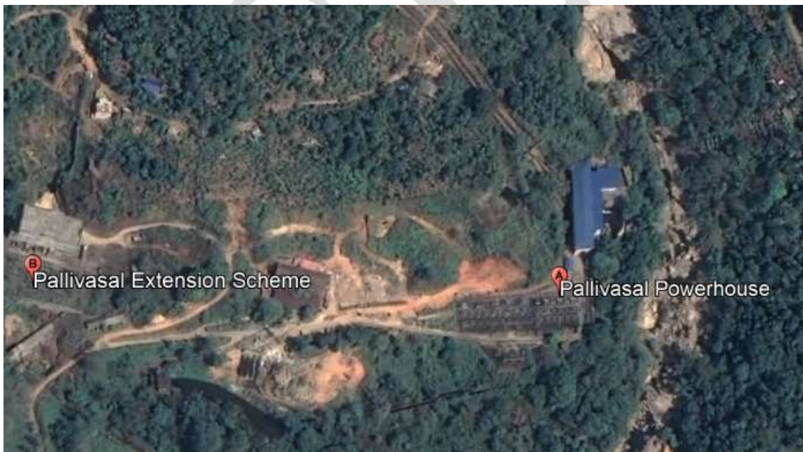
Fig 1.6 Pallivasal Power House – View from Google Earth
