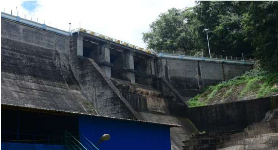
Fig 2.4 Spillway of Madupetty dam
