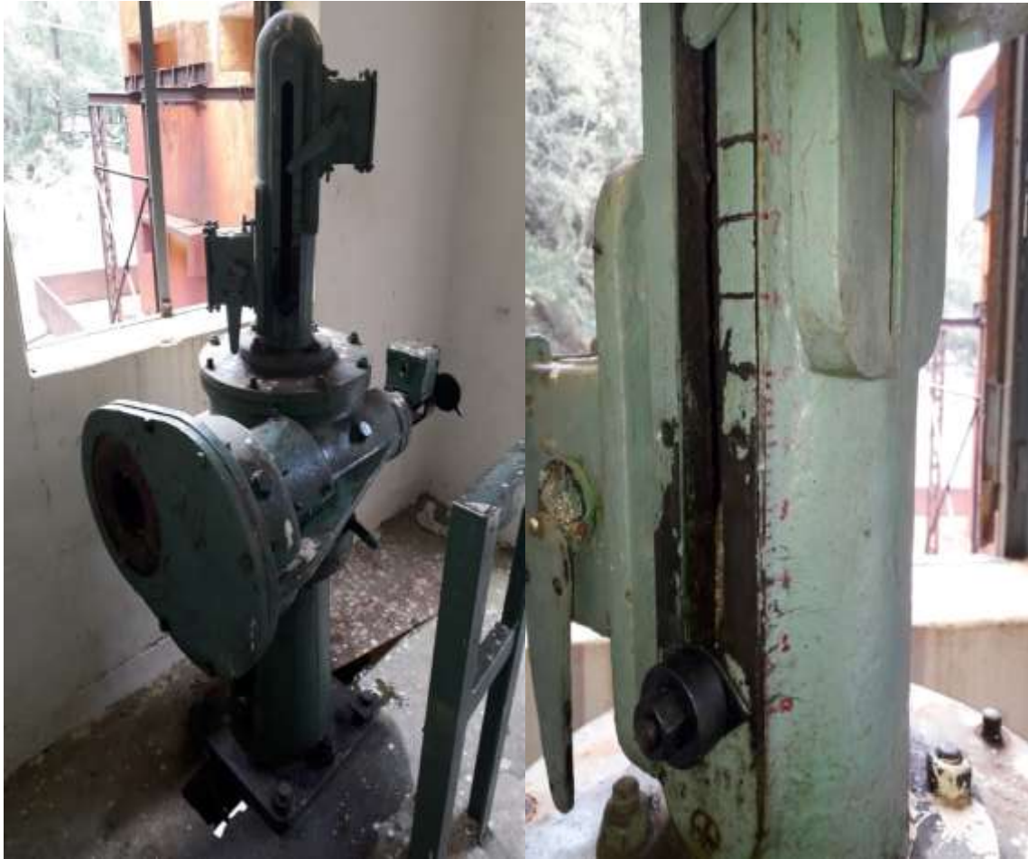
Fig 2.10 HB valve hoist and dial
