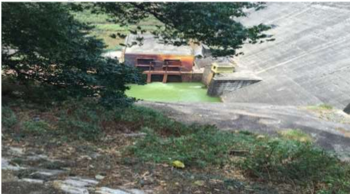
Fig 2.11 HB valve discharge
