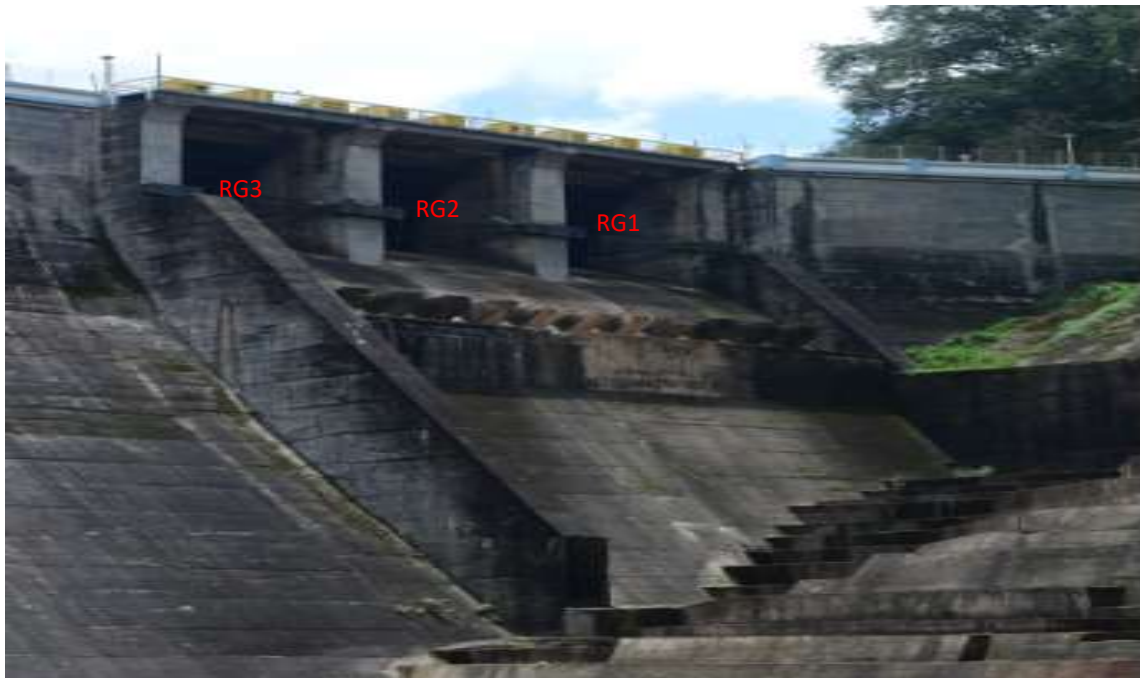
Fig 2.19 Spillway radial gates
