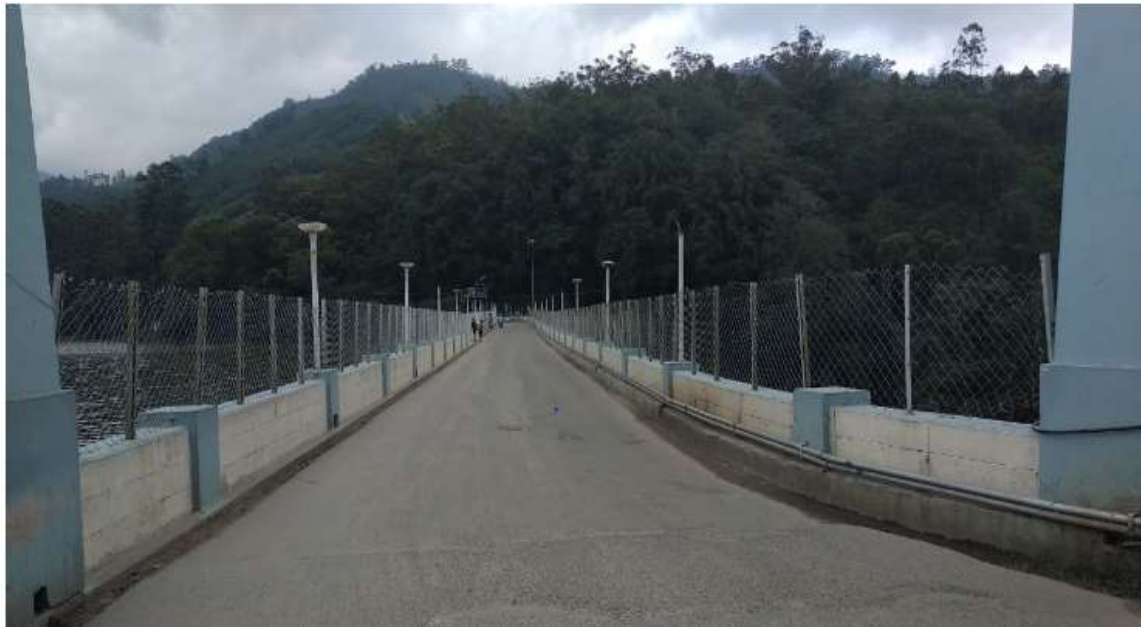
Fig 6.2 Parapet painting and security fencing
