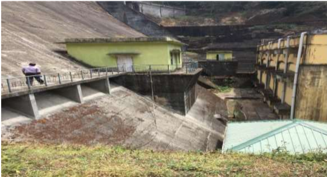
Fig 2.15 Gallery outlet and entry well
