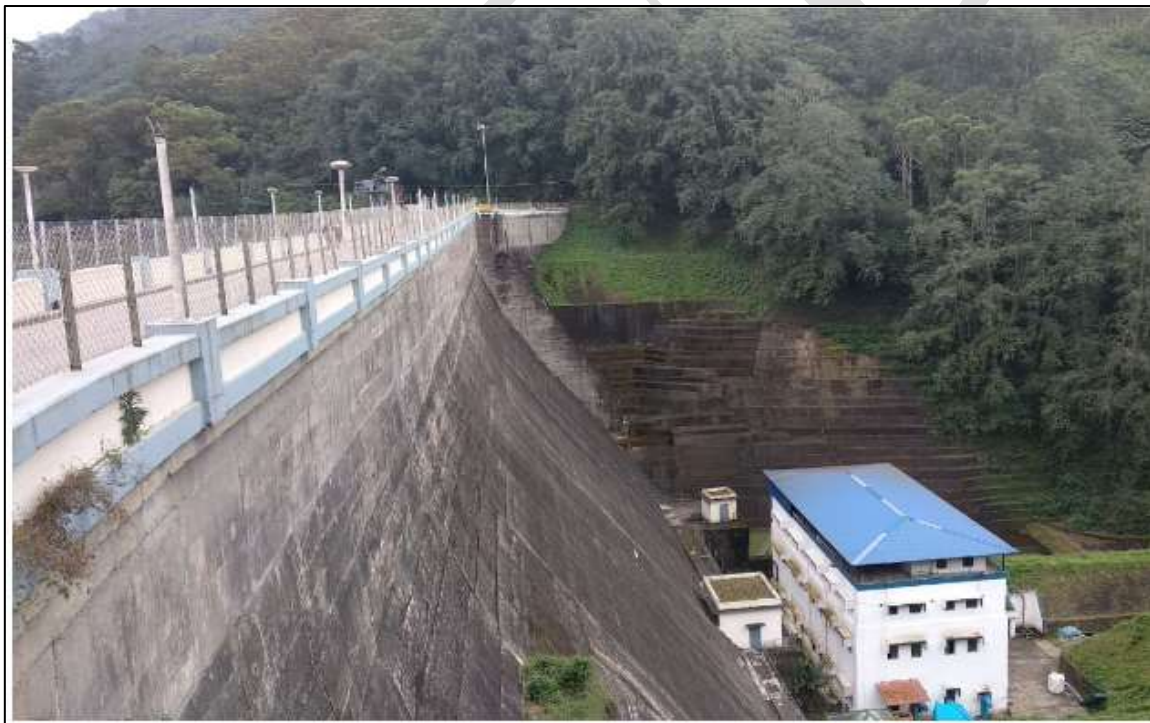
Fig 6.1 Pressure washing of dam
