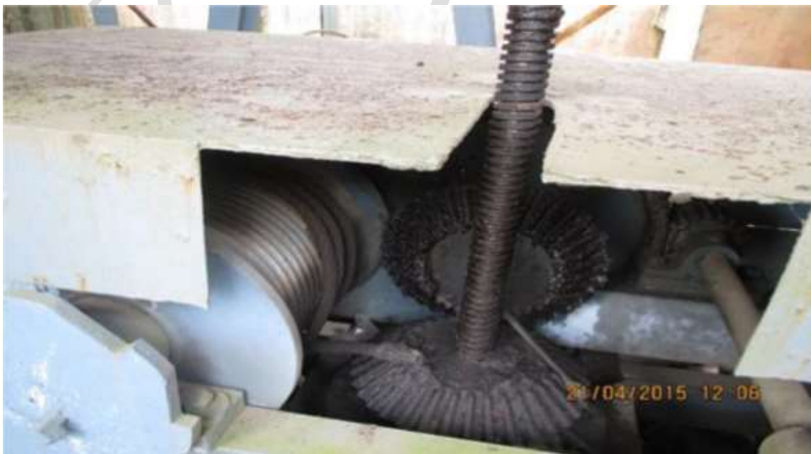
Fig 2.9 Emergency gate screw hoist
