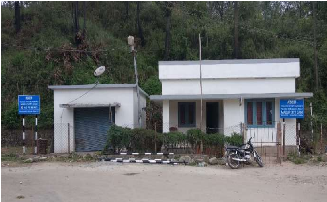
Fig 6.4 Security guard room
