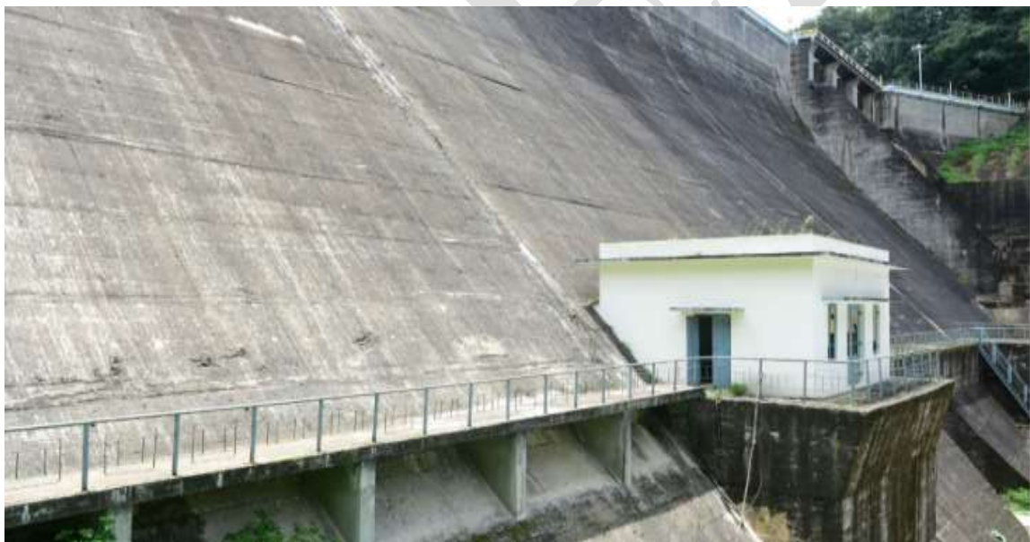
Fig 2.3 Madupetty dam – downstream view
