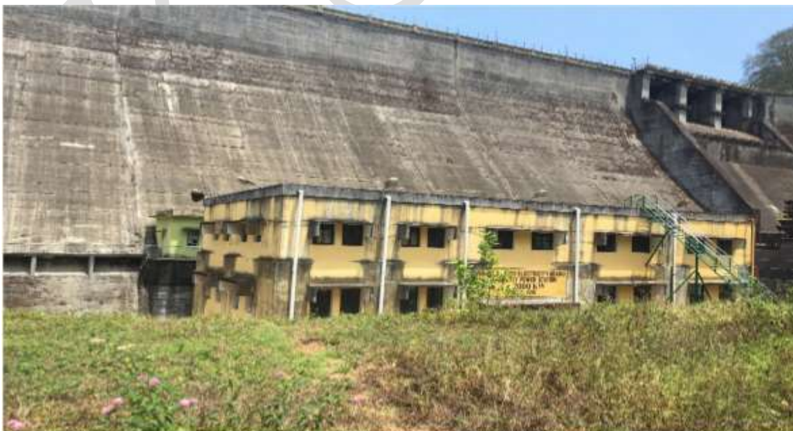
Fig 2.21 Dam toe power house
