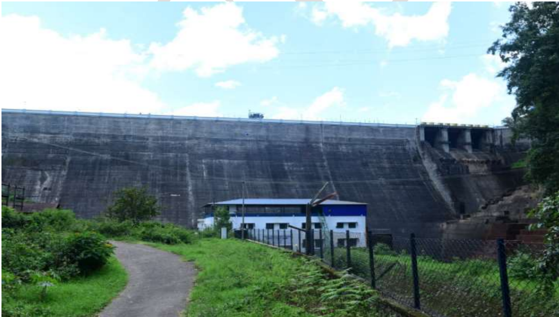
Fig 1.2 Madupetty Dam – Downstream view
