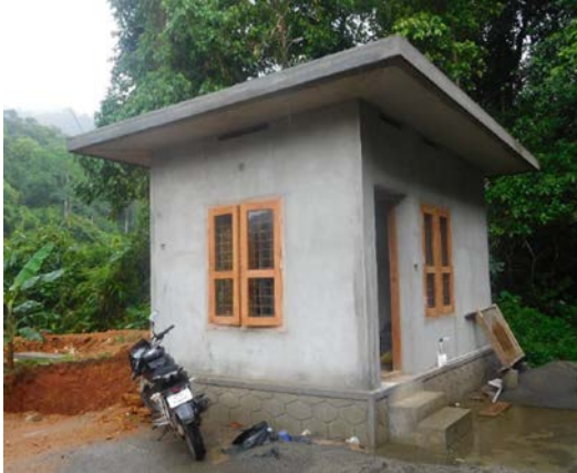
Construction of monitoring cabin
