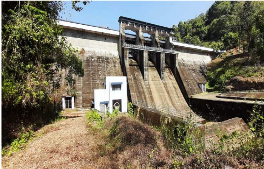
Fig 1.7 Spillway of Moozhiyar dam
