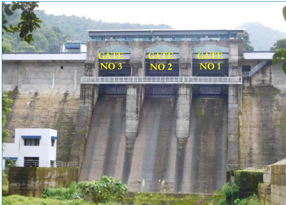
Fig 2.9 General View of Spillway Hoist Bridge
