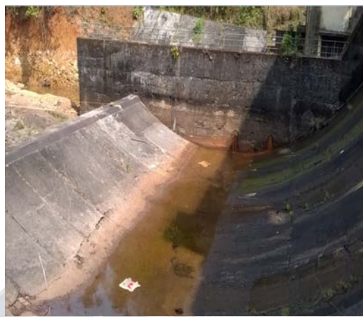
Repair works to the spillway bucket
