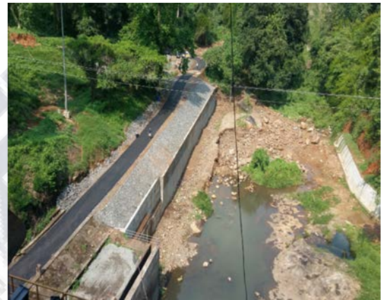
After - Extension of concrete retaining wall of L/B road at downstream
