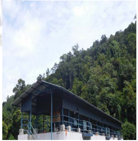
After - Protective roofing to the hoist of radial gates
