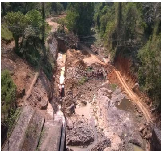
Before - Extension of concrete retaining wall of R/B road at
