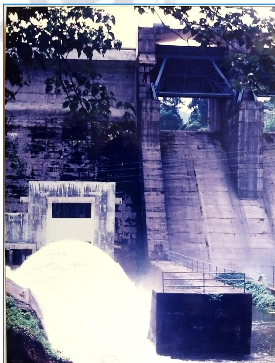
Fig 2.5b Disperser valve when opened first
