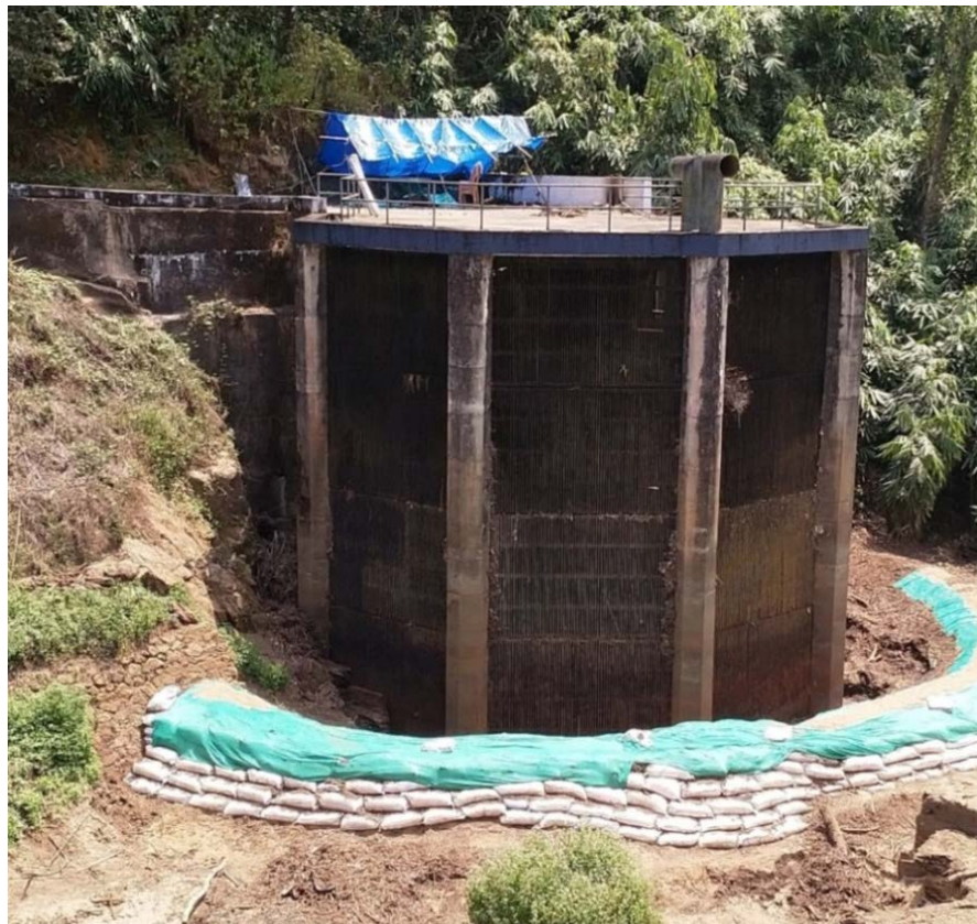
Fig 2.17 Intake shaft at Veluthode reservoir
