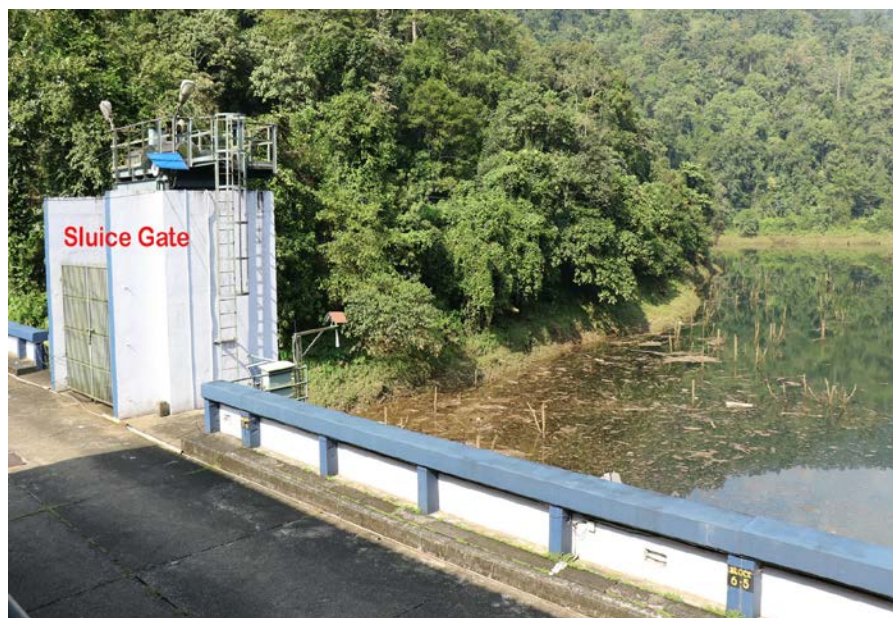
Fig 2.6 Sluice Gate Hoist
