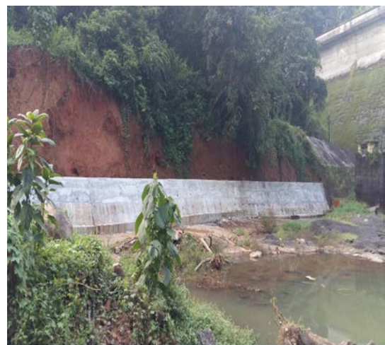
After - Extension of concrete retaining wall of R/B road at downstream
