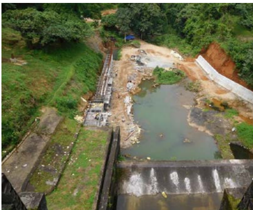
During - Extension of concrete retaining wall of L/B road at
