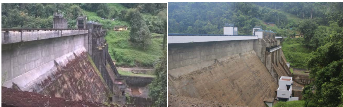
Pressure washing the downstream face before and after
