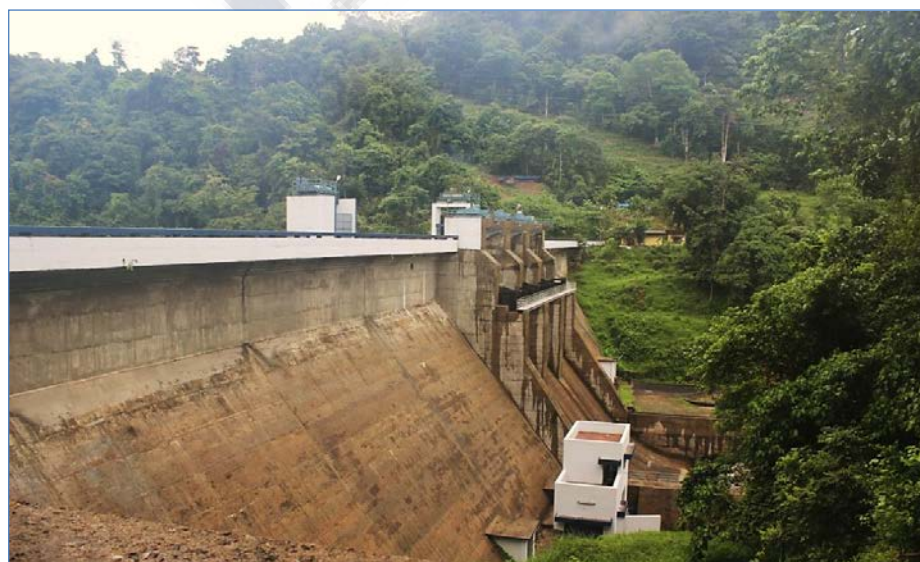
Fig 1.5a Downstream View of Moozhiyar Dam
