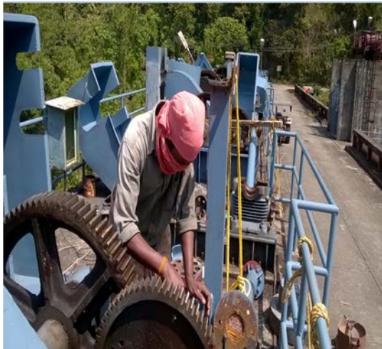
Before - Repairs to the radial gates
