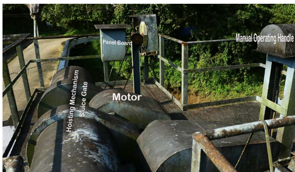
Fig 2.12b Sluice gate hoist mechanism
