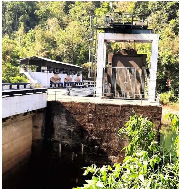
Fig 1.10 Intake Gate of Moozhiyar dam
