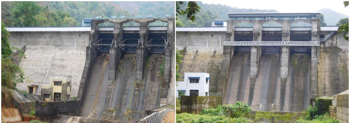
Spillway catwalk before and after
