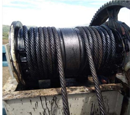
After - Repairs to the radial gates
