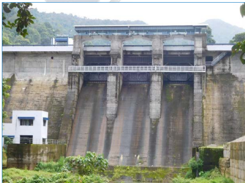
Fig 2.3 Spillway of Moozhiyar Dam downstream view
