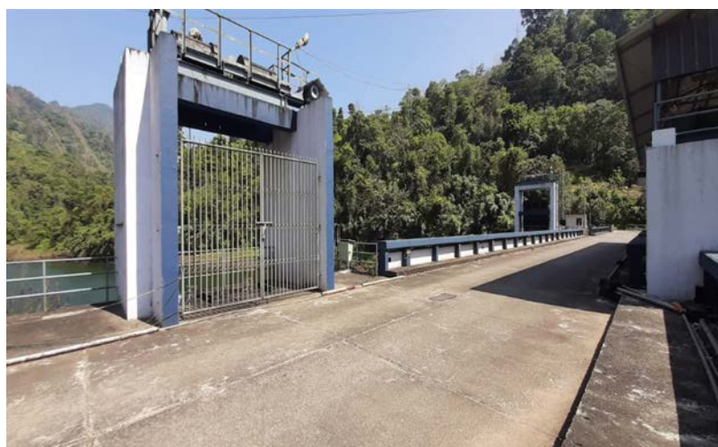
Fig 2.12a Sluice Gate Hoist Structure
