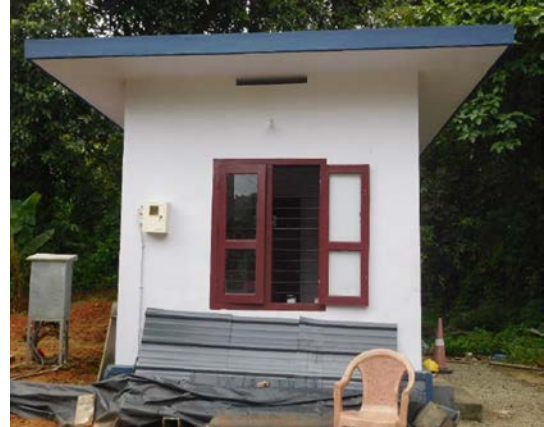
After construction of monitoring cabin
