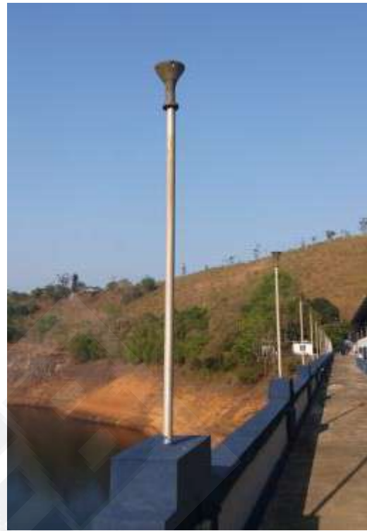
Dam Top Lantern–After
