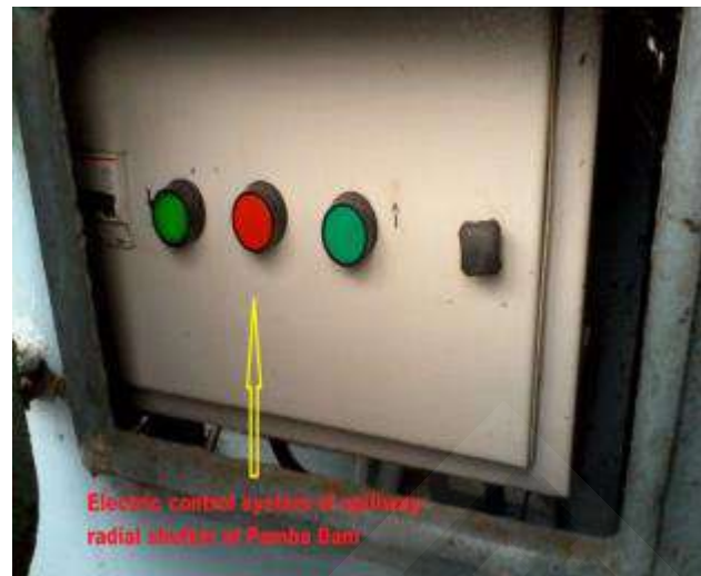
Fig 2.8 Electric Control system
