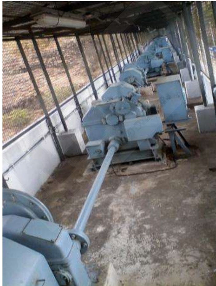
Fig 2.7 General View of Spillway Hoist Bridge
