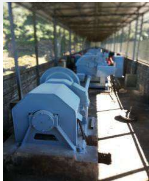
After - Special repair to Hoist mechanism
