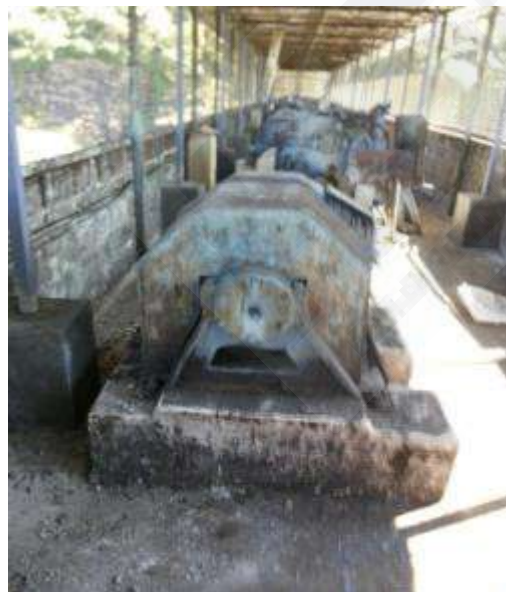
Before - Special repair to Hoist mechanism
