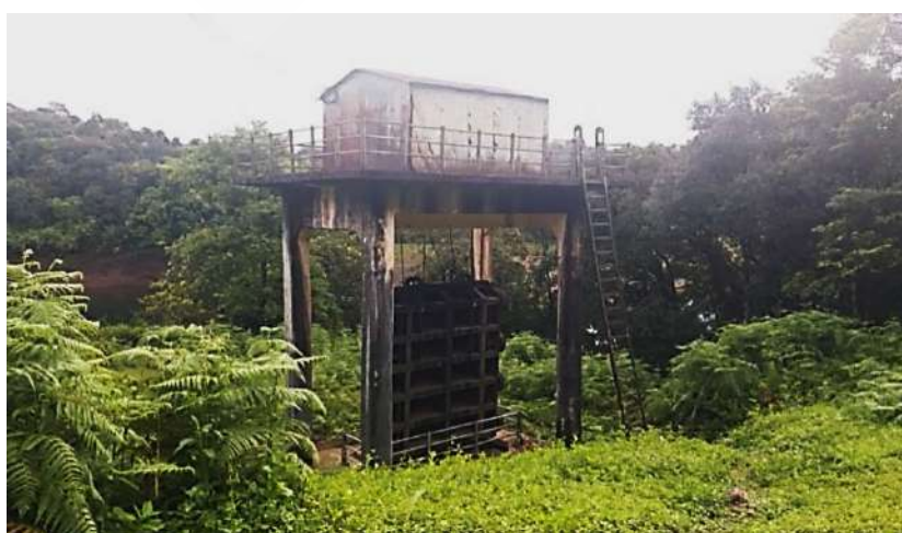
Fig 1.8 Intake Gate of Inter Connecting Tunnel Pamba-Kakki
