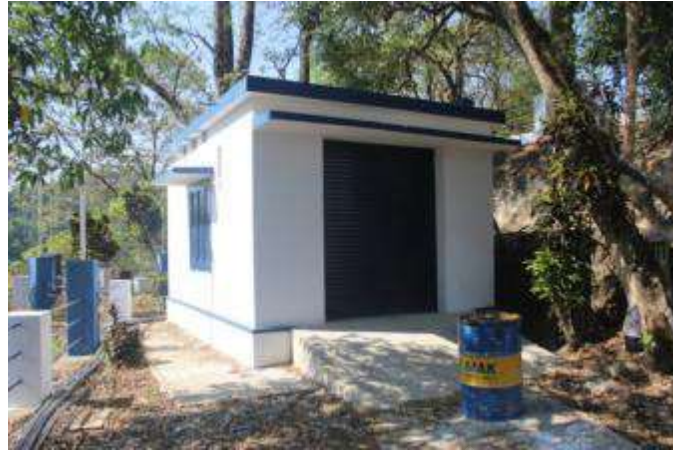
Construction of Generator room
