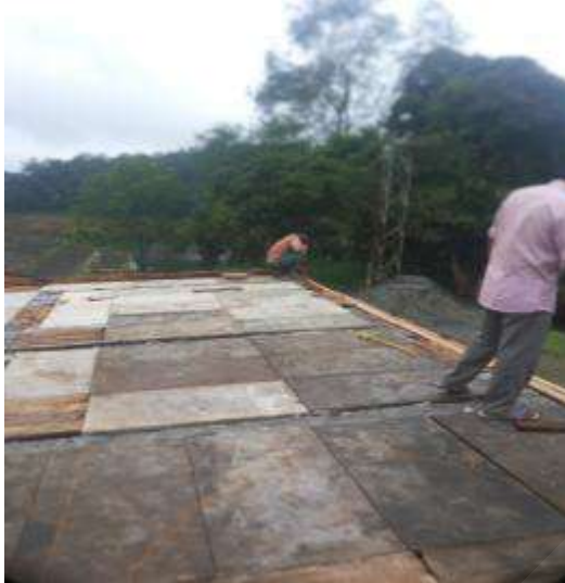
Monitoring cabin – Construction
