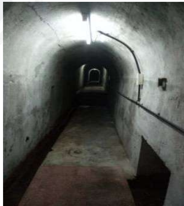
Reaming of drain holes
