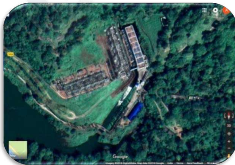
Fig 1.5 Sabarigiri Power House Google View
