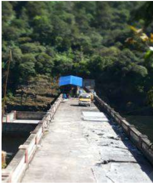
Before - Dam Top Wearing coat
