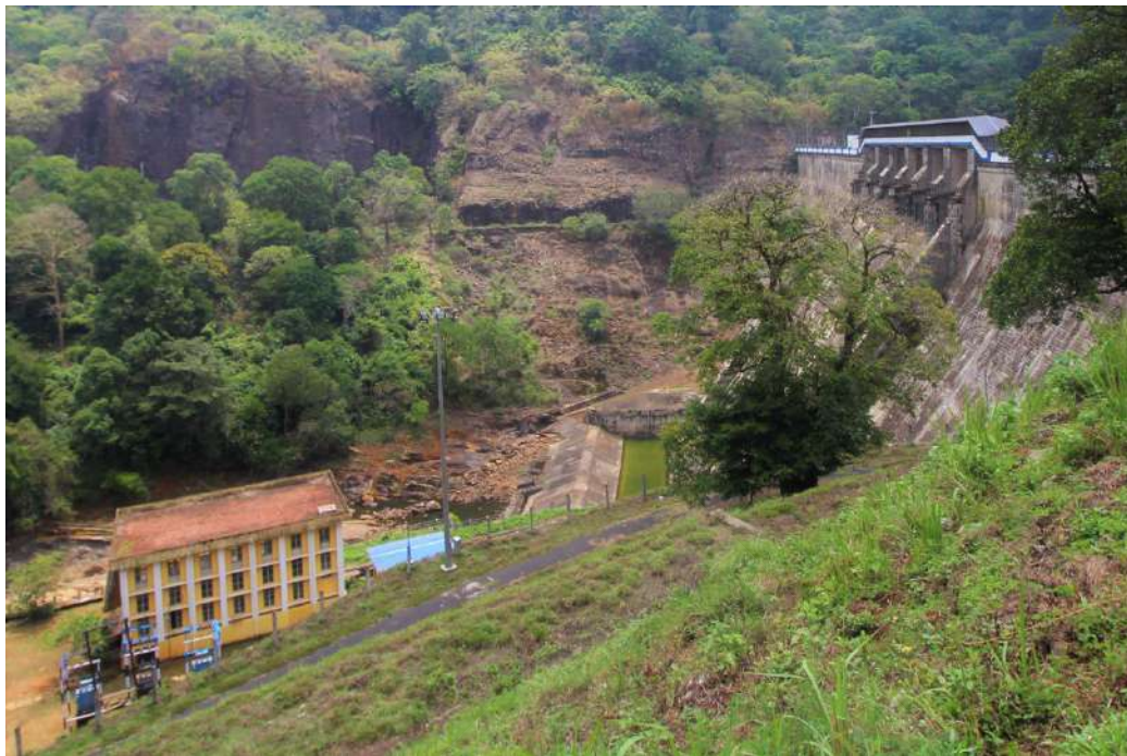
Fig 1.6 Pamba dam downstream with reverse pumping station
