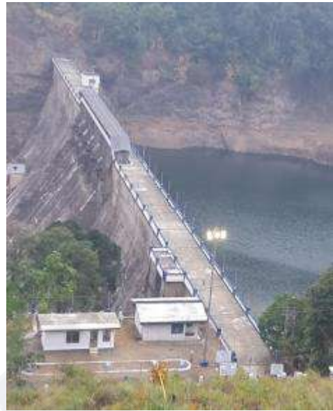
After - Dam Top Wearing coat
