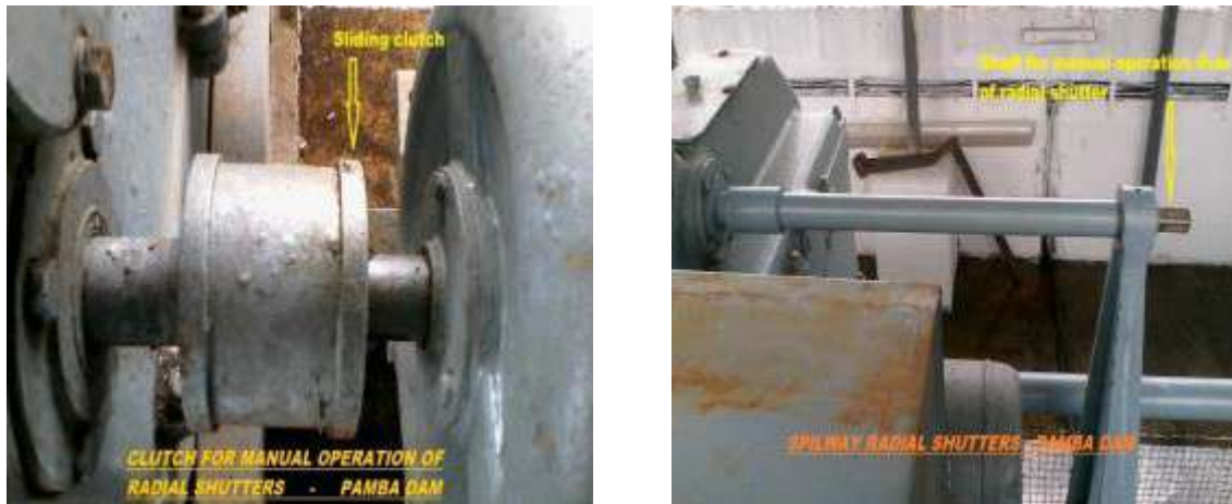
Fig 2.6 Radial Shutter Manual Operation
