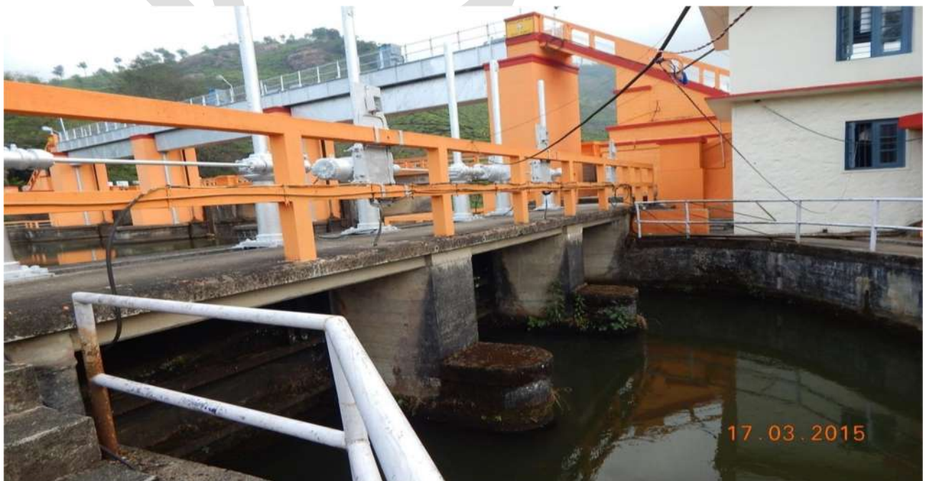
Fig 2.16 Intake Bridge and Hoisting Arrangements
