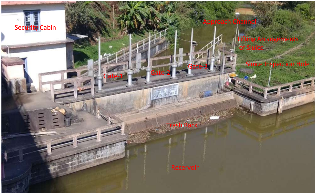
Fig 2.9 Main Intake Arrangements
