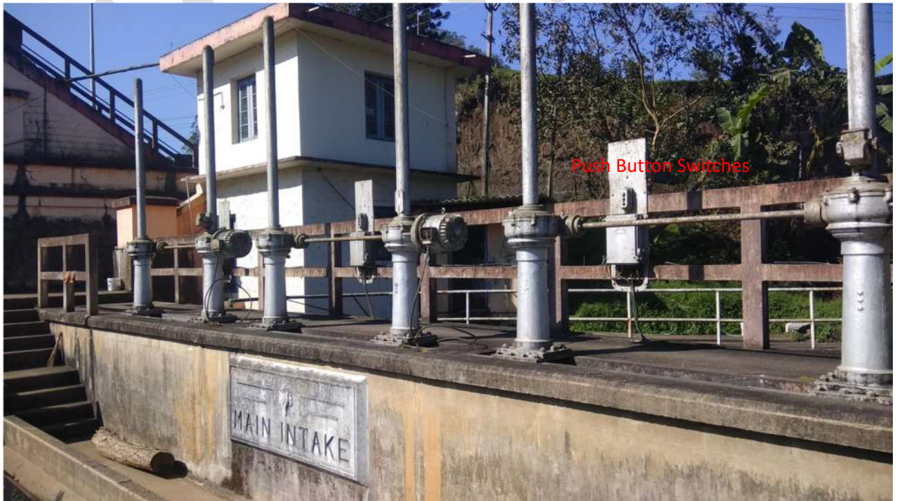
Fig 2.10 Main Intake Operating Arrangements
