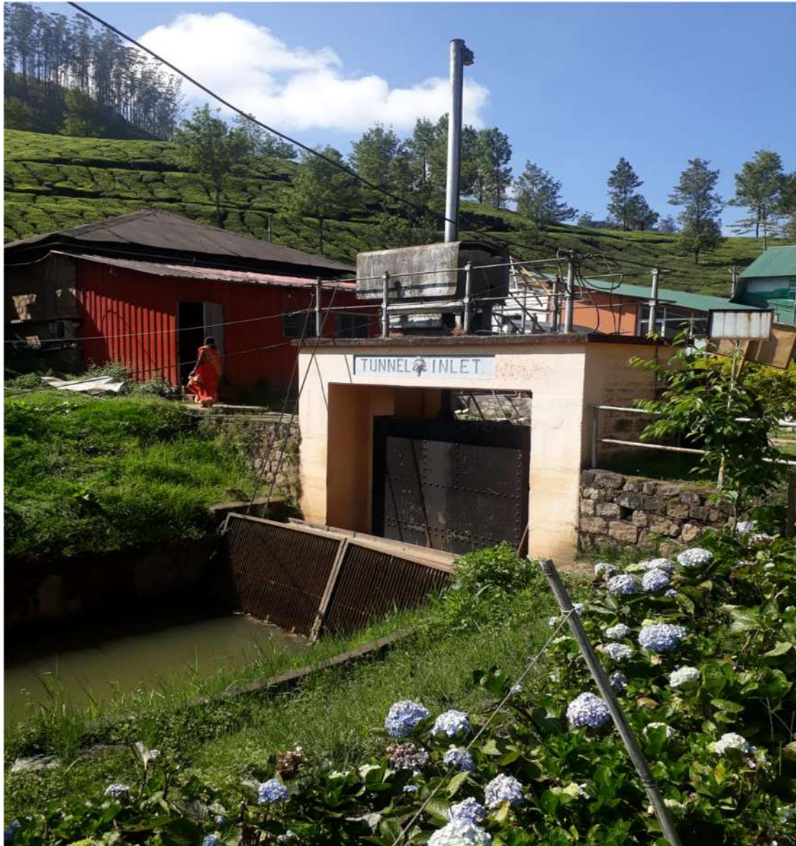
Fig 1.11 Photograph of Tunnel Inlet
