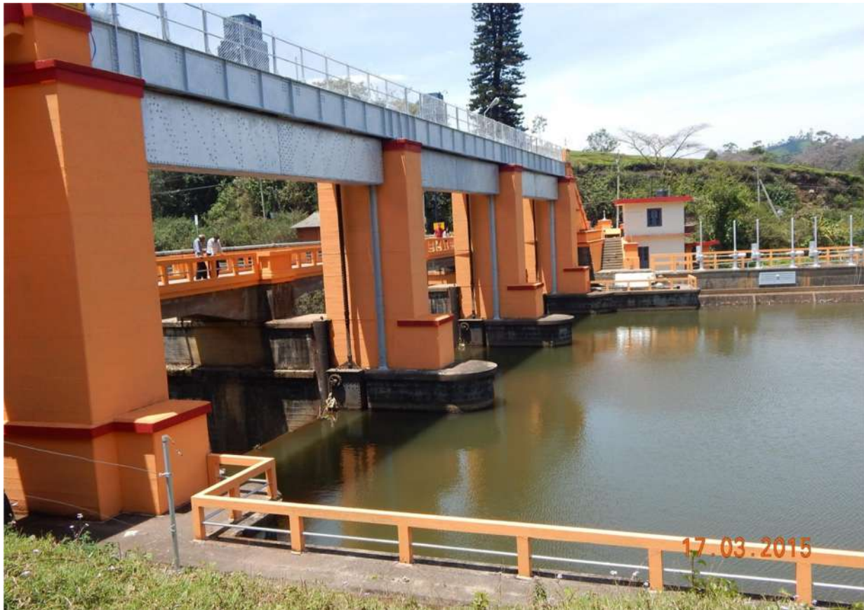
Fig 2.1 Spillway Arrangements at RA Head Works
