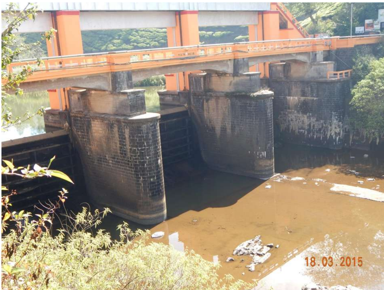
Fig 2.2 Spillway Arrangements at RA Head Works – View from Downstream
