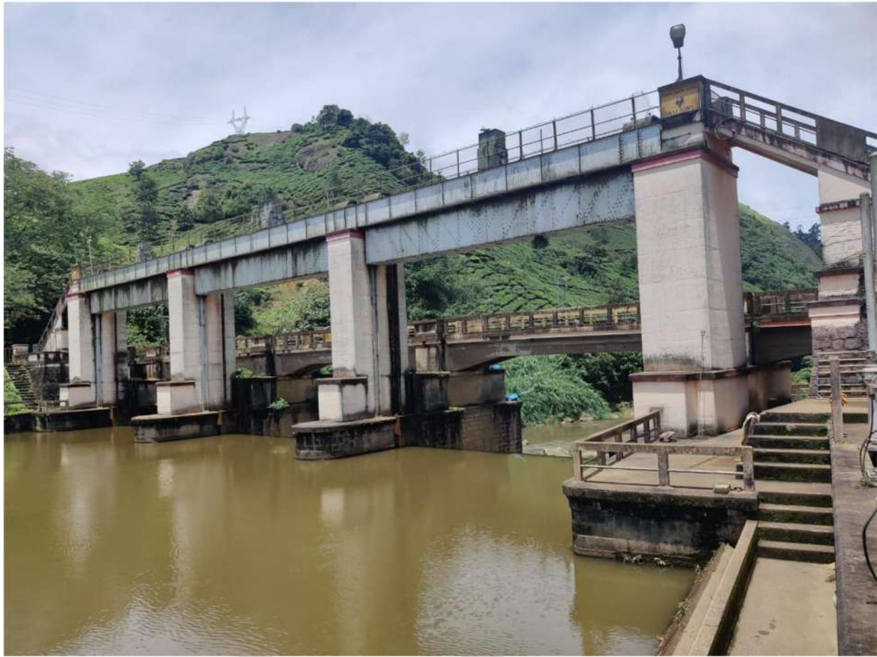
Fig 1.9 RA Head Works - Photograph
