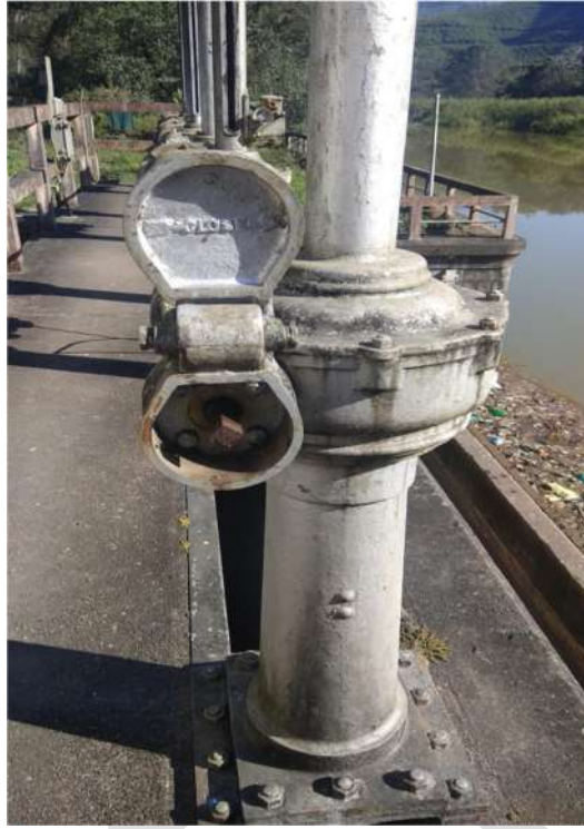
Fig 2.11 Main Intake – Hand Operating Arrangements
