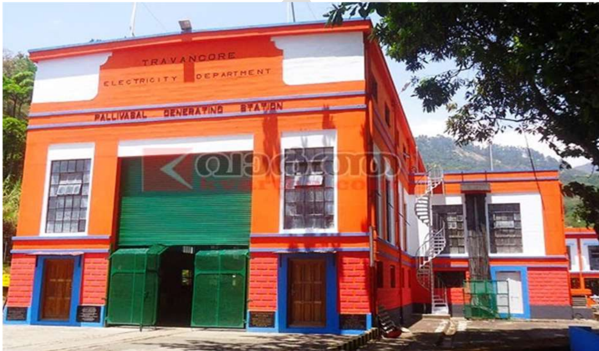
Fig 1.16 Pallivasal Power House
