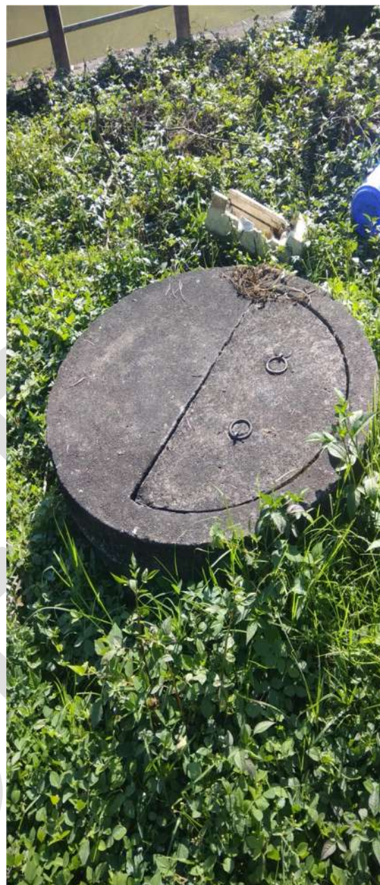
Fig 2.8 Sluice Inspection Chamber
