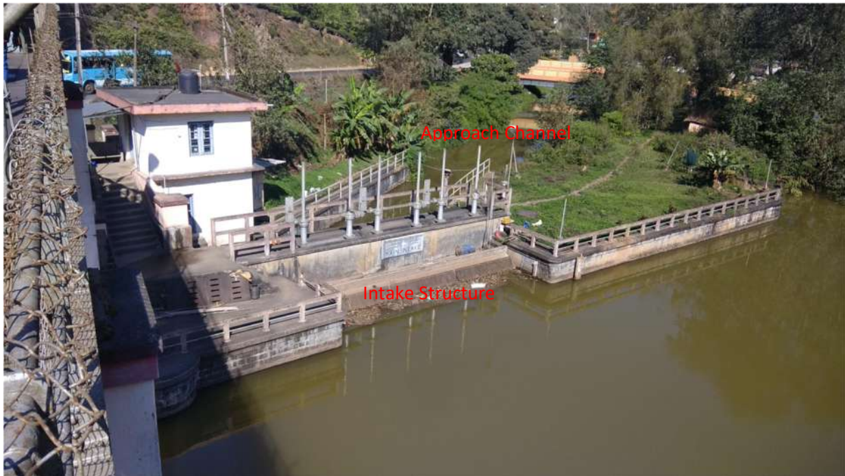
Fig 1.10 RA Head Works- Photographs of Main Intake and Approach Channel
