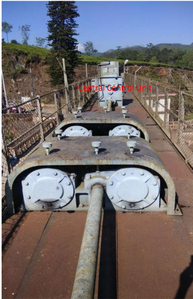
Fig 2.4 Hoisting Arrangements of Main Gate
