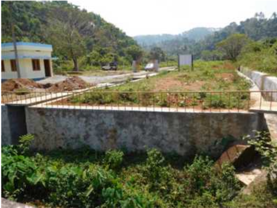
Fig 6.14 Construction of Retaining Wall and deep trench near Intake site.
