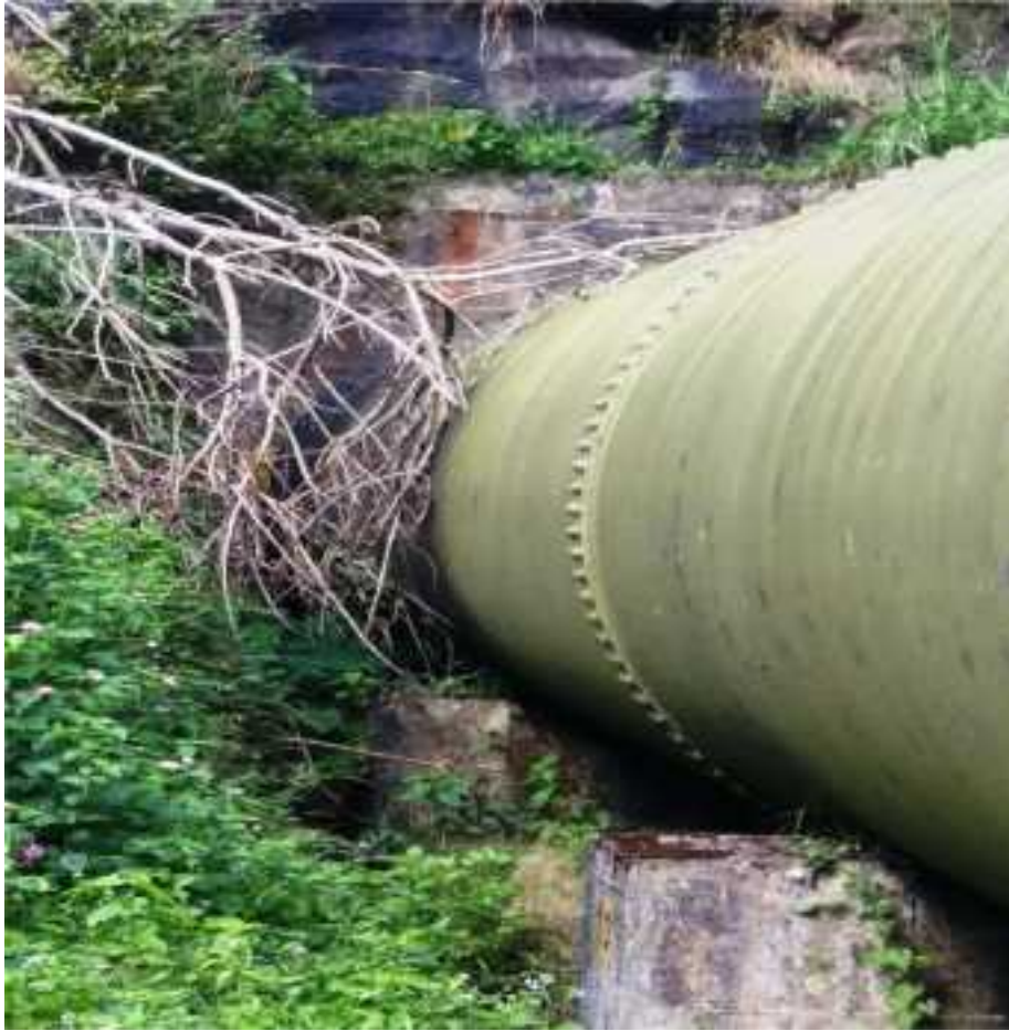
Fig 1.16 – LPP coming out from Tunnel 1 - Close up view
