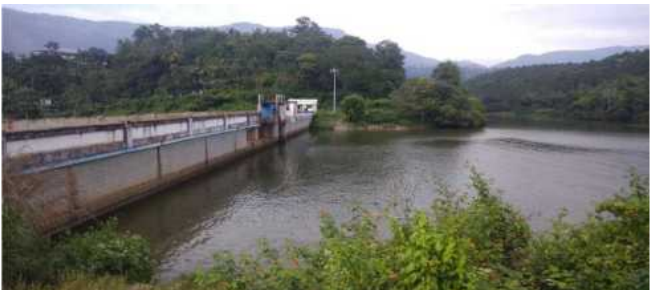
Fig 1.13 – Sengulam Dam - an Upstream View
