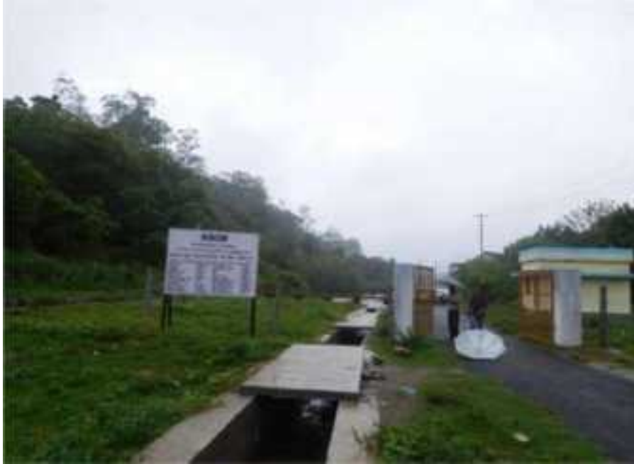
Fig 6.10 View of rehabilitation works at Intake area
