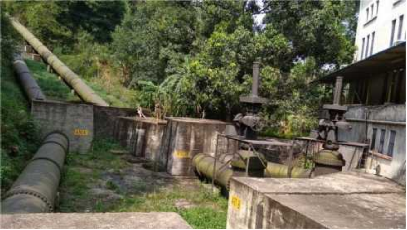
Fig 1.23 – HPPs approaching Power House Building
