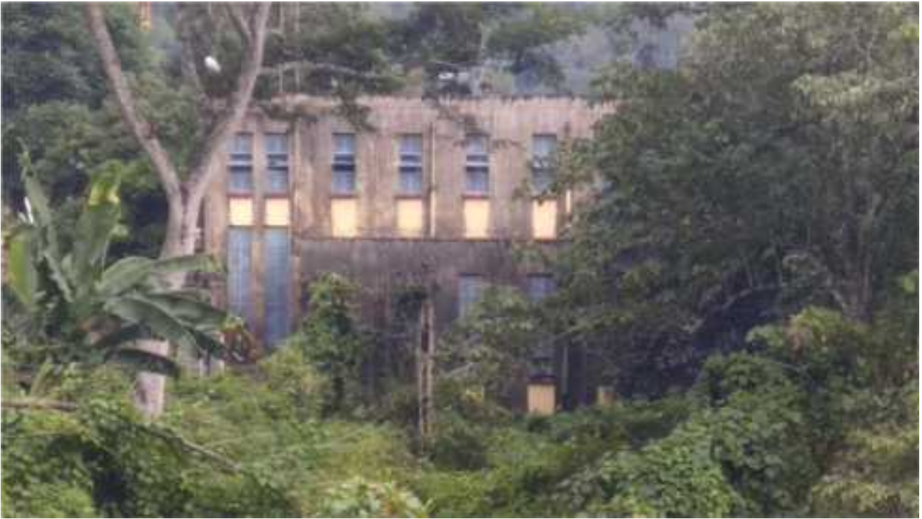
Fig 1.11 – Pump House at Pallivasal to pump the water to Tunnel No.1
