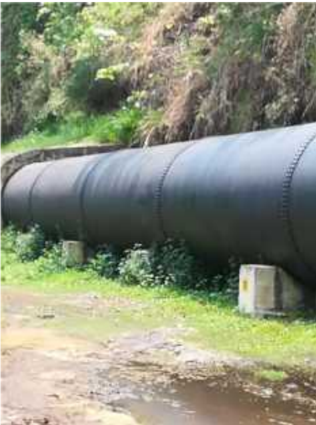
Fig 1.18 – LPP Entering to Surge Shaft Hill
