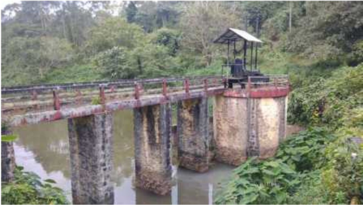
Fig 6.6 Photograph showing Intake
