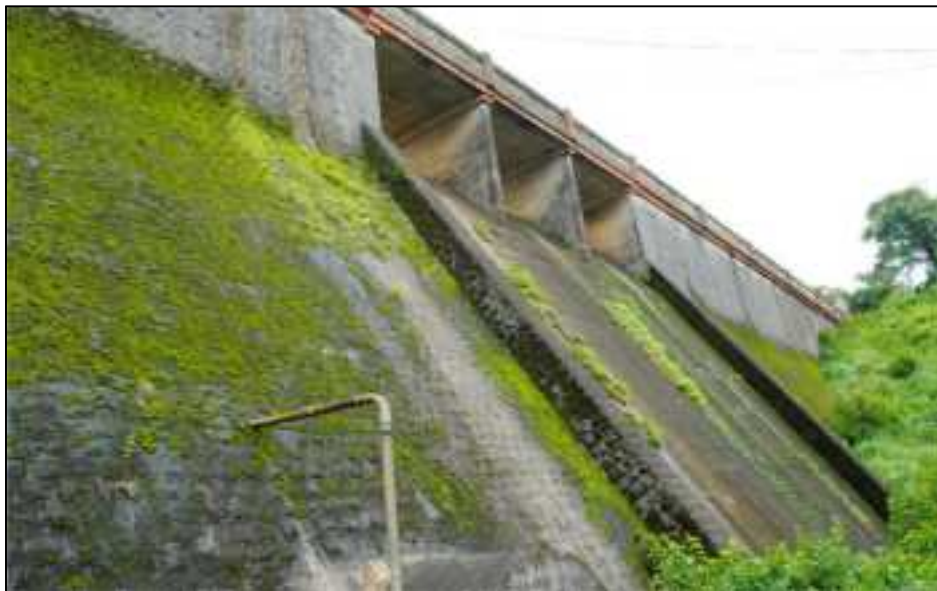
Fig 2.1 Photograph Showing un-gated Spillway Arrangements of Sengulam Dam
