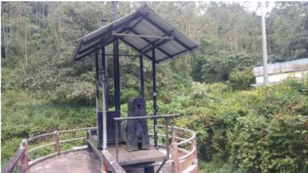
Fig 6.7 Photograph showing Roofing works of Intake
