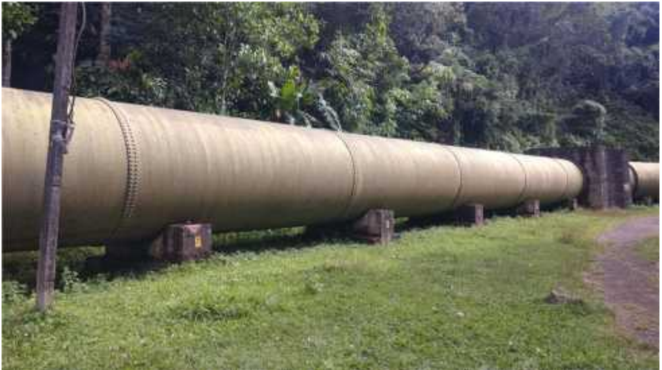
Fig 1.17 – Low Pressure Pipe
