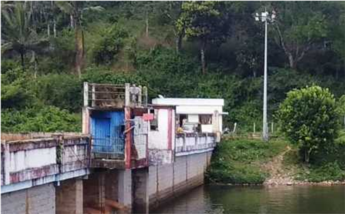
Fig 6.1 Photograph showing Newly Constructed Security cabin at Right Bank of Dam
