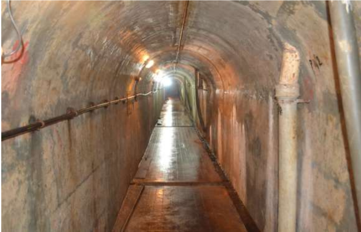
Fig 2.9 Drainage and inspection gallery
