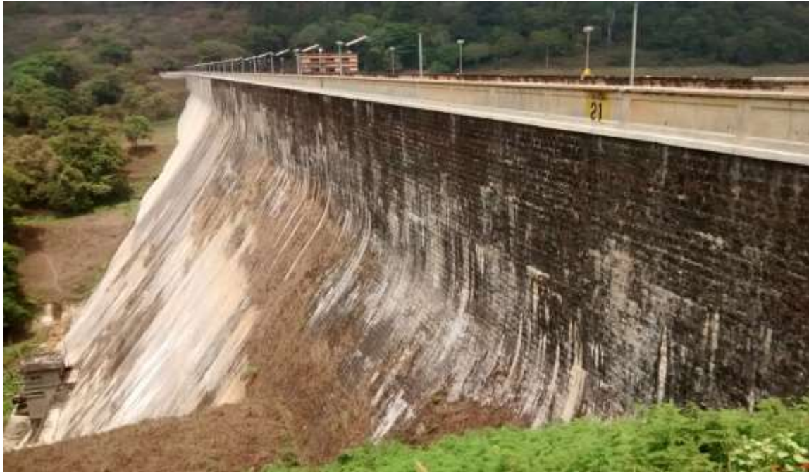
Fig 6.7 D/s face of main dam before pressure washing
