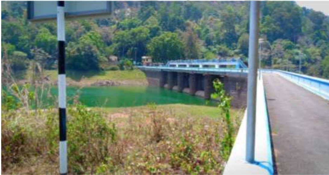
Fig 1.4 Upstream view of the Flanking Dam
