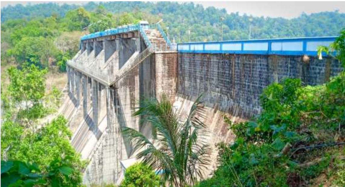
Fig 2.4 Spillway of Sholayar Flanking Dam
