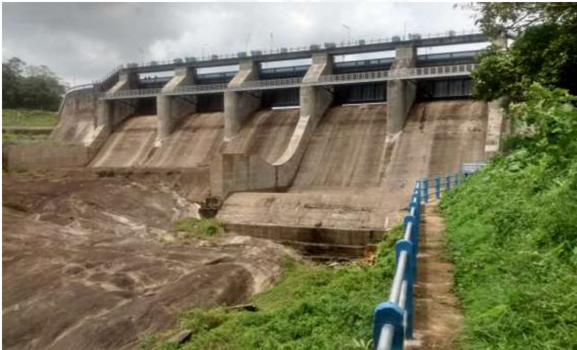
Fig 2.2 Downstream view of spillway
