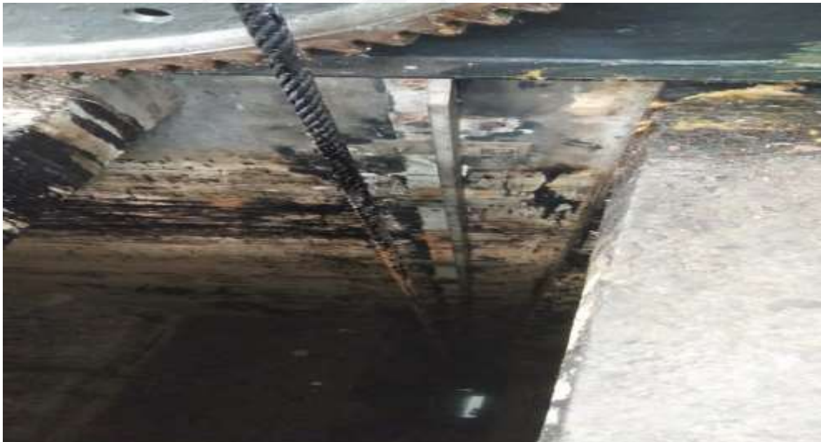
Fig 6.4 Emergency gate guide after replacement
