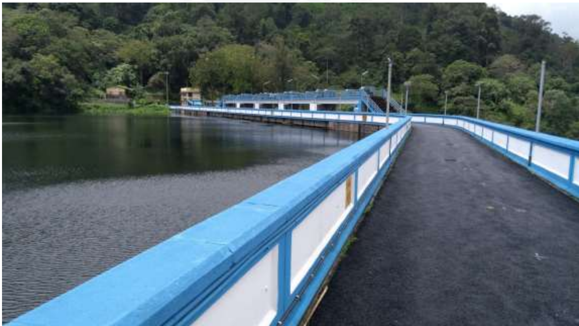
Fig 6.12 Flanking dam – road work
