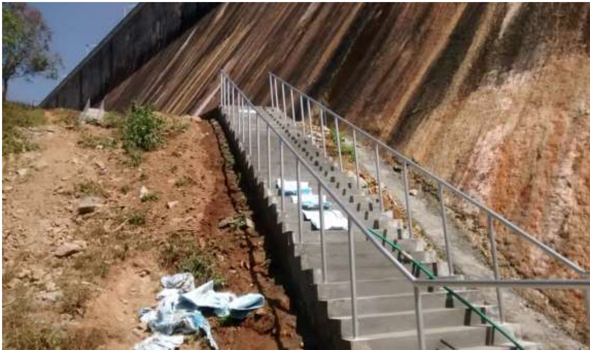
Fig 6.9 Access steps constructed
