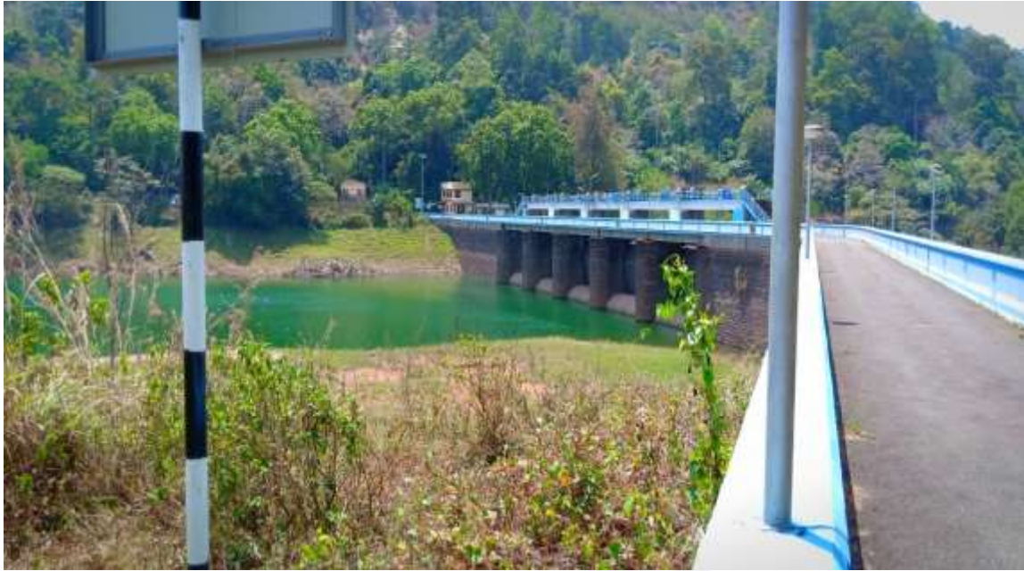
Fig 2.3 Sholayar Flanking Dam u/s view
