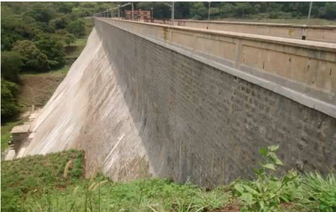
Fig 6.8 D/s face of main dam after pressure washing
