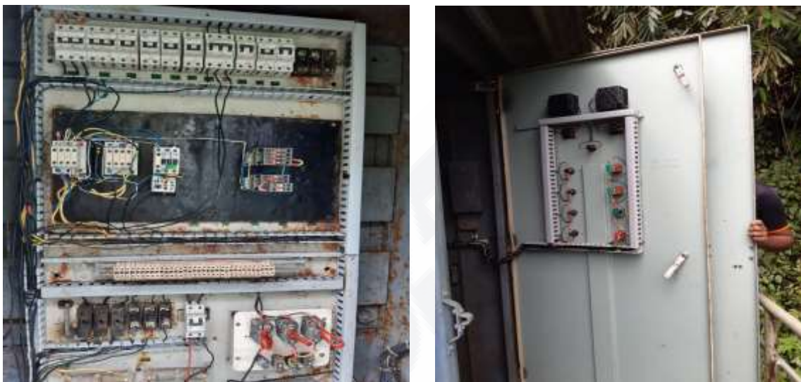
Fig 2 Control panel of intake gate
