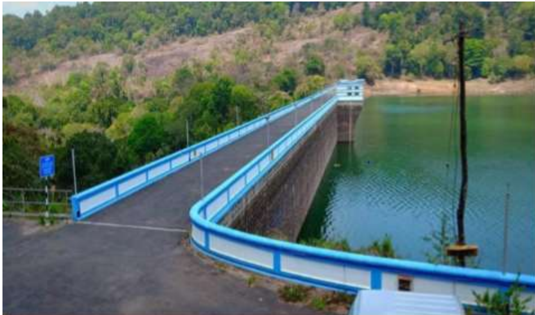
Fig 1.5 View of Main Dam
