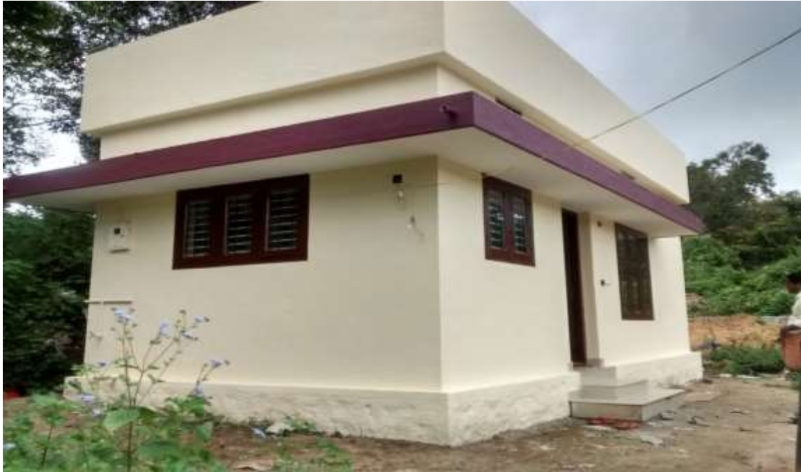
Fig 6.11 Security guard room constructed
