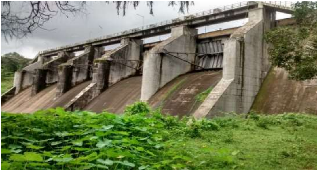
Fig 6.1 Flanking Dam before construction of catwalk
