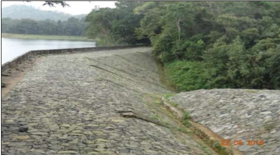
Fig 1.6 View of Saddle Dam
