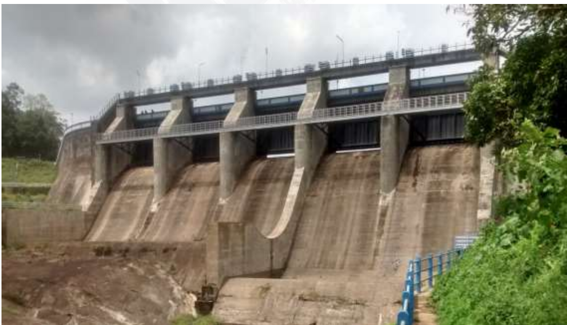
Fig 6.2 Flanking Dam after construction of catwalk
