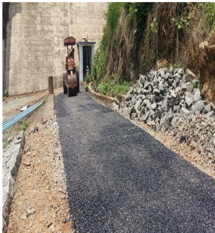
After - Improvements to road to Veluthode dam
