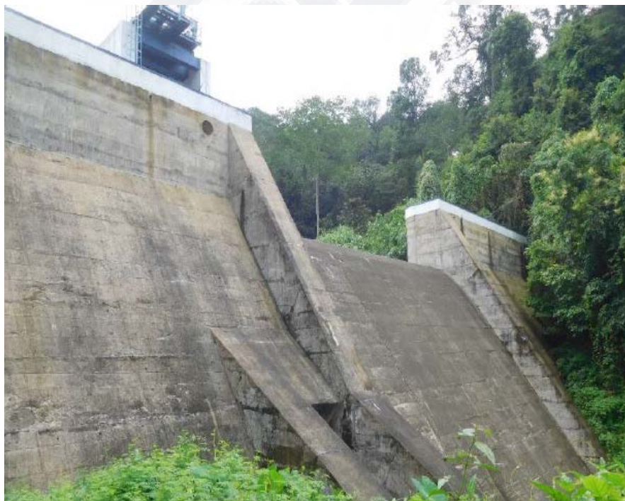
Fig 1.5a Downstream Elevation of Veluthode Dam
