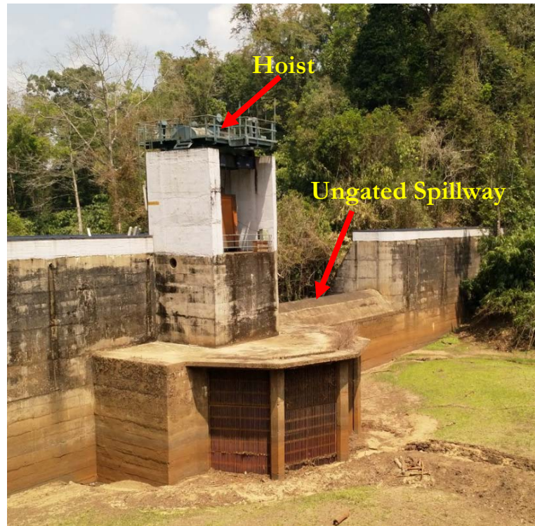
Fig 2.4 Upstream view of Veluthode dam with scour sluice
