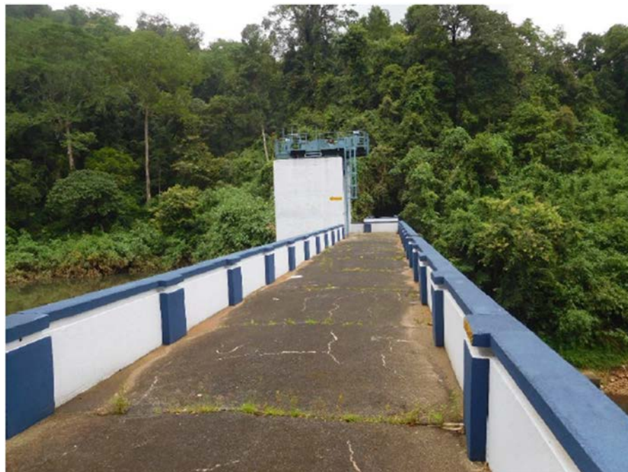
After - Painting works of Veluthode dam
