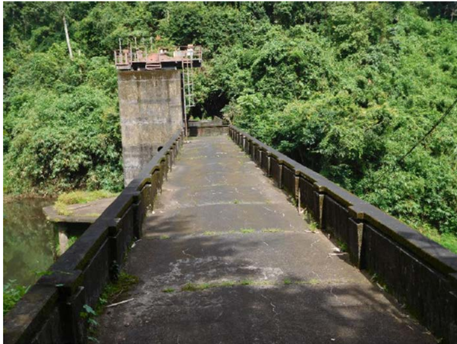
Before - Painting works of Veluthode dam
