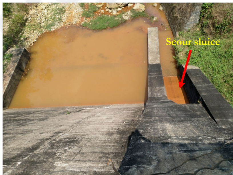
Fig 2.5 Downstream view of Veluthode dam
