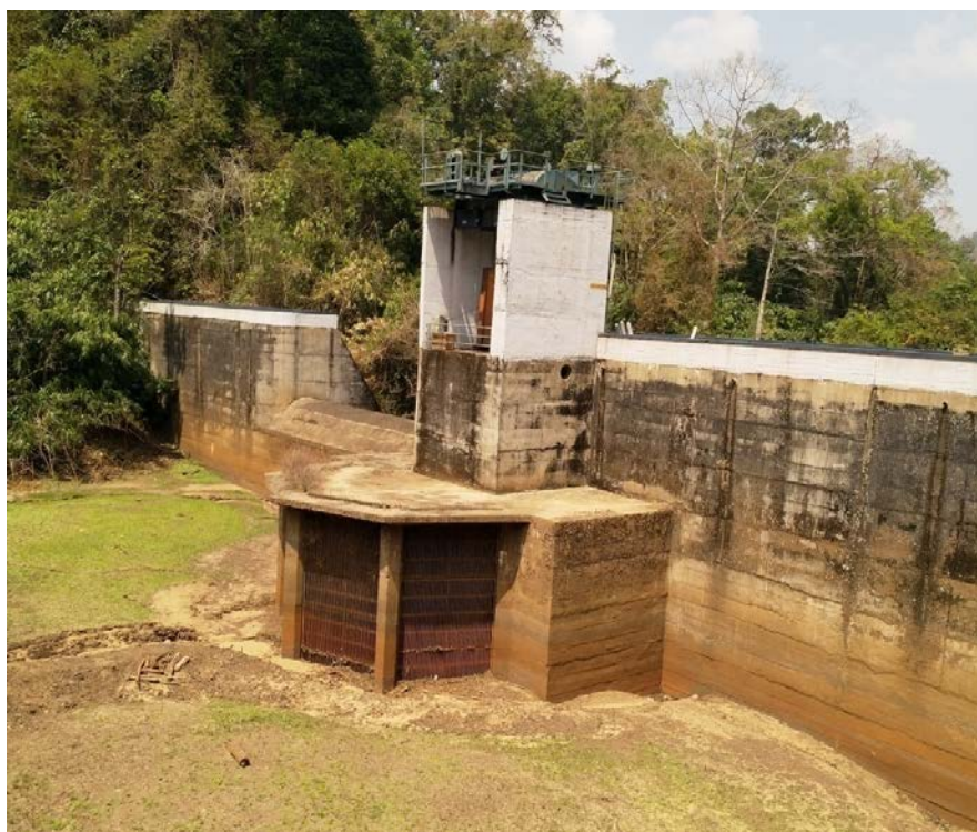
Fig 1.5b Upstream Elevation of Veluthode Dam with ungated Spillway and trash rack of scour sluice
