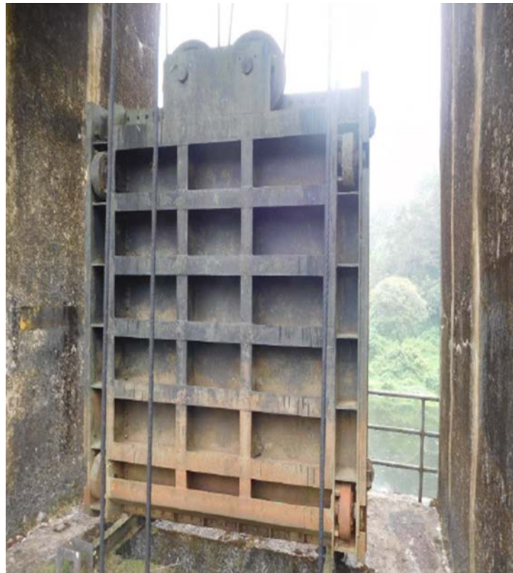
Before - Painting of gate at Veluthode dam
