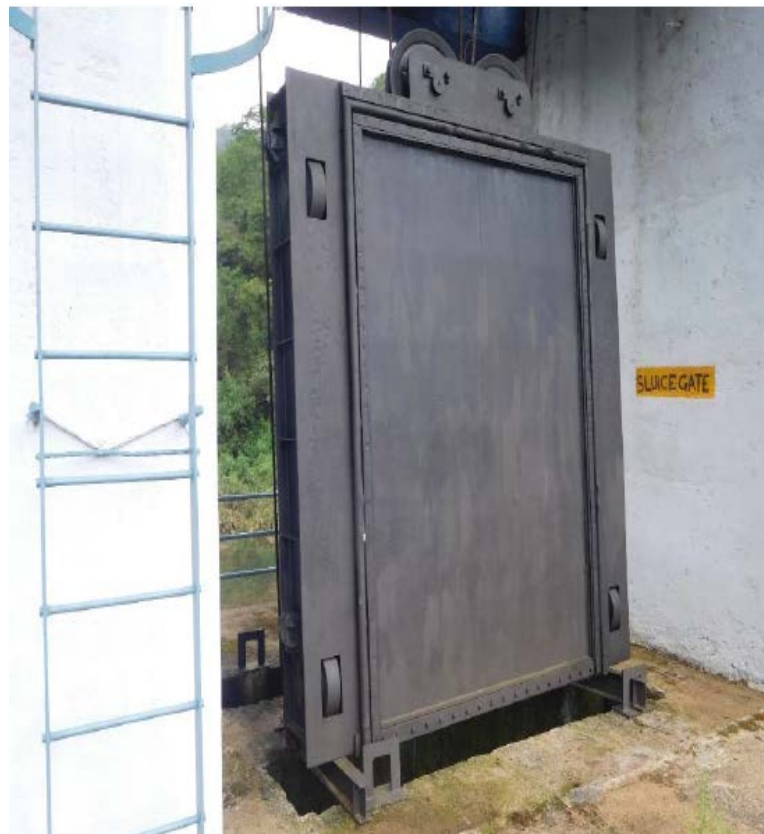
Fig 2.6 Sluice gate at Veluthode dam
