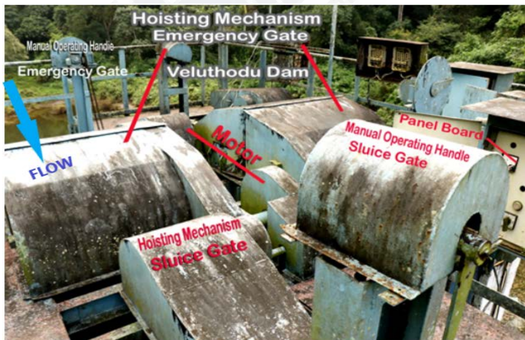
Fig 2.8b Emergency gates hoisting mechanism
