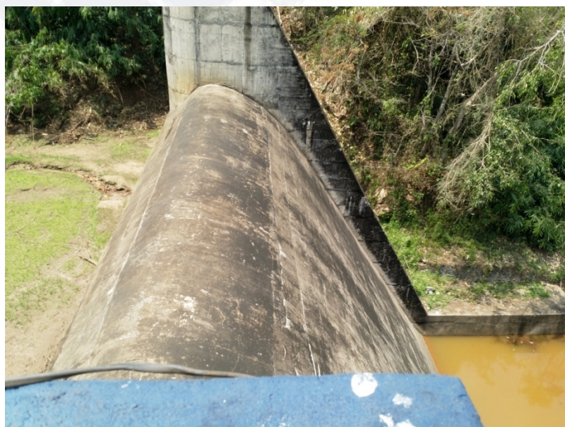
Fig 2.2 Spillway of Veluthode dam
