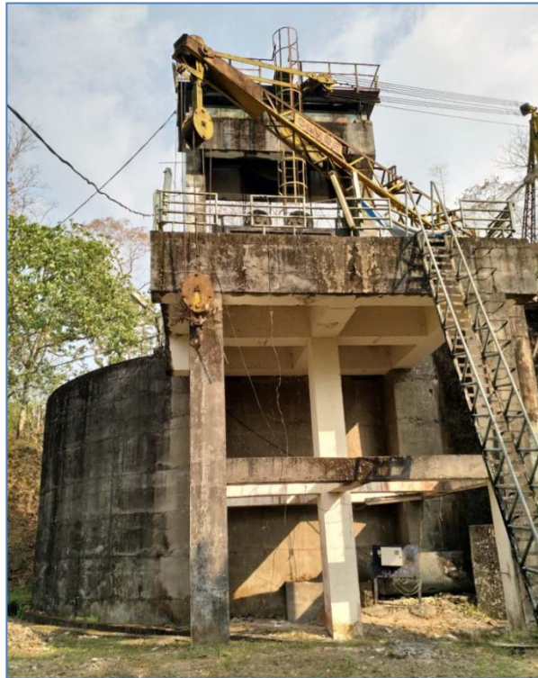
Fig 2.11 Surge shaft gallery
