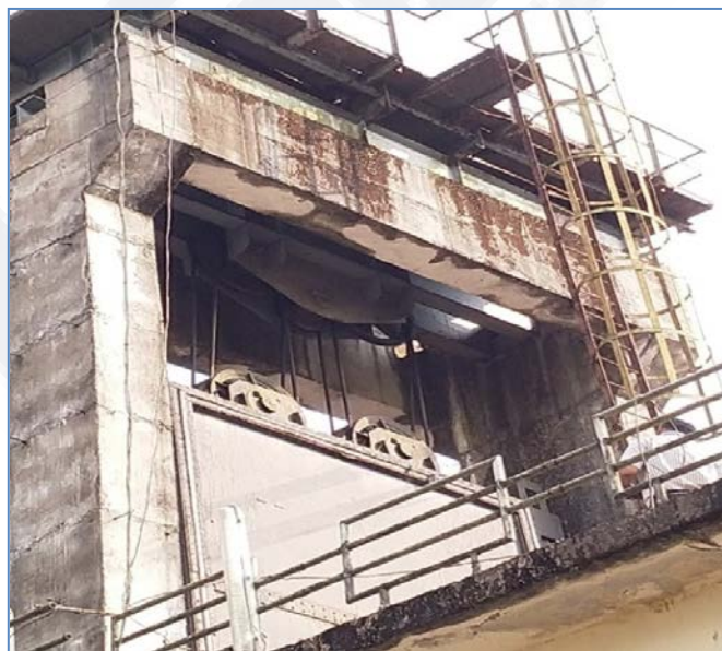
Fig 2.12 Vertical lift gate of the surge shaft
