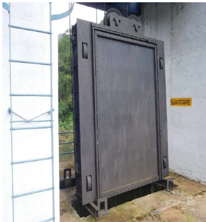
After - Painting of gate at Veluthode dam
