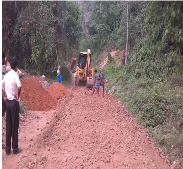
During - Improvements to road to Veluthode dam gallery
