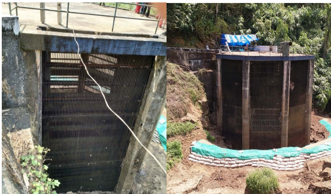
Fig 2.10 Vertical Intake Shaft
