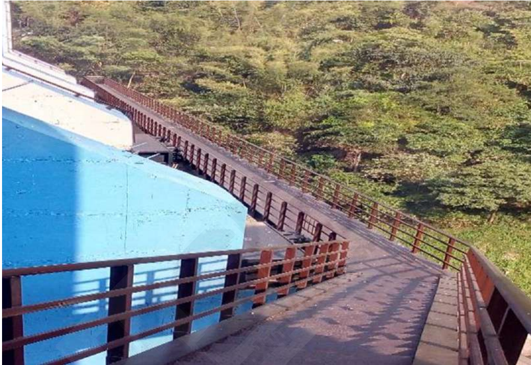
Fig 6.2 Catwalk connecting Radial gate trunnions
