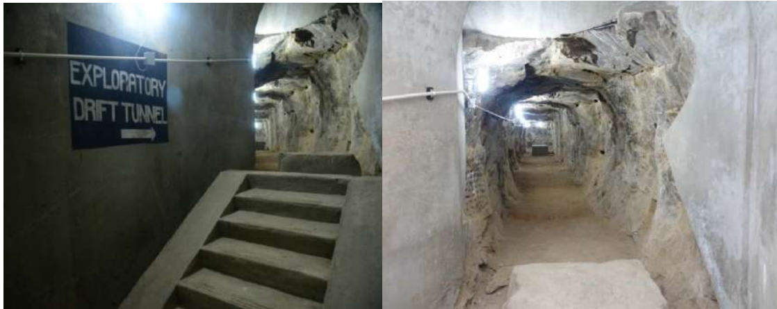
Fig 1.16 Exploratory drift tunnel at El.1925 Right bank
