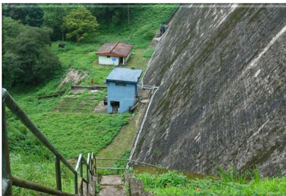
Fig 1.31 Disperser Valve House
