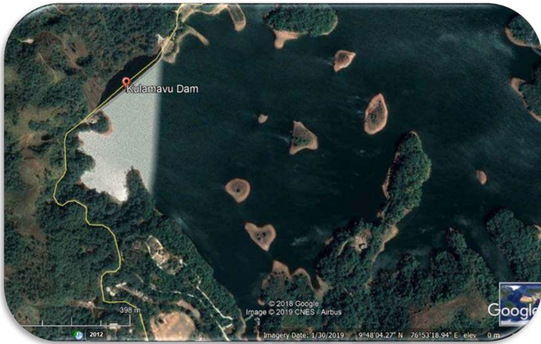
Fig 1.28 Google view of the Kulamavu Dam
