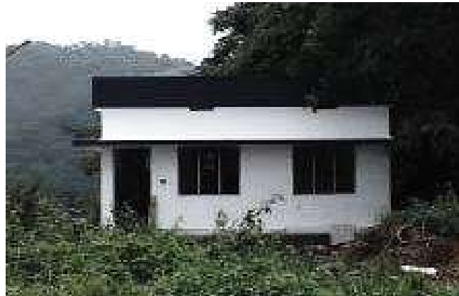
Security cabin at Idukki dam bottom
