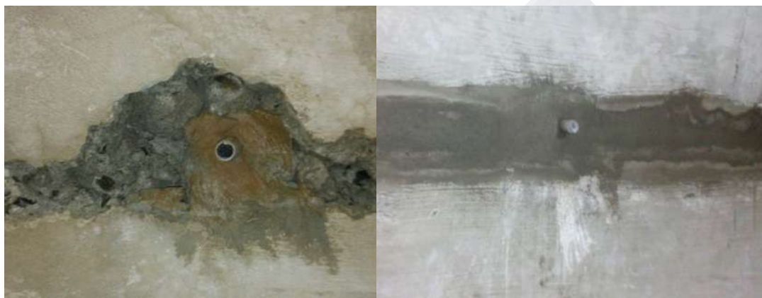
Crack Treatment in Gallery at El.2300 ft (before & After)
