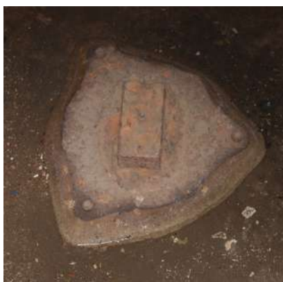
Fig 5.8 Anchoring point of pendulum at dam top
