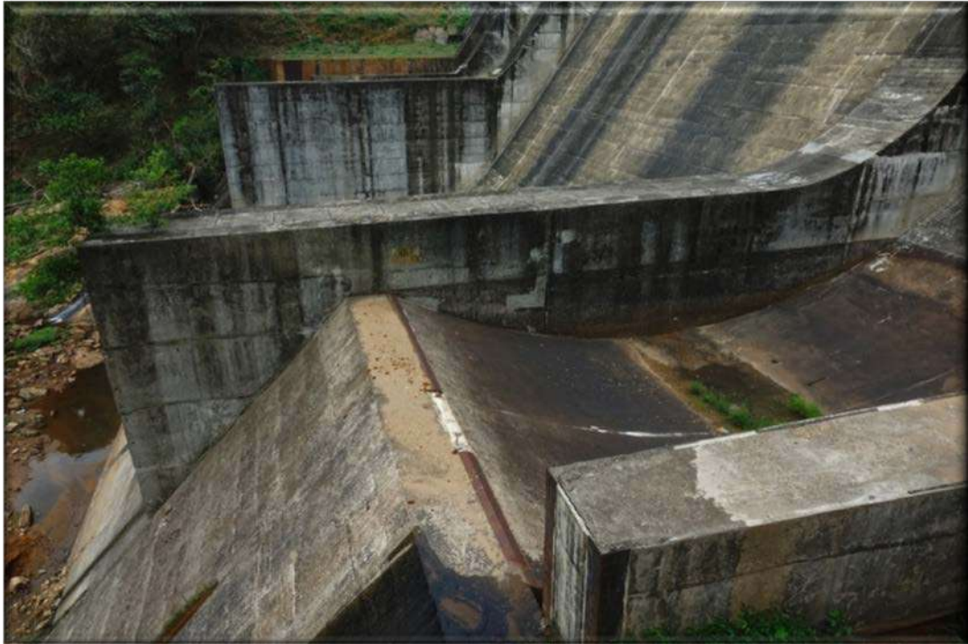
Fig 2.9 View of Spillway bucket from Left bank
