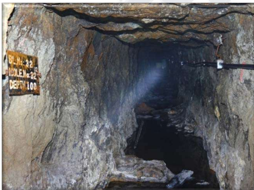
Fig 1.25 View of Drift tunnel at Cheruthoni dam
