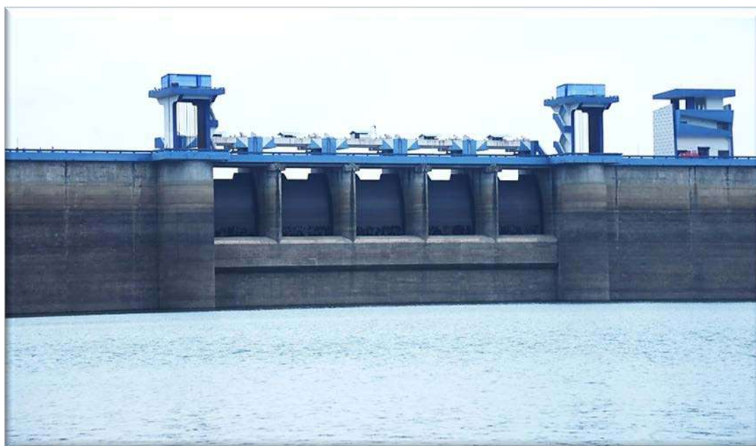
Fig 2.2b Upstream Elevation of Spillway
