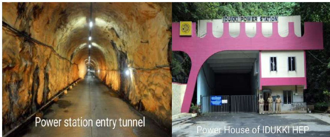
Fig 1.35 IHEP Power House
