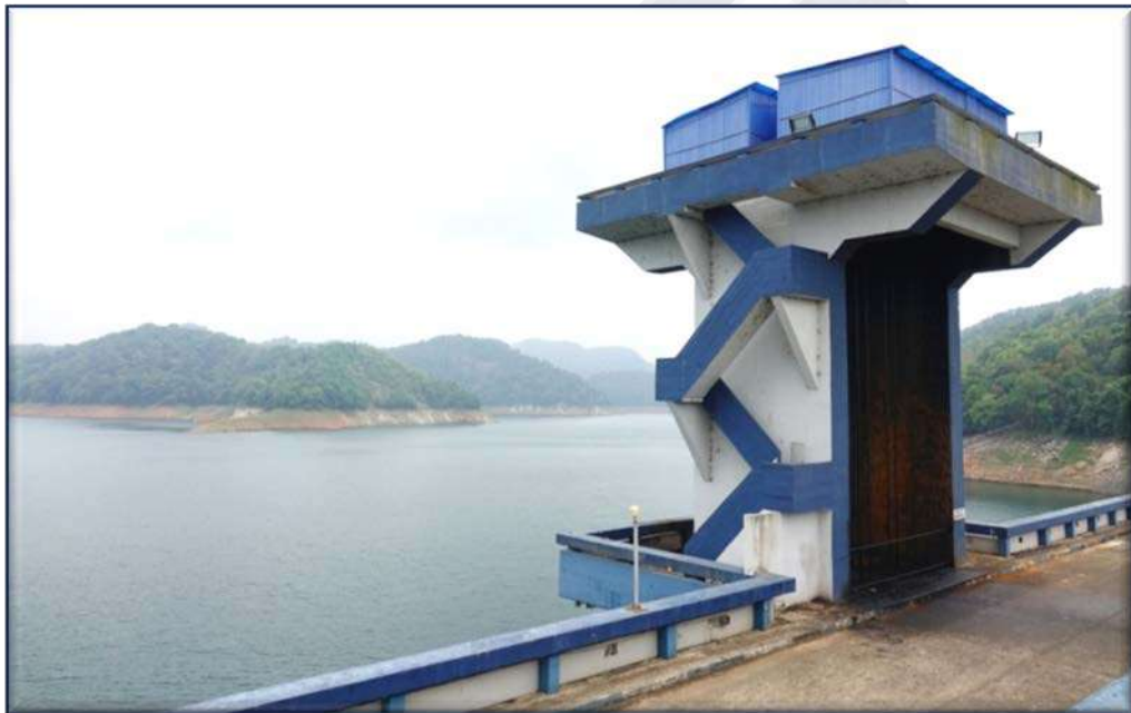
Fig 2.15 Hoist Bridge for sluice gate operation (Service and Emergency Gates)
