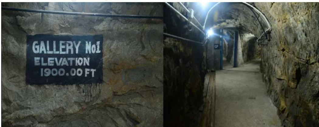
Fig 1.14c Foundation gallery at El.1900'
