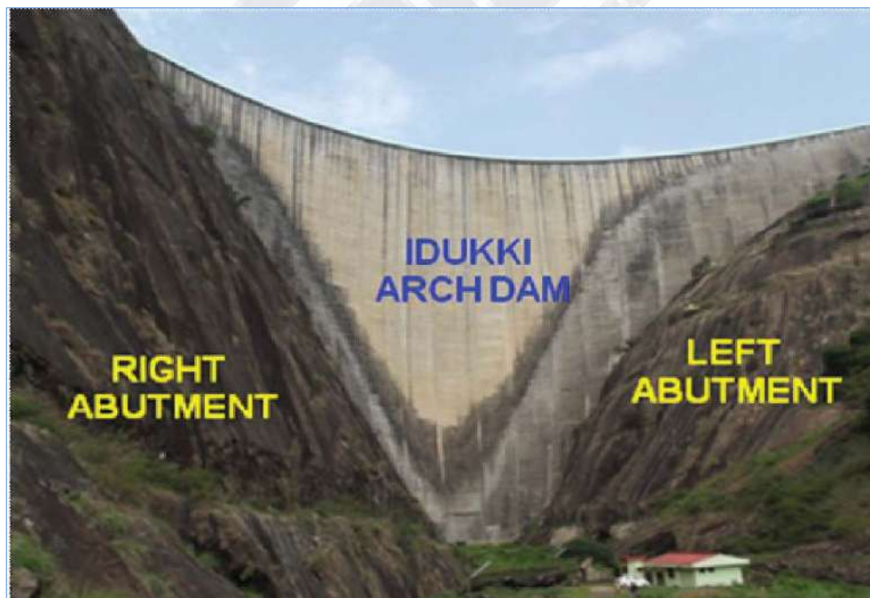
Fig 1.11b View of Idukki dam downstream
