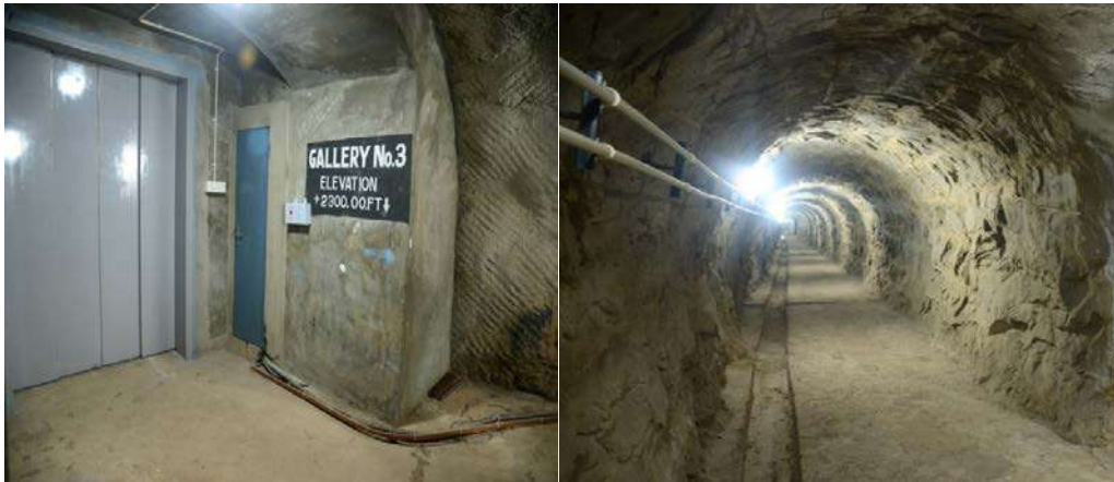
Fig 1.14a Inspection gallery at El. 2300'
