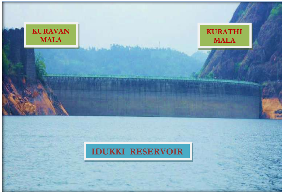
Fig 1.11a View of Idukki dam from upstream of reservoir
