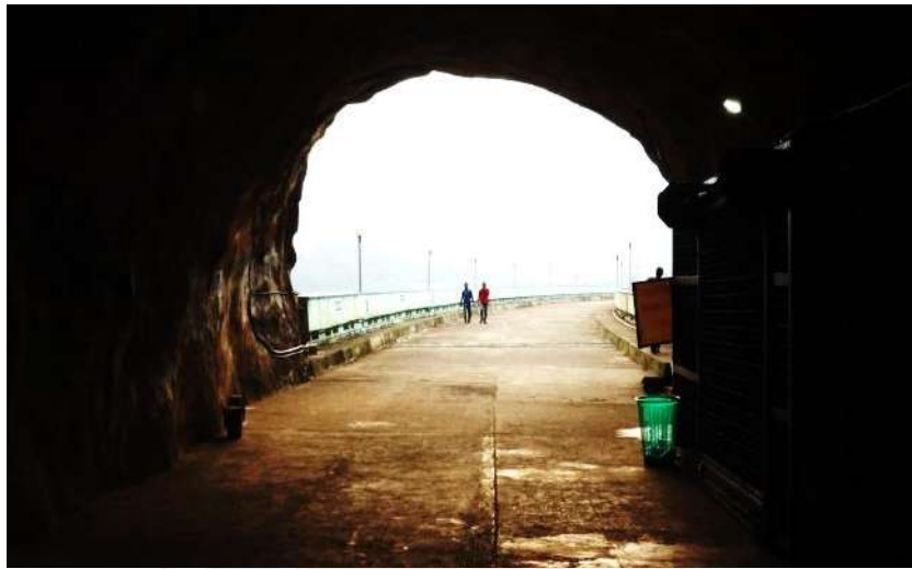
Fig 1.15a View of Idukki dam from road tunnel at right bank
