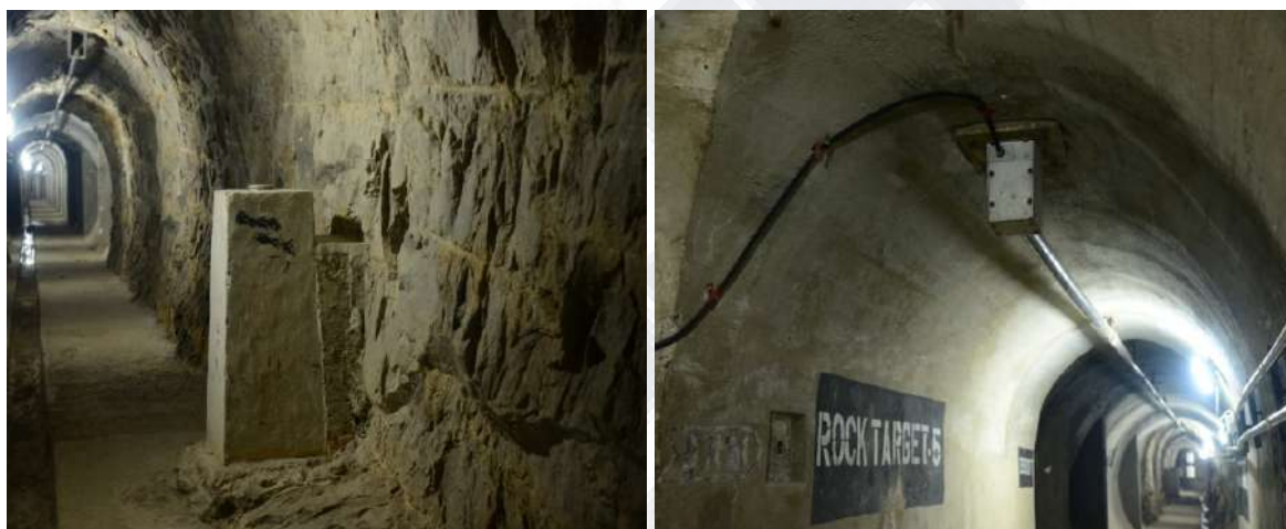
Fig 5.4 View of rock target station at galleries
