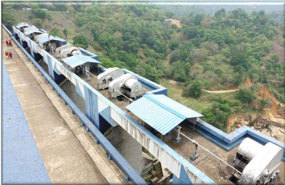
Fig 2.7 View of Spillway Gate Operation Bridge of Cheruthoni dam (Units #1 to #5 Left to Right)
