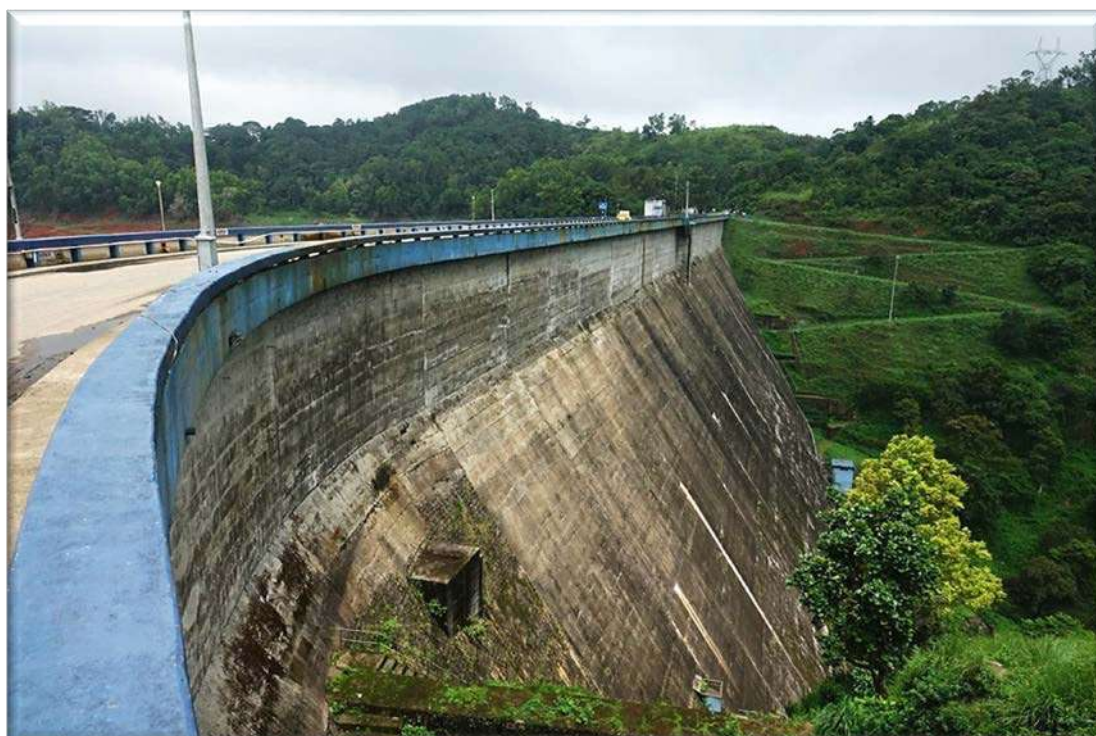
Fig 1.30 Kulamavu Dam Downstream view
