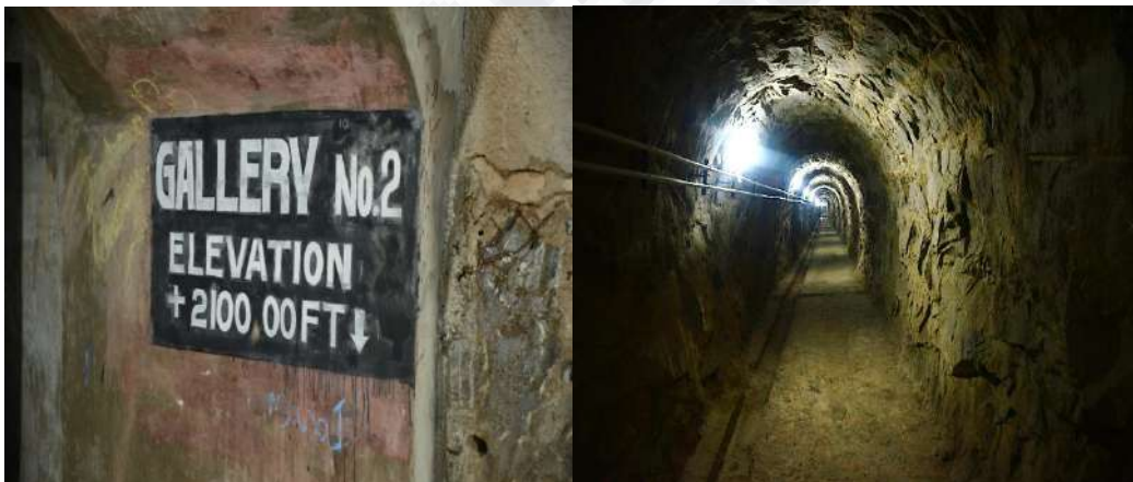
Fig 1.14b Inspection gallery at El. 2100'
