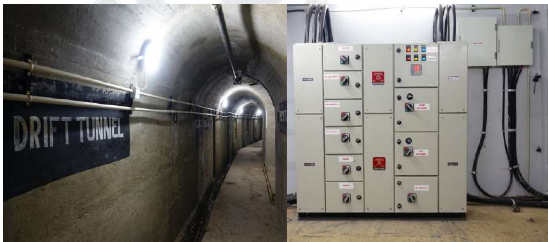
Rewiring of Idukki arch dam Gallery
