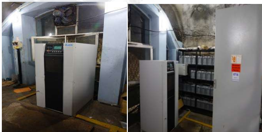
Modernization of Elevator with ARD (power backup) and control systems
