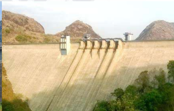
Pressure washing (after)
