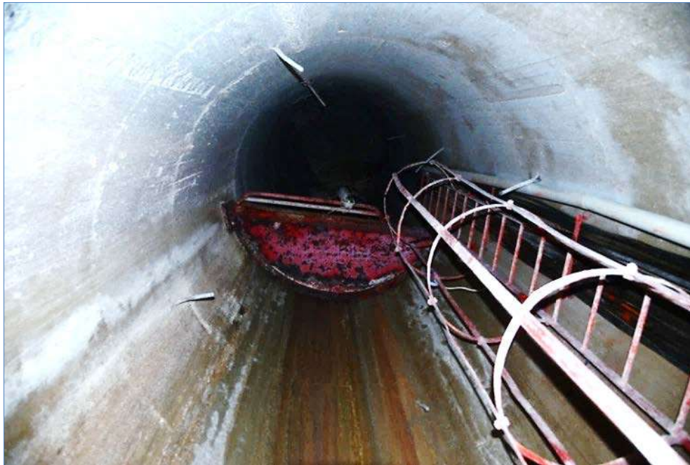
Fig 1.18a Vertical shaft at right bank
