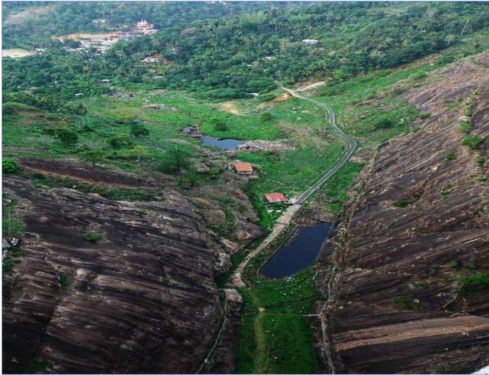
Fig 1.12a View of Idukki dam d/s bottom from central block – 01
