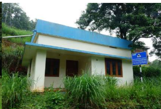
Guard Room at Intake control shaft
