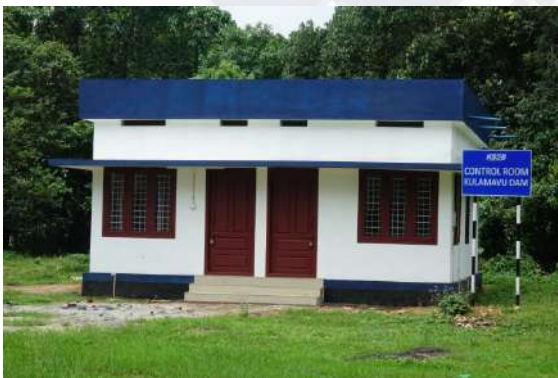
Control room for Kulamavu dam
