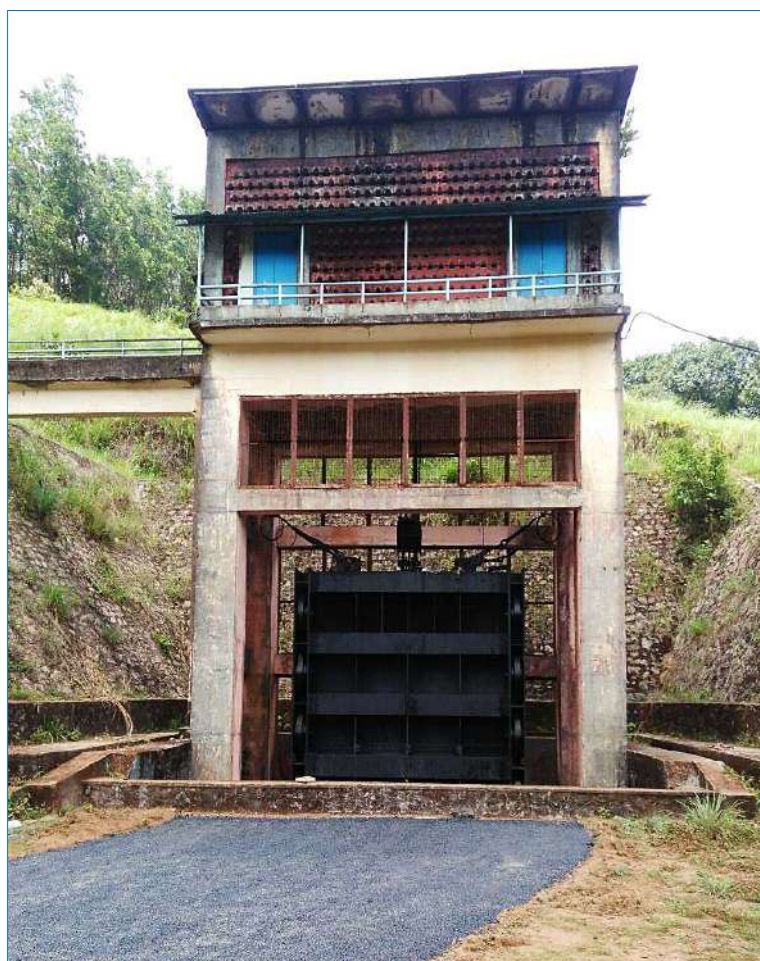
Fig 2.21a Intake gate and Hoist
