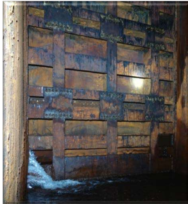
Fig1.23 Sluice gate downstream side view from manhole
