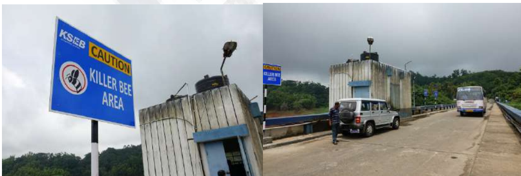
Emergency gate hoisting machine room
