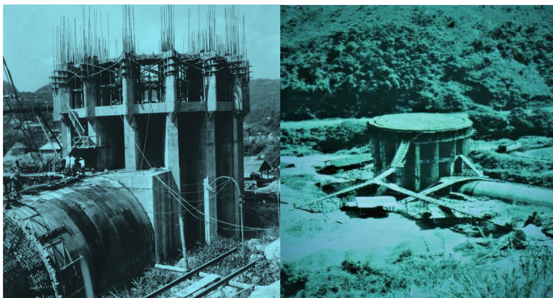
Fig 2.19 Morning Glory Intake during and after Construction
