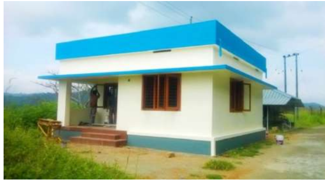
Security Guard Rooms
