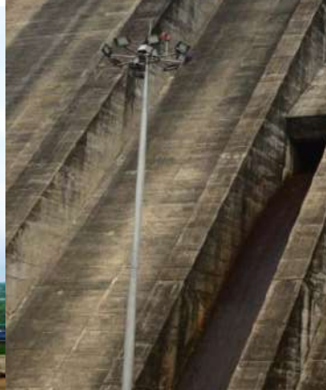
At Dam bottom near spillway bucket
