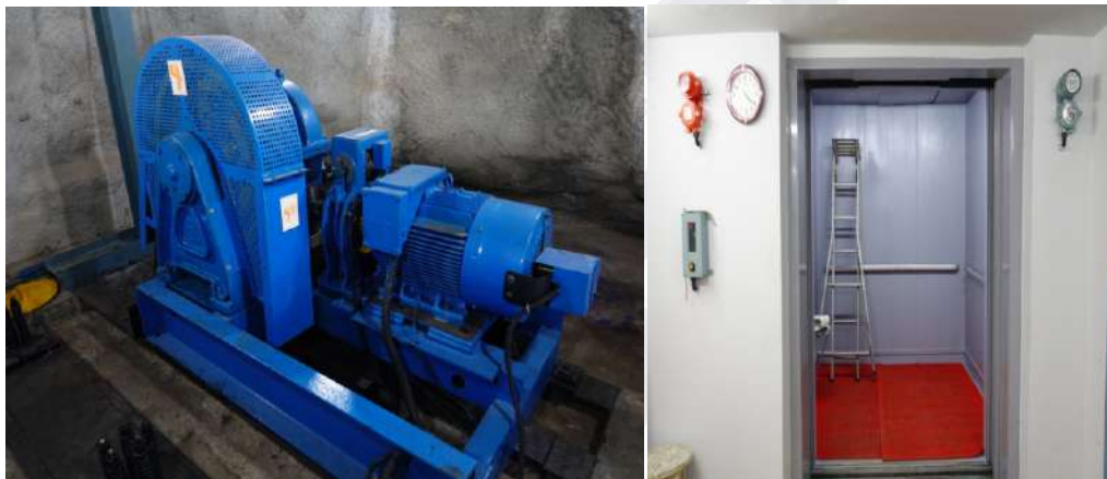
Modification to Elevator
