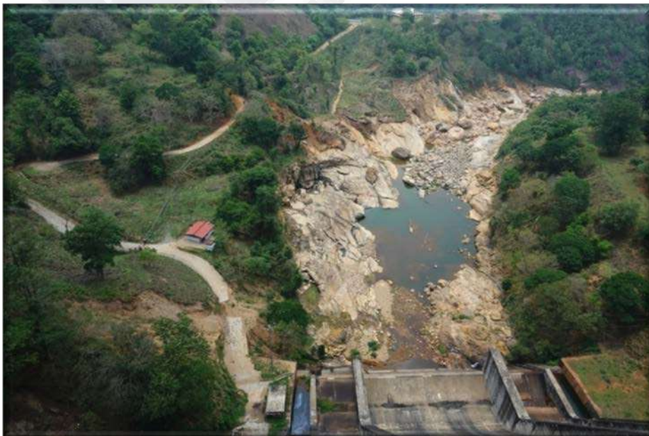
Fig 2.8 View of Spillway bucket from Hoist bridge
