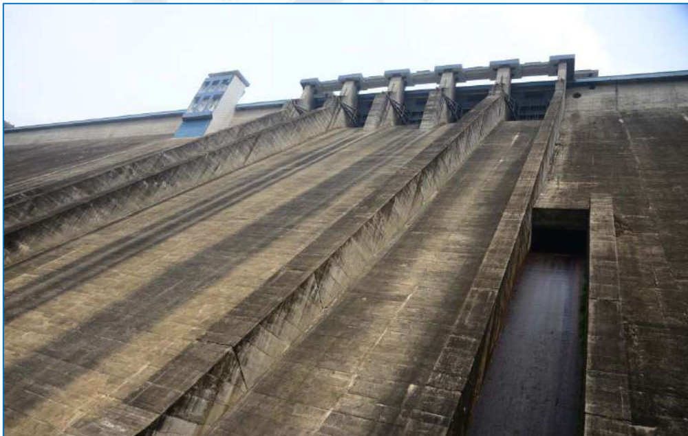
Fig 2.2a Downstream Elevation of Spillway
