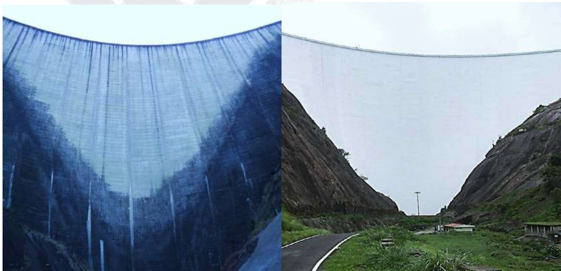
Painting the d/s face of Idukki dam
