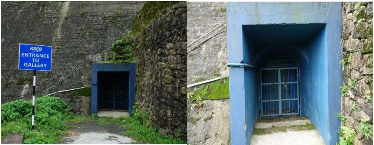
Entrance to Inspection Gallery
